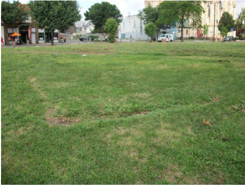
View of a former foundation wall located in the middle of the subject property.
