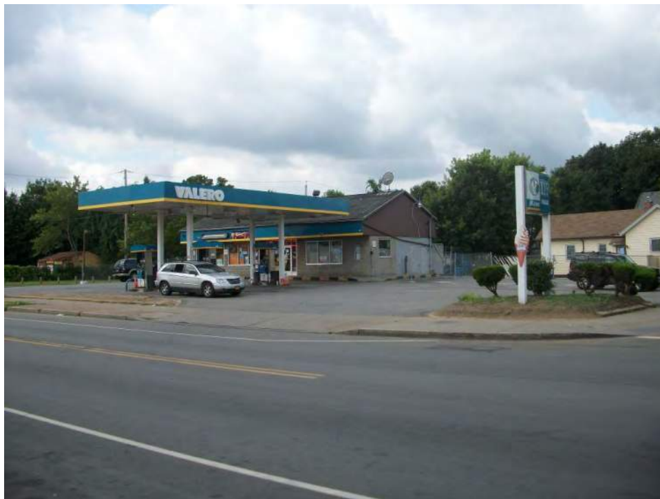
View of 799 North Clinton Avenue from the southwest corner of the subject property.
