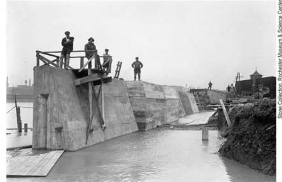
1917 H River retaining wall under construction near rail yard (RR roundhouse in background). Built for Barge Canal Terminal, dredging, and flooding control.
