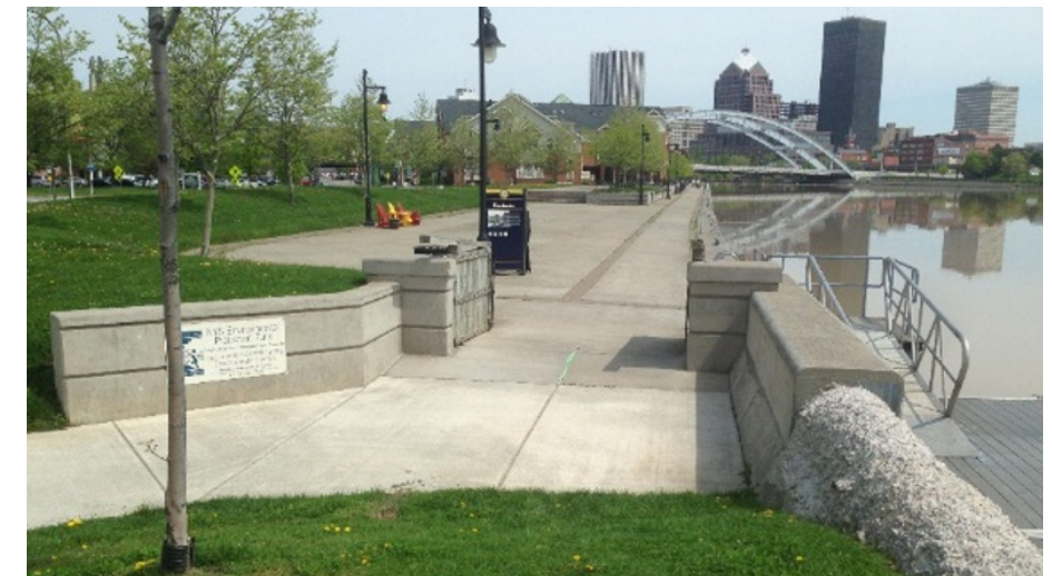
THE RIVERWAY TRAIL LOOKING NORTH TOWARDS CORN HILL LANDING, SHOWING EXISTING FLOOD GATES AND THE TRANSITION FROM OLD TO NEW SECTIONS OF THE RIVER WALL
