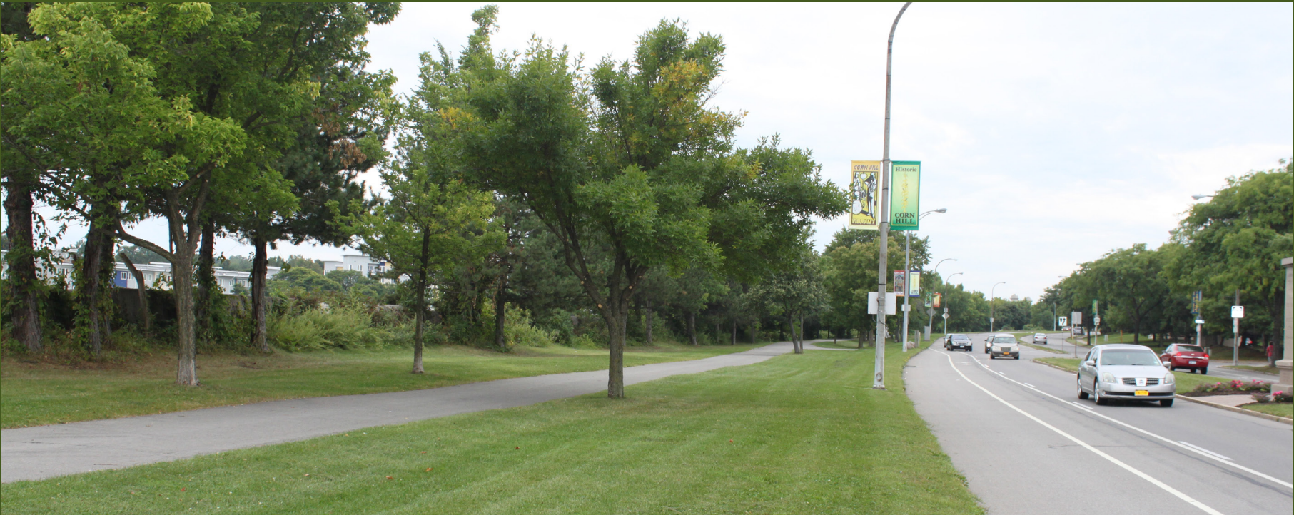
EXISTING VIEW LOOKING SOUTH TOWARDS FORD STREET
