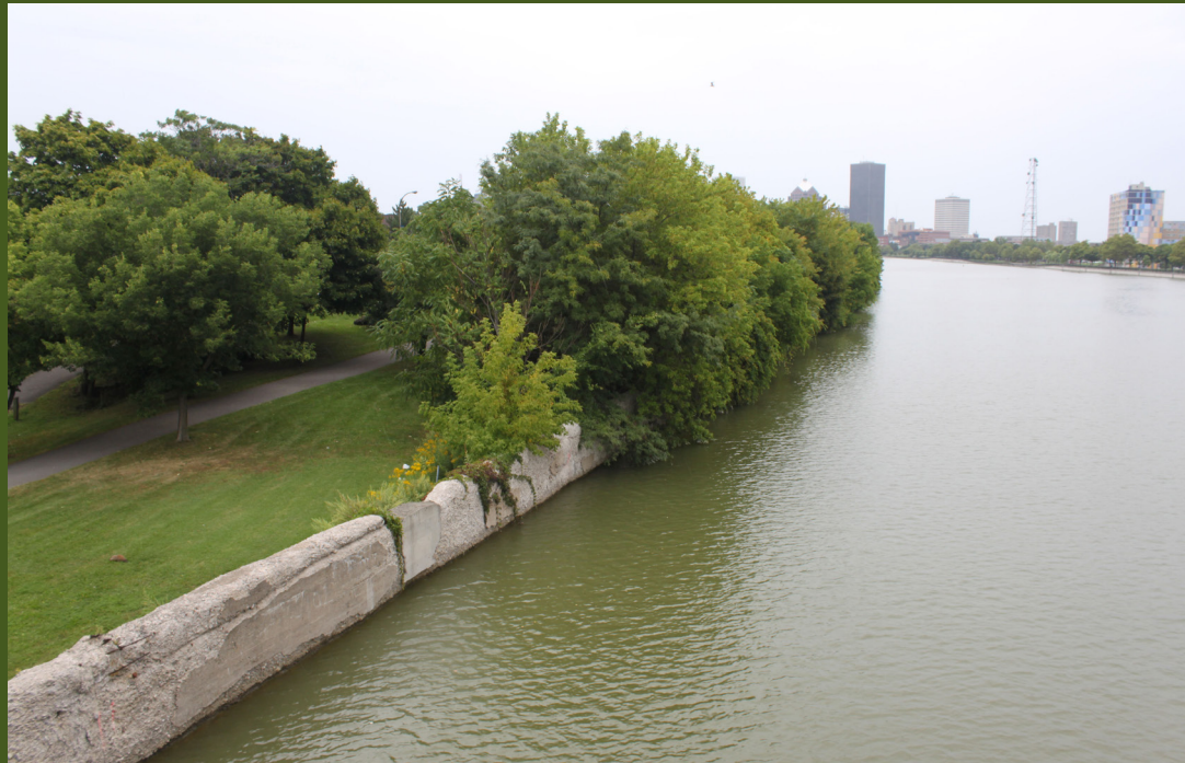
EXISTING VIEW LOOKING NORTH FROM FORD STREET BRIDGE
