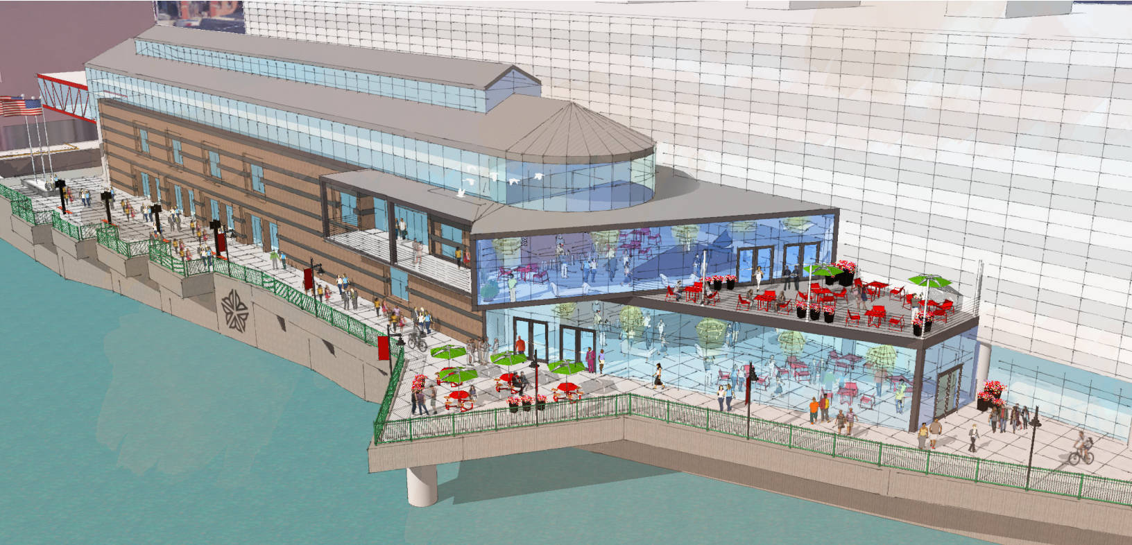
RIVERSIDE CONVENTION CENTER LOOKING NORTHEAST, SHOWING TERRACE IMPROVEMENTS AND PARTIAL EXPANSION
