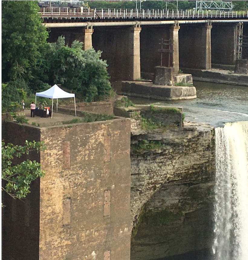
VIEW OF FORMER RG&E HYDROSTATION #4 | LOOKING SOUTH
