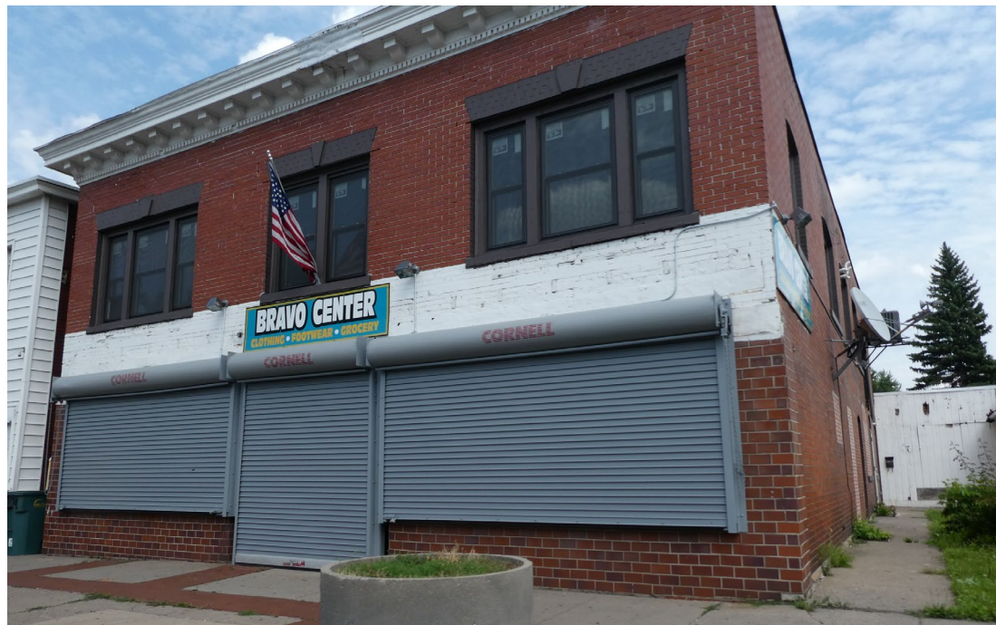
Perceptions concerning crime and safety are reinforced through elements of urban design such as rolling doors and bars on windows, and vacant, poorly maintained, or boarded-up properties.
