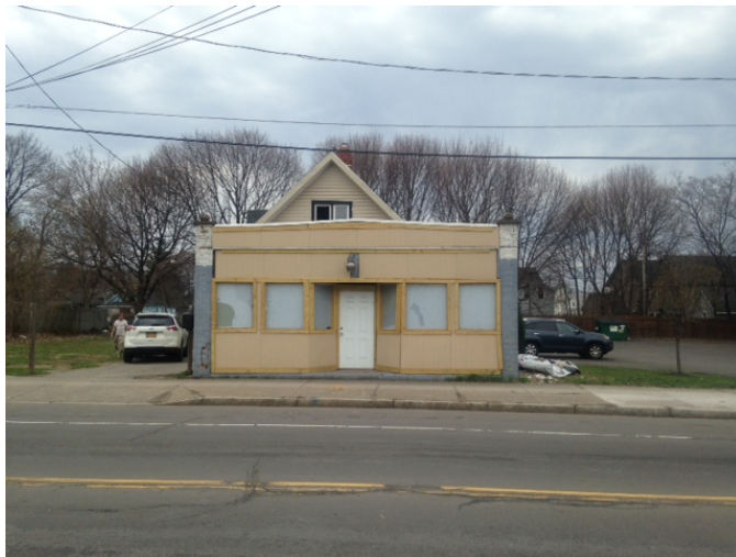
Building conditions vary considerably. Low demand for space and the large amount of vacant space work against the need for renovation and repair.
