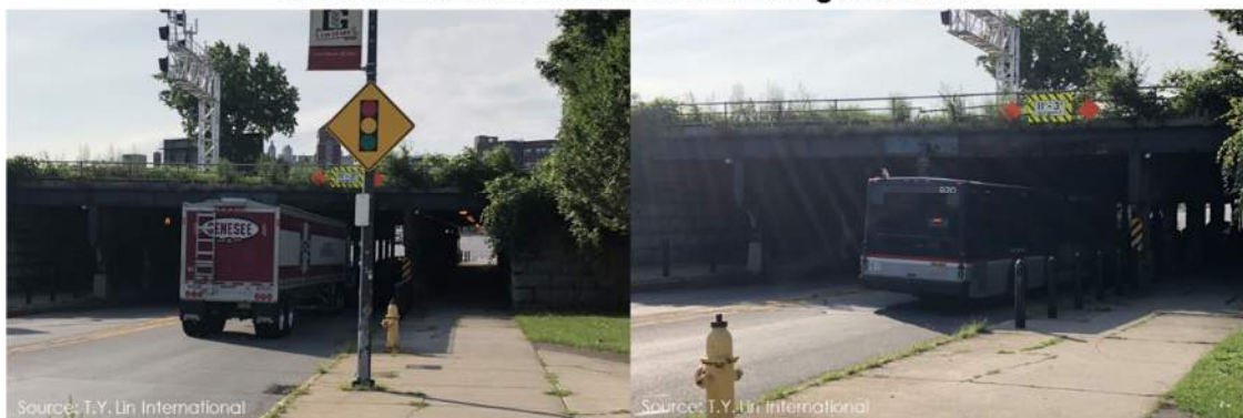
Figure 9. Low Bridge Clearance at St. Paul Street North of the Inner Loop in Rochester, New York
