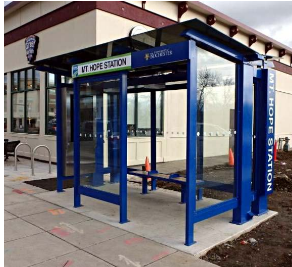
Figure 5 Shelter with Seating
