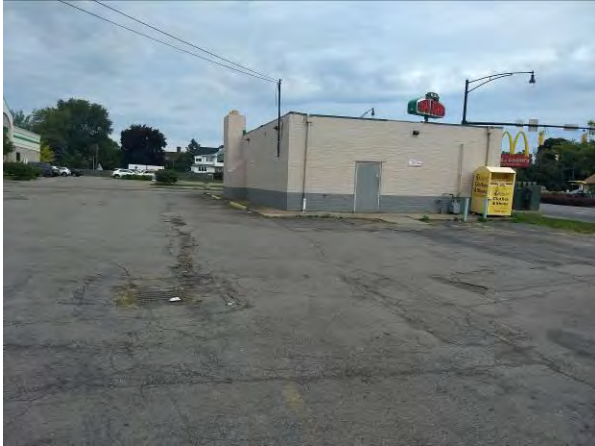
Photo No. 19 1667-1673 E. Main Street looking north to E. Main Street; former gasoline station.
