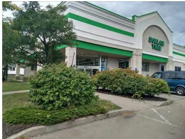
Photo No. 22 821 Culver Road.
