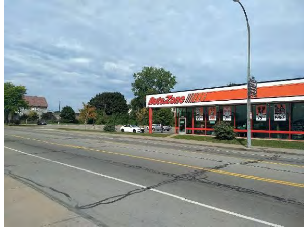
Photo No. 8 1154-1192 E. Main Street looking west.
