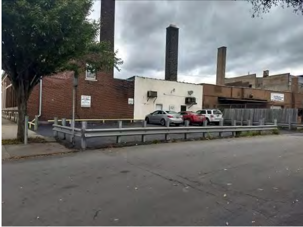
Photo No. 1 460-466 N. Goodman Street looking west; former gasoline station in parking lot area
