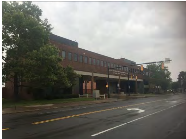
Photo No. 16 1372 E. Main Street looking northeast; NYSDEC PBS and spill facility
