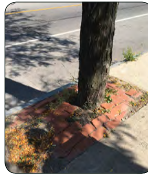
Special Condition Photo: Brick tree pit
