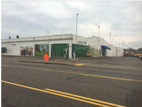
Photo No. 9 1185-1223 E. Main Street looking east/southeast.
