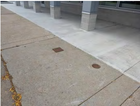
Photo No. 5 Monitoring well in sidewalk in front of 1124-1130 E. Main Street
