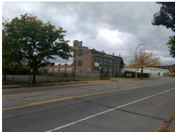
Photo No. 12 1233 and 1185-1223 E. Main Street looking west.
