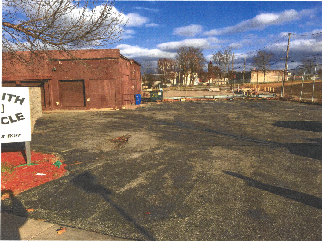
View of the assessed property (and a portion of the adjoining building to the north) looking east from York Street.
