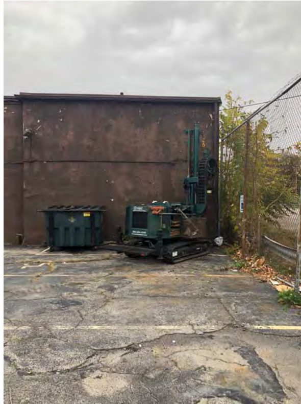
Track-Mounted Geoprobe direct-push drill-rig at test location TB/TMW-14-24 – looking north
