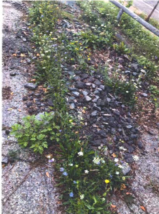
A mound of apparent asphalt along the south/central edge of the parking lot on the assessed property on 8/27/2018. (Note, this pile was removed prior to the 9/17/2018 site visit.)
