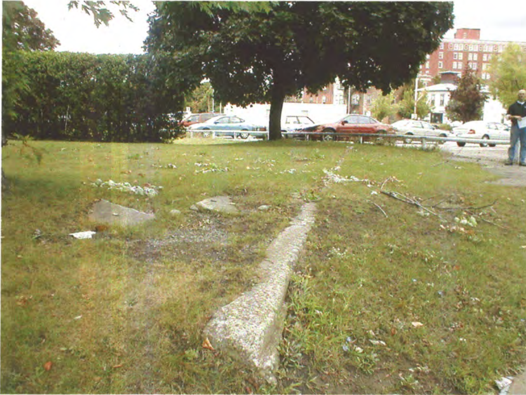
View of a visible concrete foundation on the southwest portion of the assessed property.
