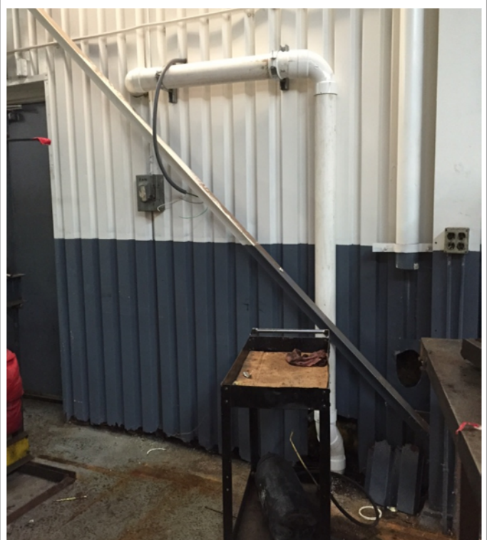
New interior vertical riser pipe (March 2017)
