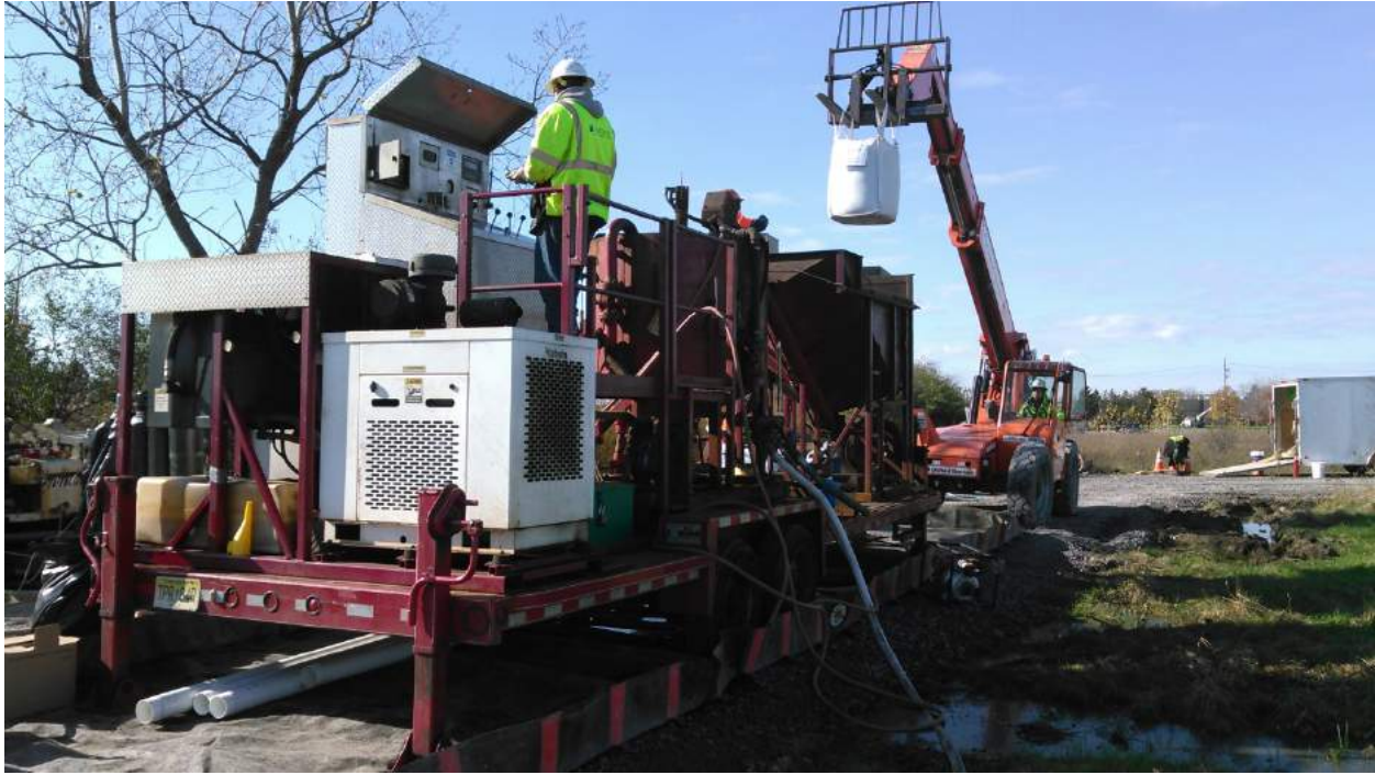
Loading Iron into Injection trailer
