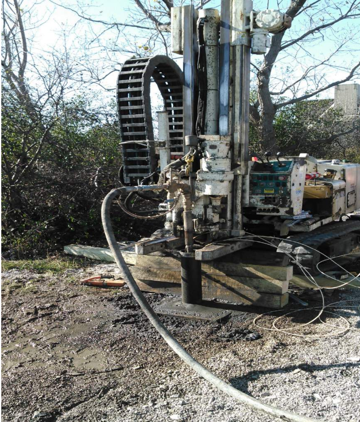
Injecting on Blast Frac Location
