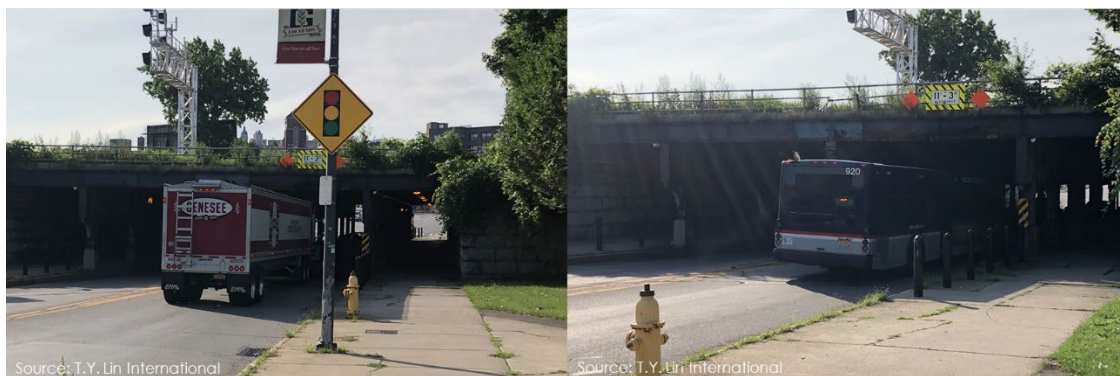
Figure 9 Low Bridge Clearance at St. Paul Street and the Inner Loop
