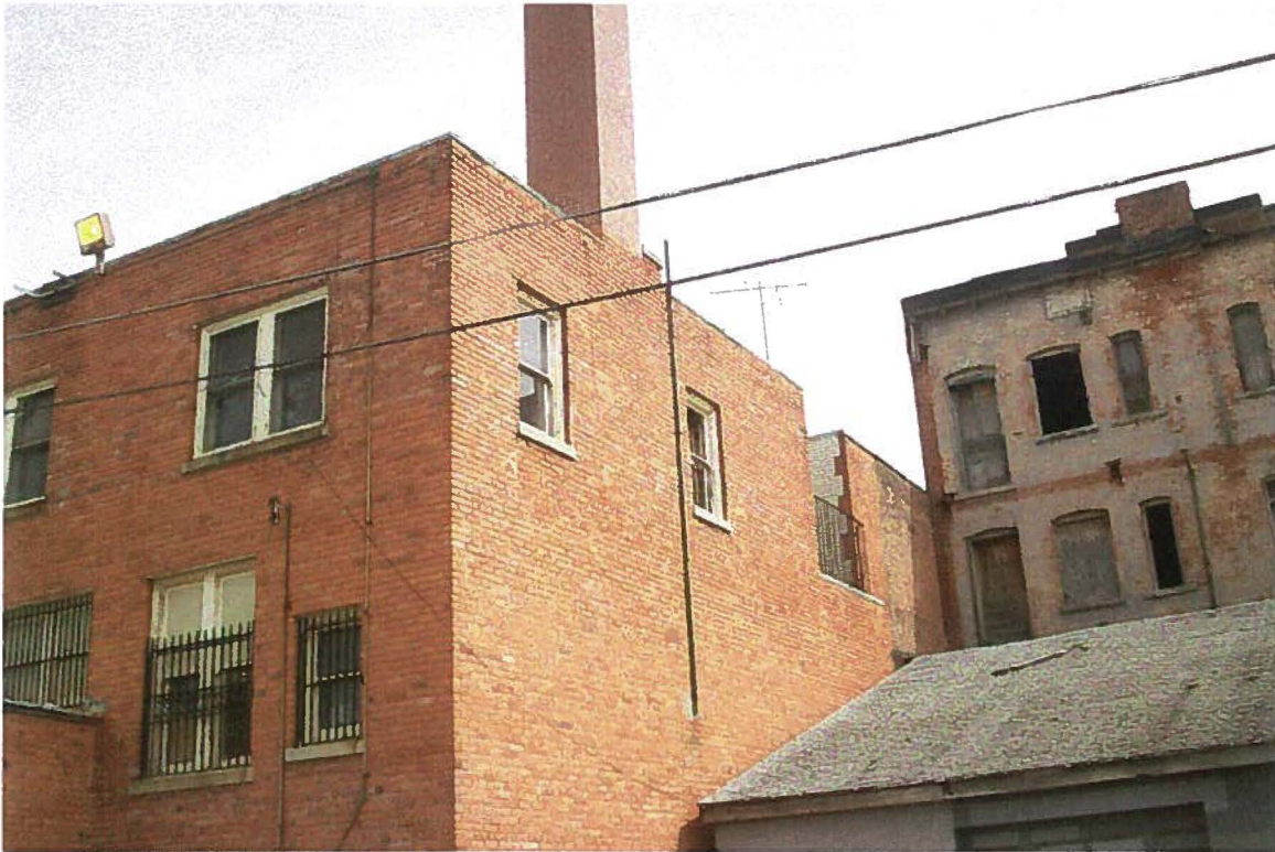
Property #74 (888-892 West Main Street) - View of vent pipe located on the west side of property.
