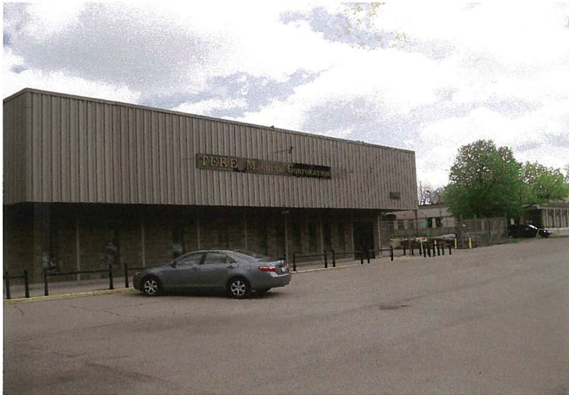
Property #21 (34-36 Colvin Street) - View of machine shop.
