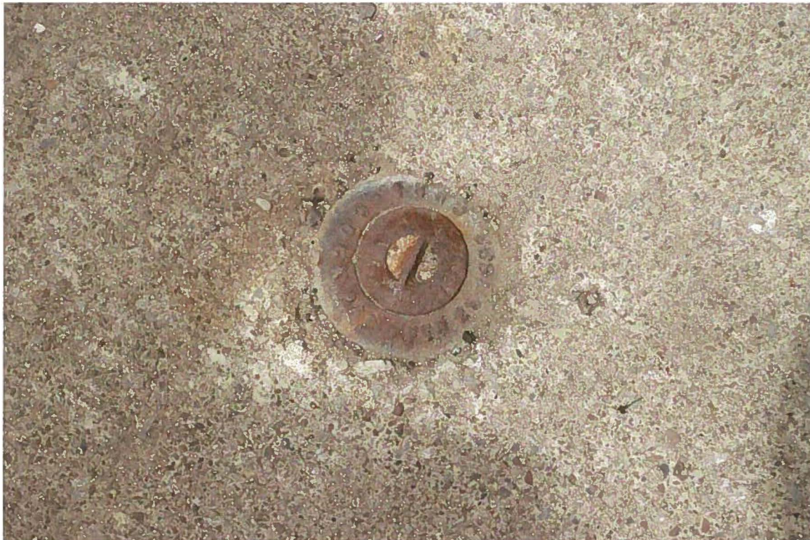
Property #2 (2 Algonquin Terrace) - View of potential fill port in sidewalk in front of property.
