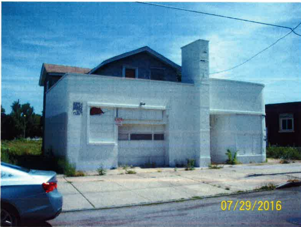
View of the adjoining property to the north (50 York Street) looking east.
