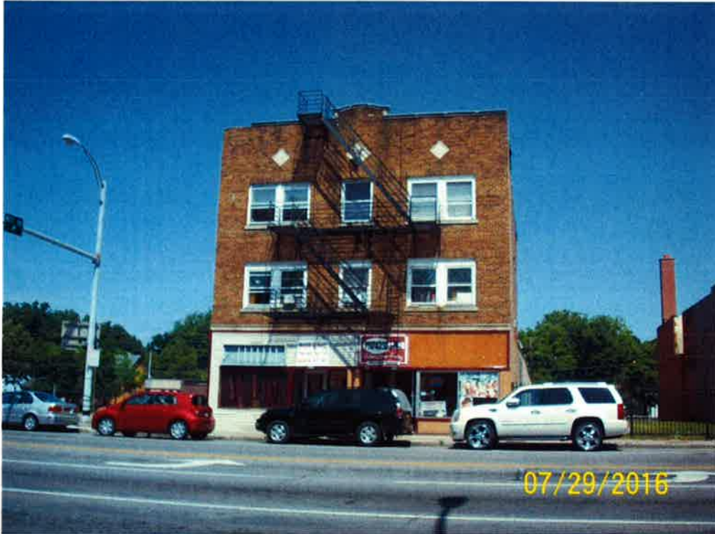
View of the assessed building looking north from the south side of W. Main Street.
