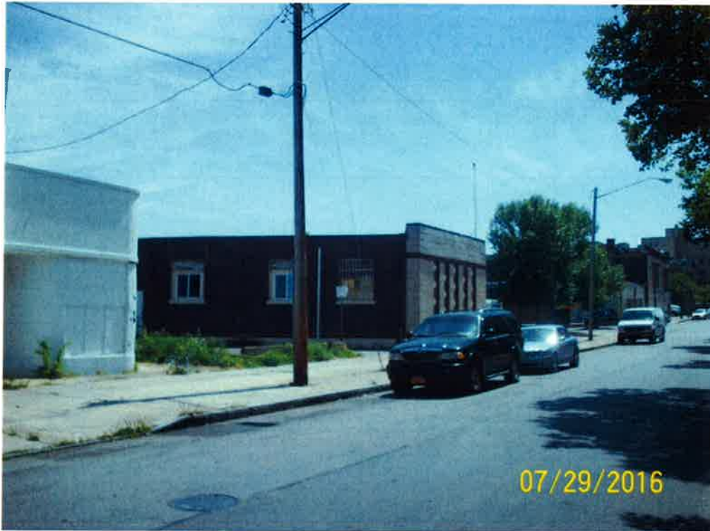
View of the adjoining property to the east (32 York Street) looking south/southeast.
