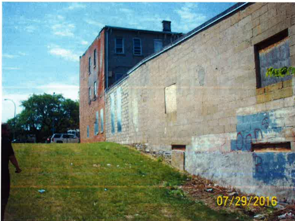
View of the eastern exterior of the assessed building looking south.
