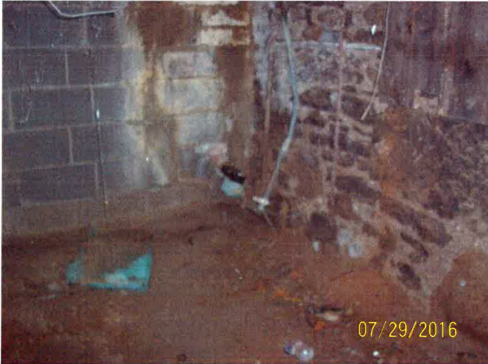
View of the interior basement walls on the northern portion of the assessed building.
