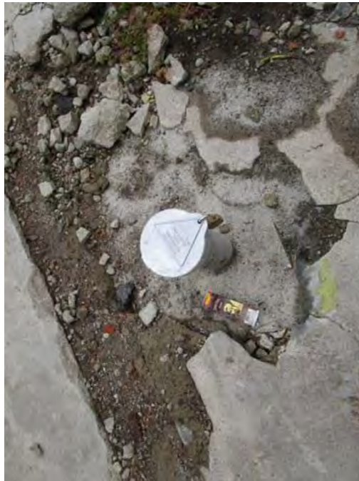
Typical monitoring well on former off-site drycleaning site
