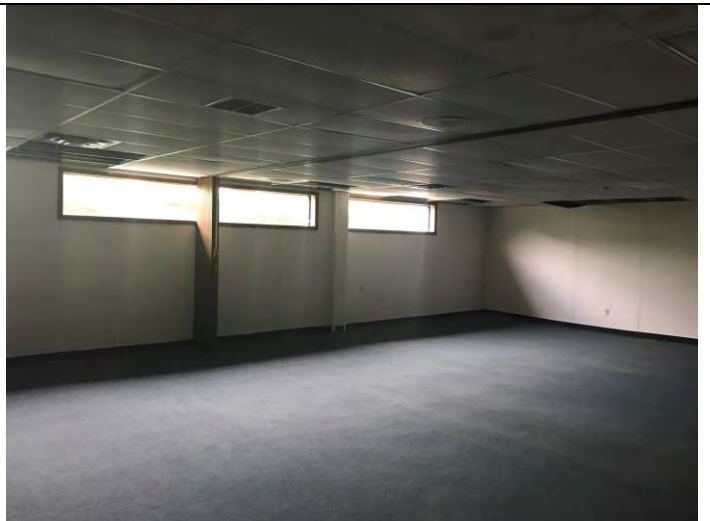
Typical view of the interior of Section 9
