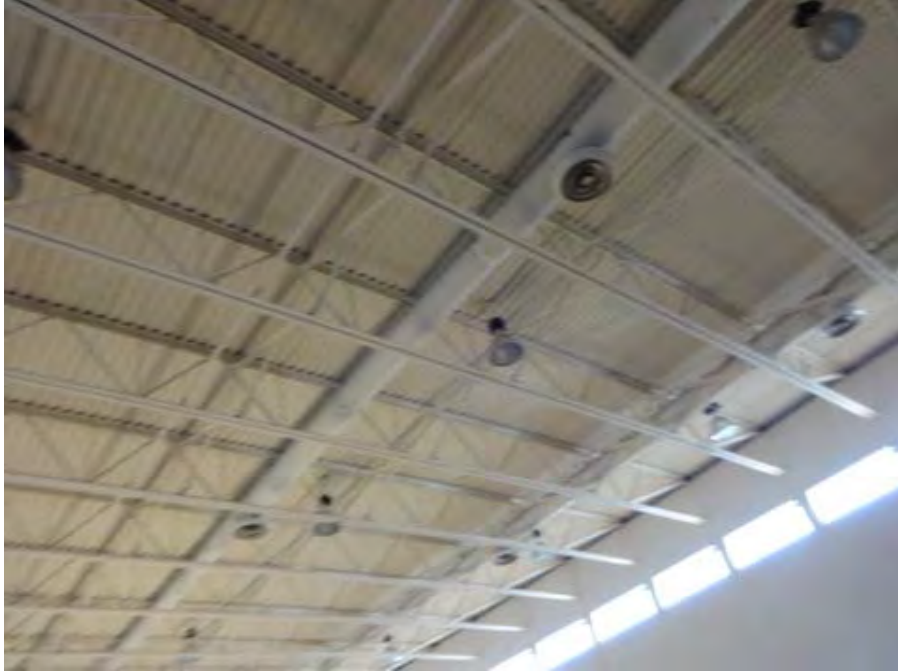
Steel framing and roof decking in basketball court
