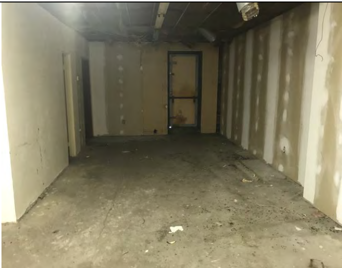
Typical view of the second floor interior of Section 6- Garage
