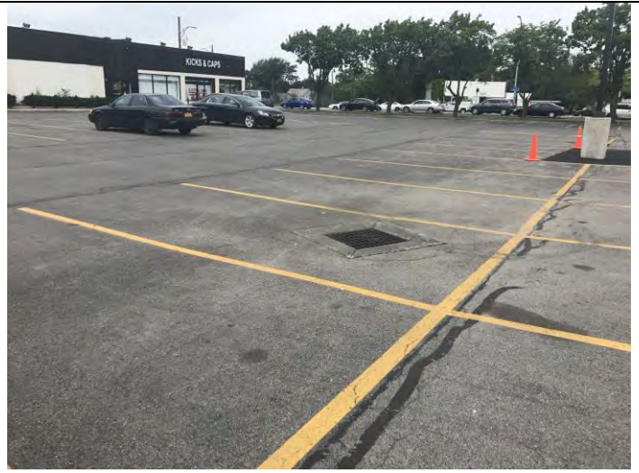
Representative storm drain located on the eastern portion of the Site
