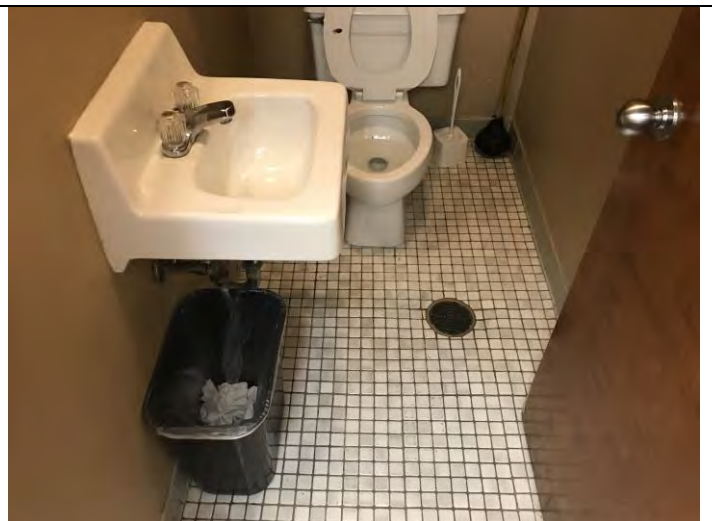
Representative restroom and associated floor drain in Section 4
