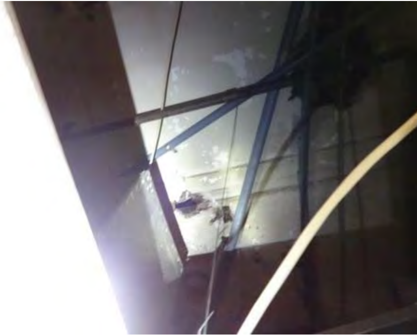
Steel framing and roof decking
