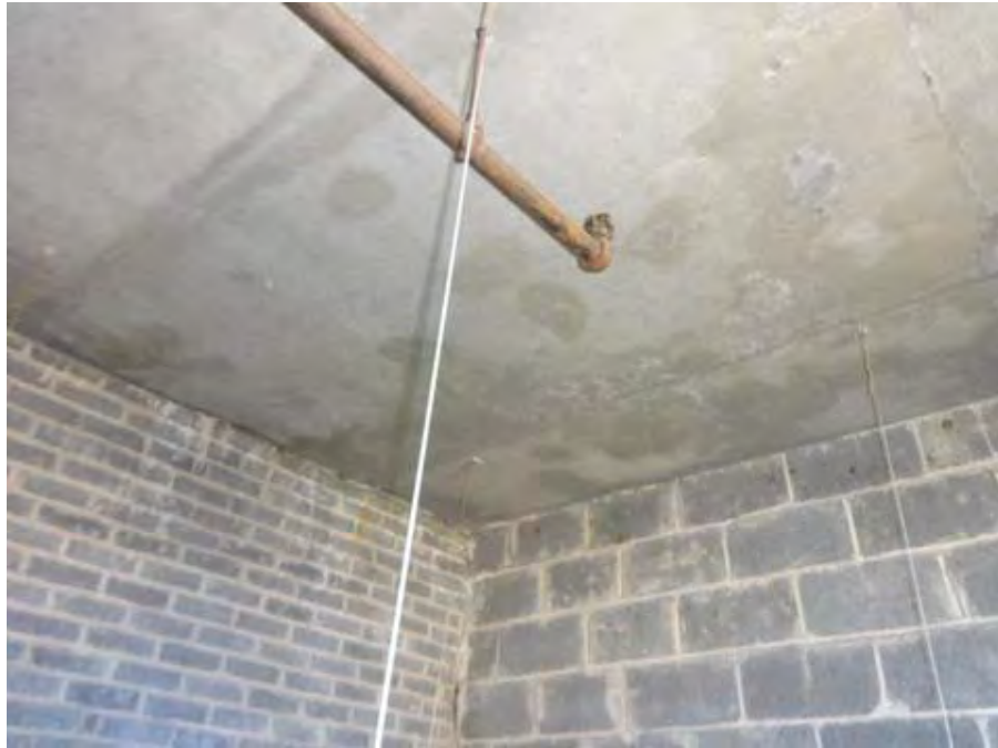
CMU wall and roof decking
