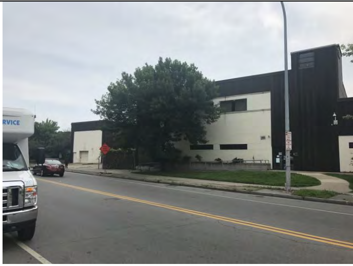
Typical view of the western exterior of the Site Building
