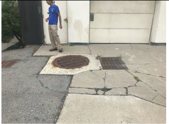
Typical view of the western exterior of the Site Building (Section 6)
