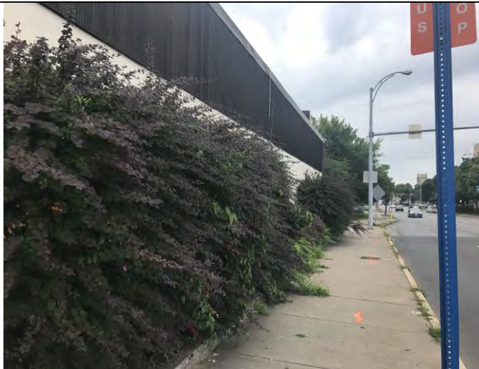
Typical view of the western exterior of the Site Building
