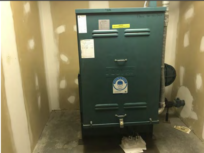
Typical view of the elevator components in the elevator room on the first floor of Section 7
