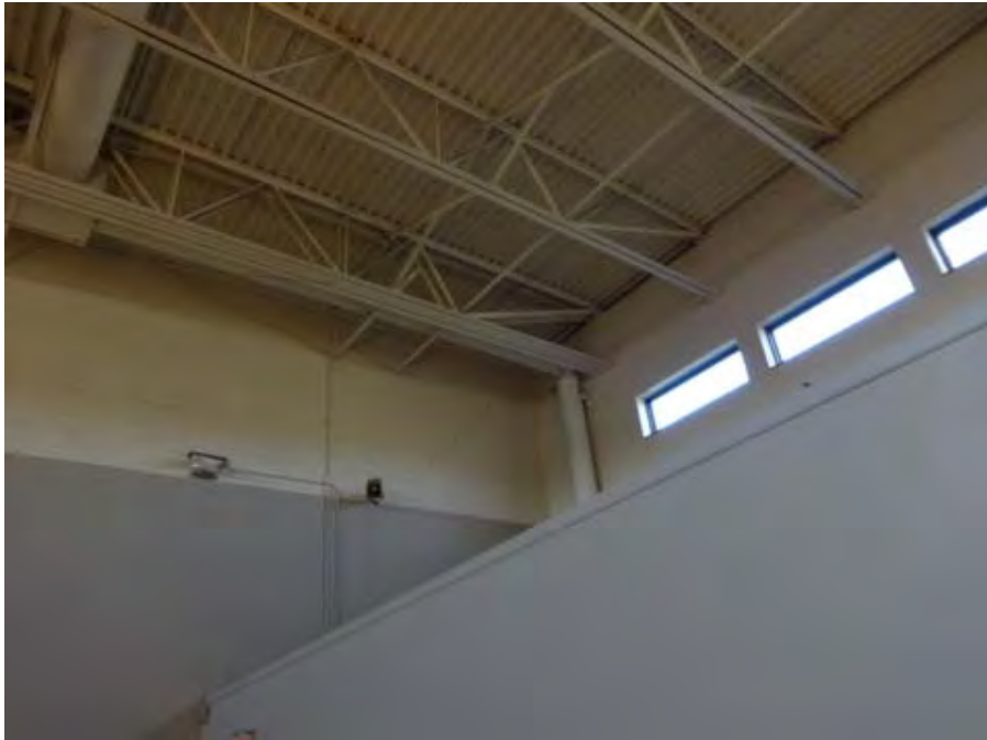
CMU wall, steel framing and roof decking in basketball court
