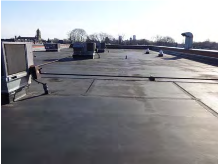
Typical roof surface
