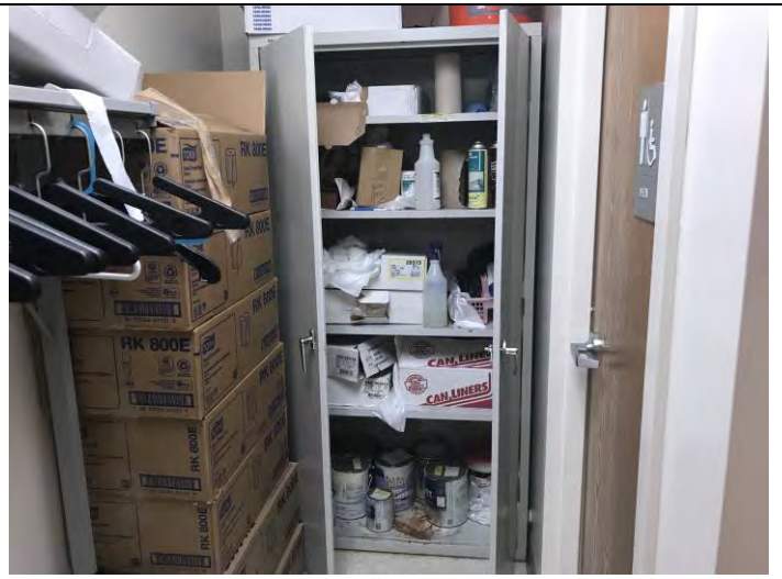
Typical view of a storage closet containing paint located on the second floor of Section 7
