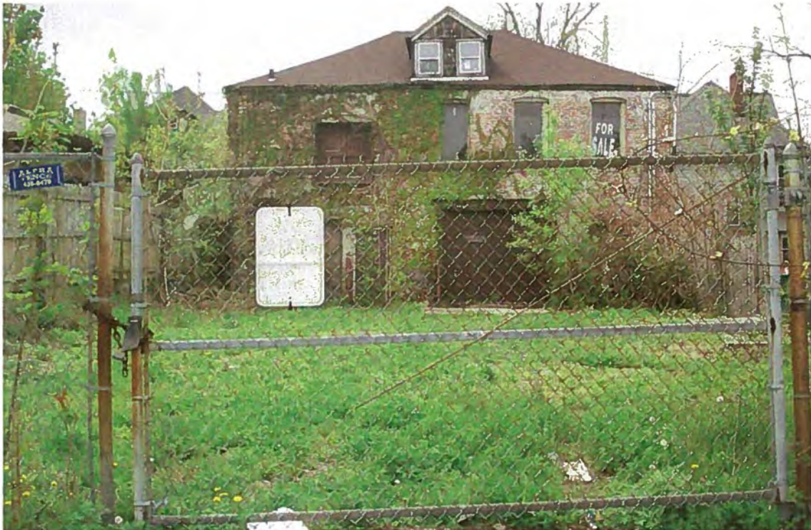
Property #87 (21-23 York Street) - View of former automobile repair facility, looking west.
