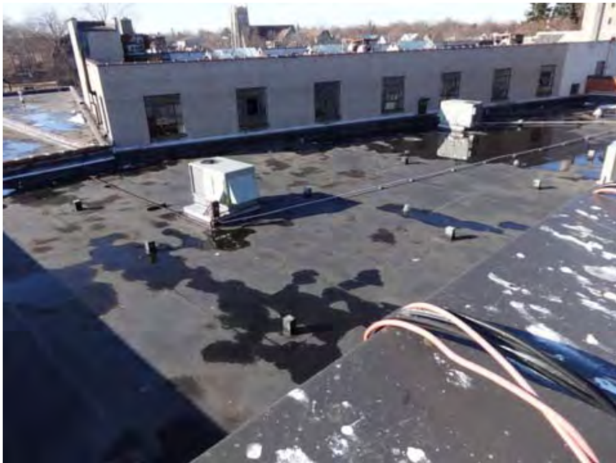
Various building roofs
