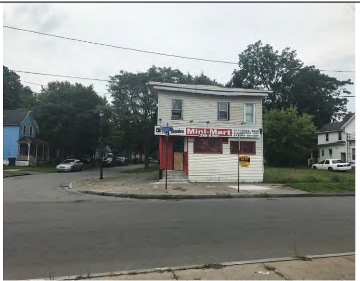
Typical view of a southern adjacent property
