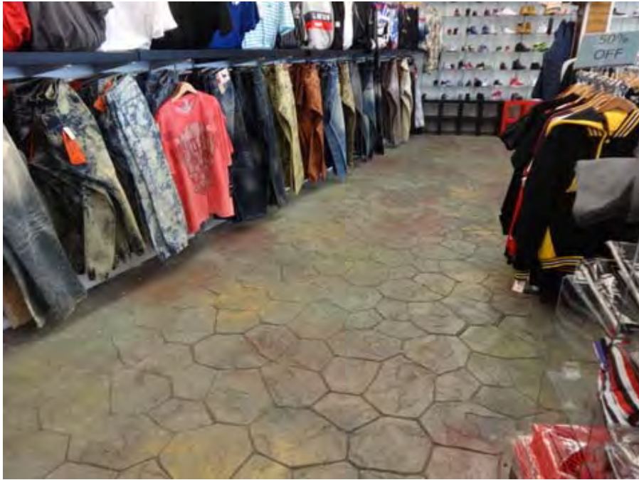
Typical occupied tenant space
