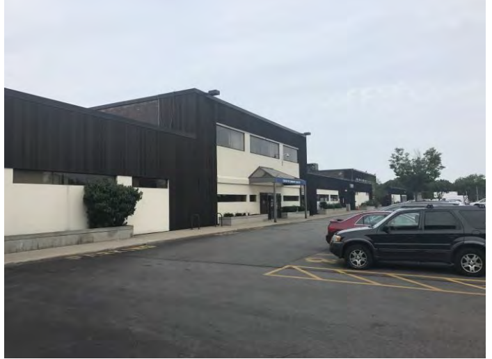
Typical view of the eastern exterior of the Site Building (Sections 5, 7 and 8)
