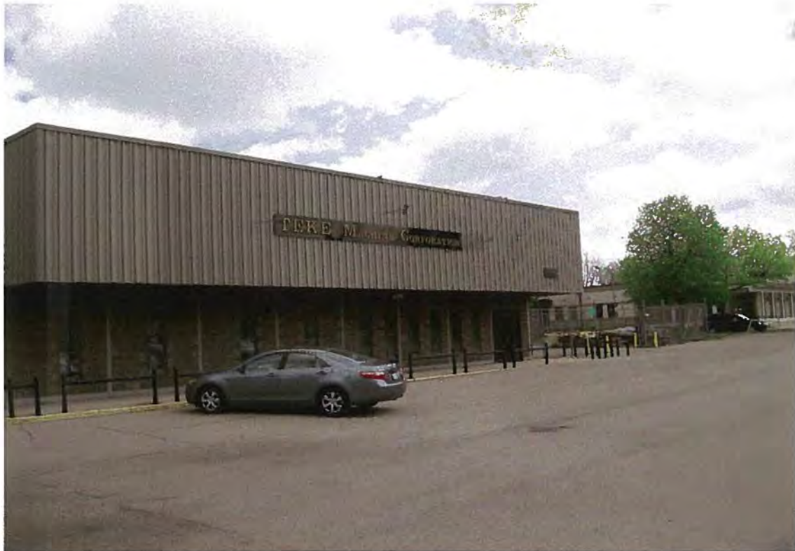
Property #21 (34-36 Colvin Street) - View of machine shop.
