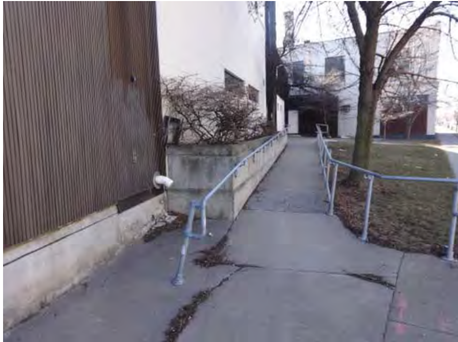
ADA ramp and metal railing
