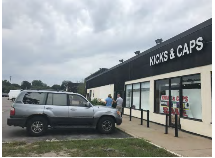
Typical view of the eastern exterior of the Site Building (Sections 1 and 2)
