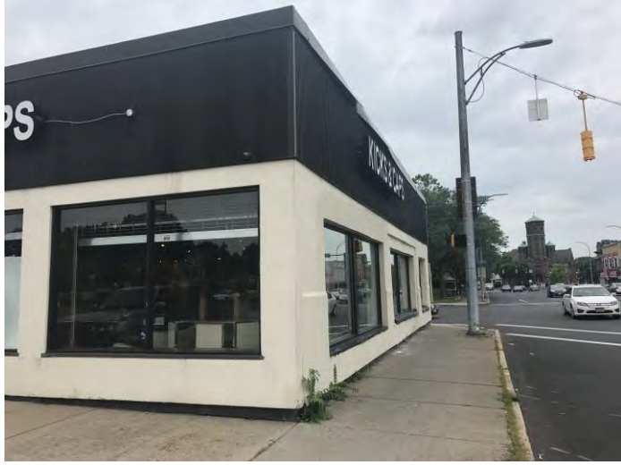
Typical view of the northern exterior of the Site Building
