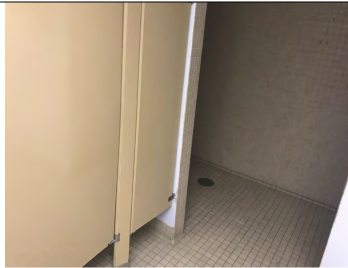
Representative restroom and associated floor drain in Section 3
