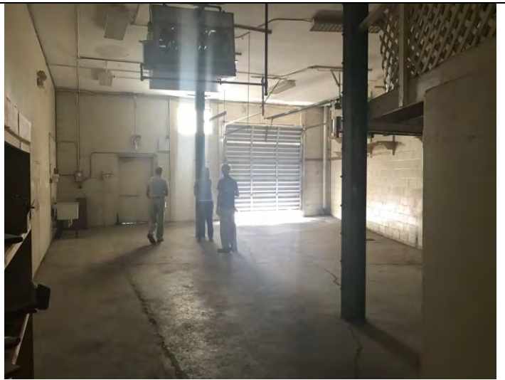
Loading dock area in Section 8
