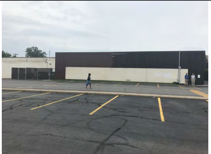
Typical view of the eastern exterior of the Site Building (Section 9)
