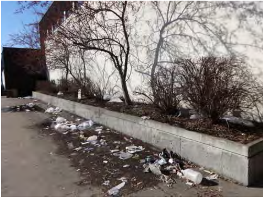
Landscaping and retaining walls
