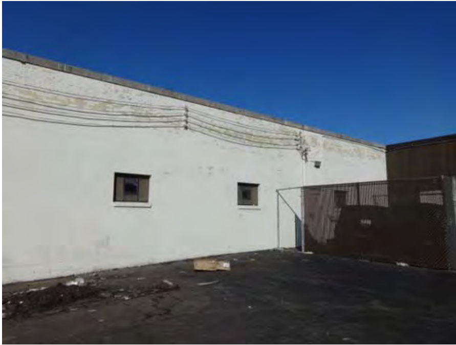
Typical facade on rear building elevation
