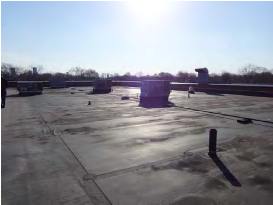
Typical roof surface
