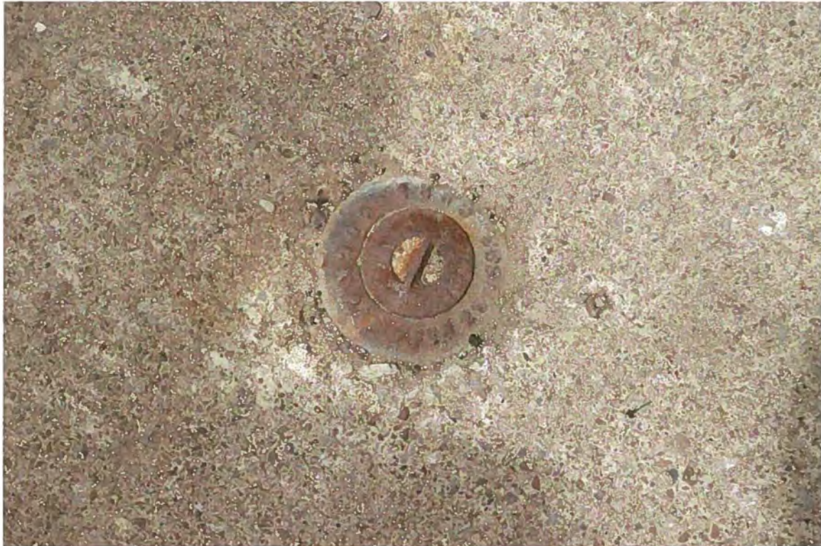
Property #2 (2 Algonquin Terrace) - View of potential fill port in sidewalk in front of property.
