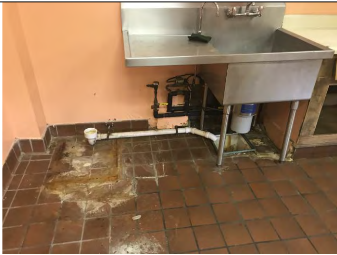
Representative floor drain in the kitchen in Section 9
