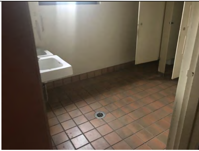
Representative restroom and associated floor drain in Section 9
