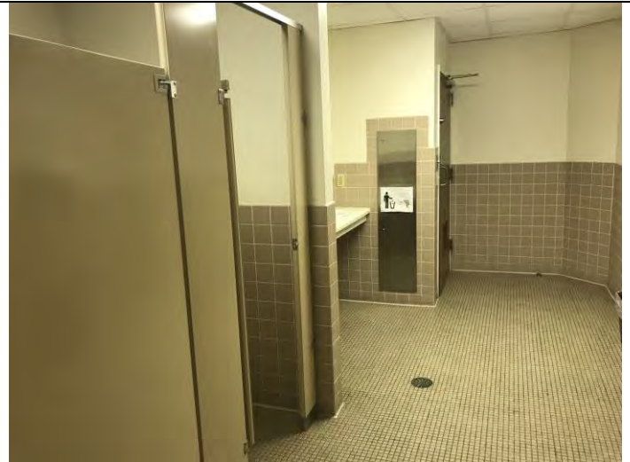
Representative restroom and associated floor drain located on the first floor of Section 7
