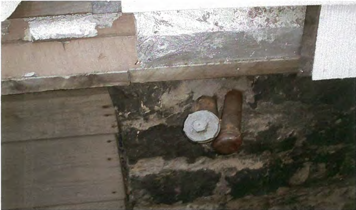
Property #58 (4 Kensington Street) - View of vent and fill pipes associated with apparent residential heating oil tank.
