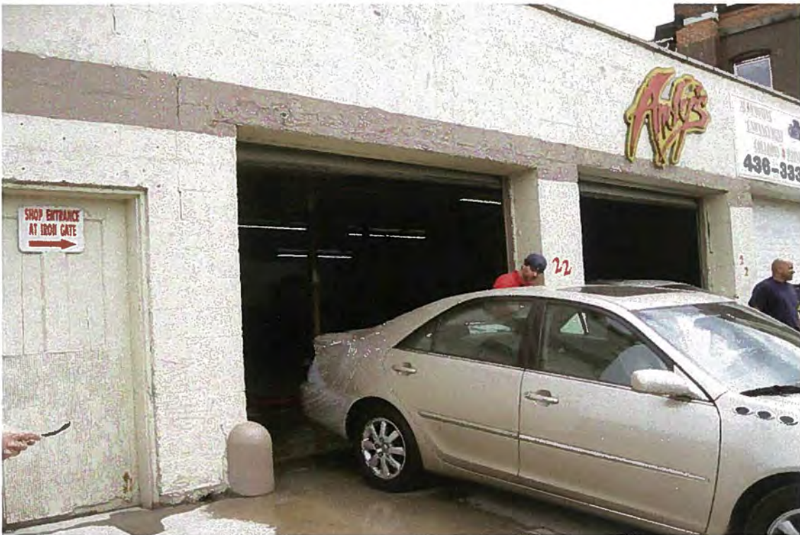
Property #82 (932-938 West Main Street) - View of automobile repair shop.
