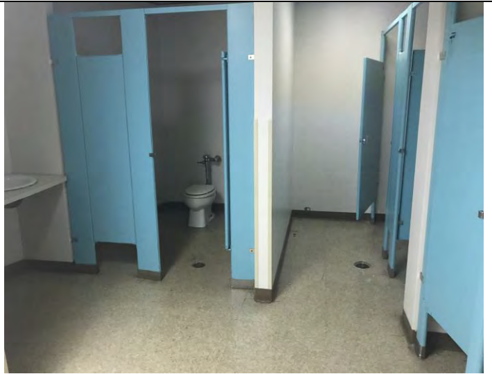
Representative restroom and associated floor drain in Section 8
