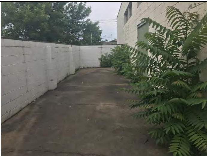
Typical view of the southern exterior of the Site Building
