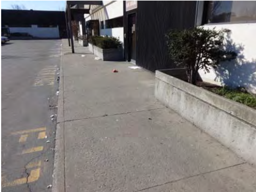
Typical flatwork and retaining walls
