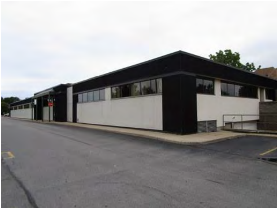
Adjacent property to the East
