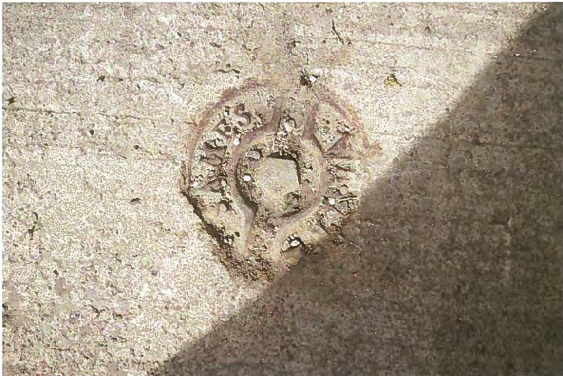
Property #71 (239 Silver Street) - View of potential fill port in sidewalk surface in front of property.
