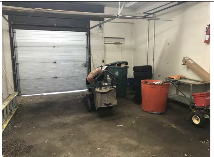
Typical view of the first floor interior of Section 6- Garage
