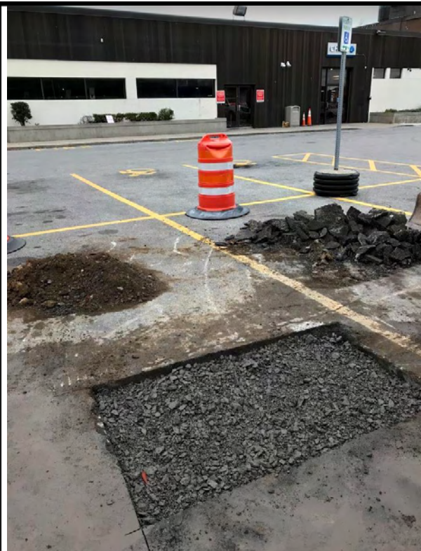
TP-04 post excavation. Filled with crushed stone to prepare for repaving.
