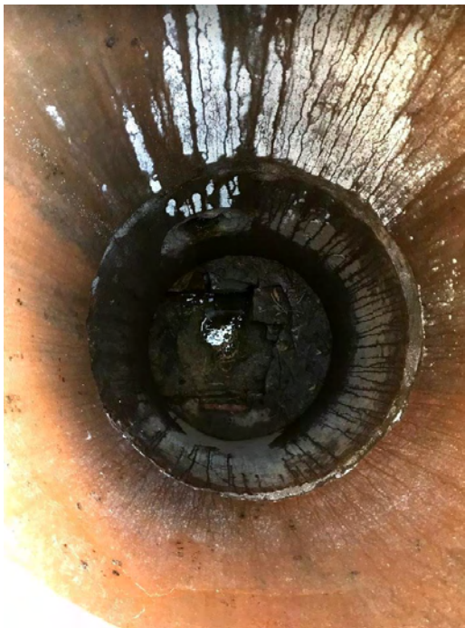
Catch basin in bedrock in northwest corner of the Site.
