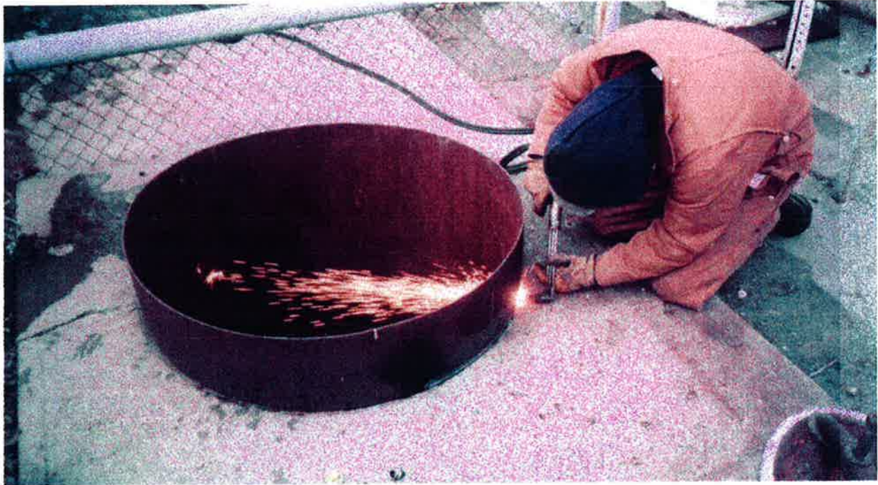
Methanol UST manway riser being removed (pressure cover at bottom right)
