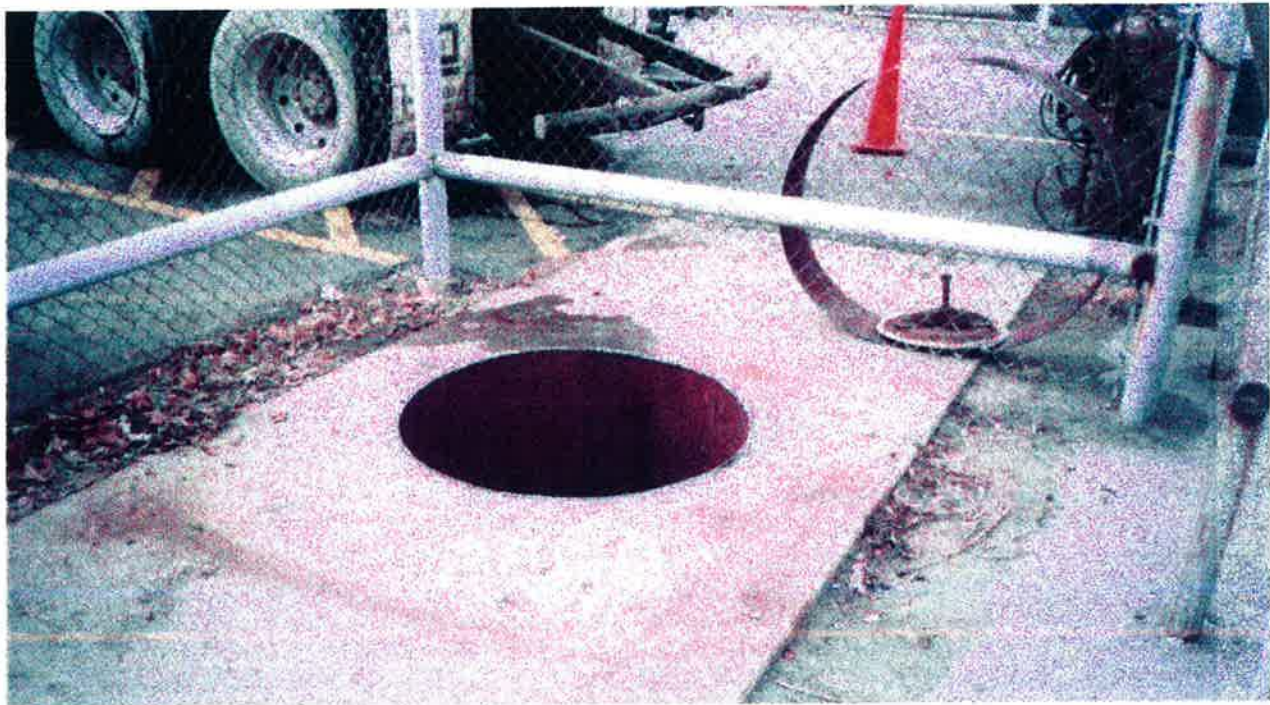
Manway riser removed (upper right) prior to filling UST
