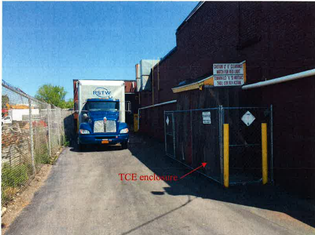
View of the western exterior portion of the assessed property, looking north. Note the enclosure for TCE tanks.
