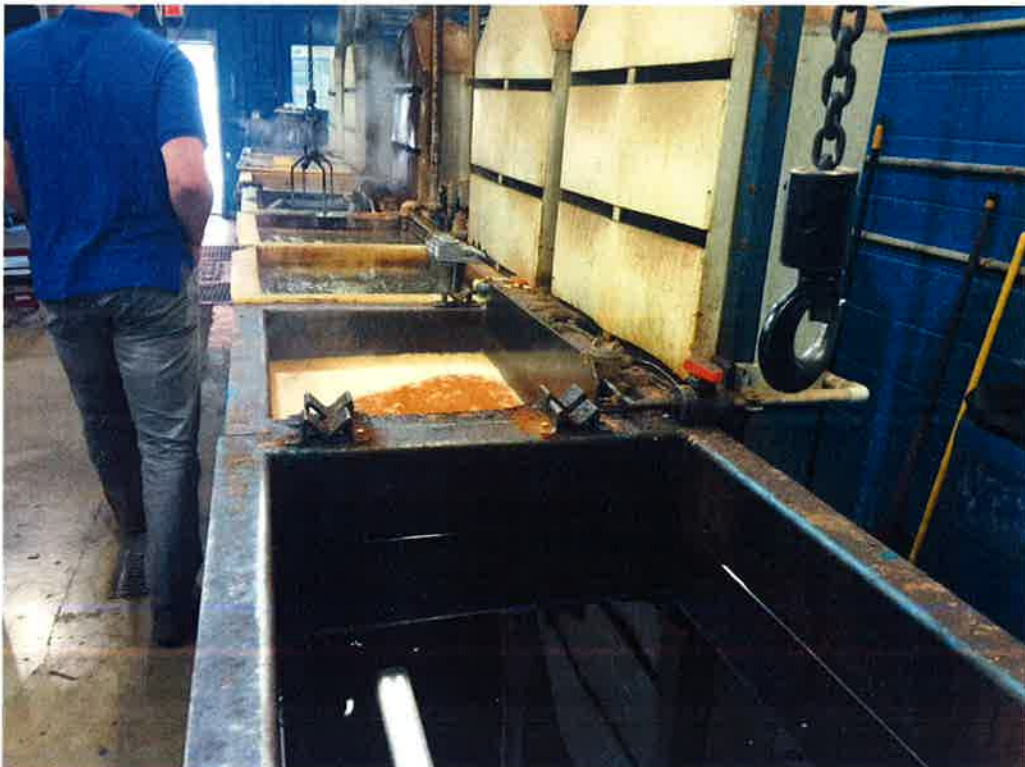
View of the black oxide line (i.e., on the northeast interior portion of the assessed building).
