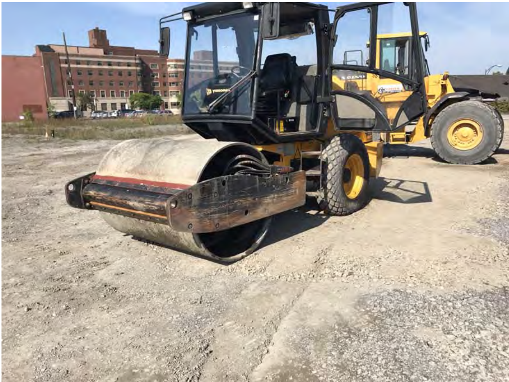
Decontaminated vibratory roller and loader – looking northwest (9-25-2019)
