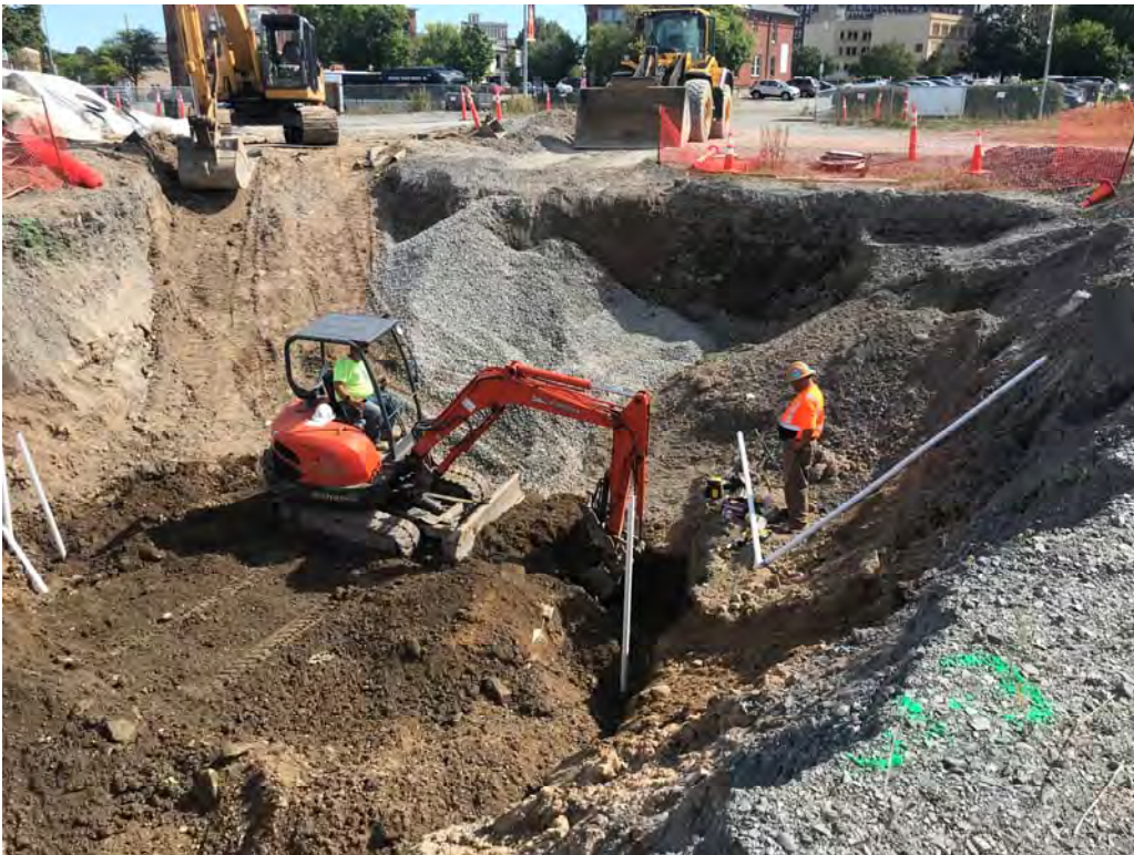
Installing ISCO piping in trench within partial backfill – looking southeast (9-18-2019)
