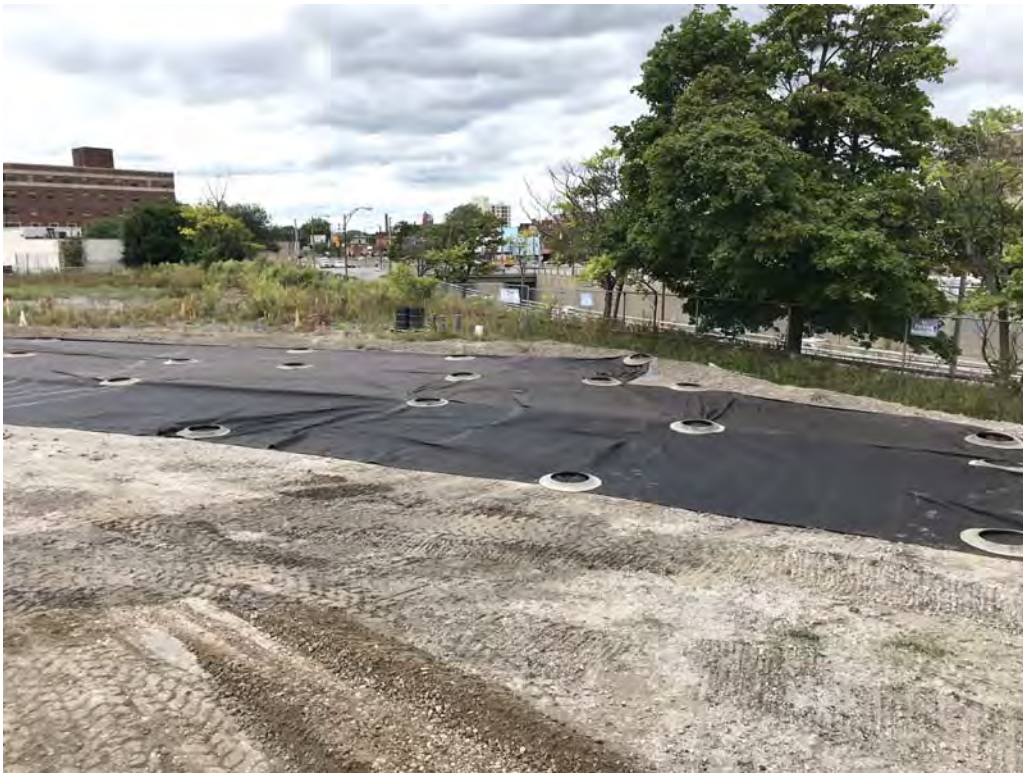
Construction of soil staging area – looking west (9-4-2019)
