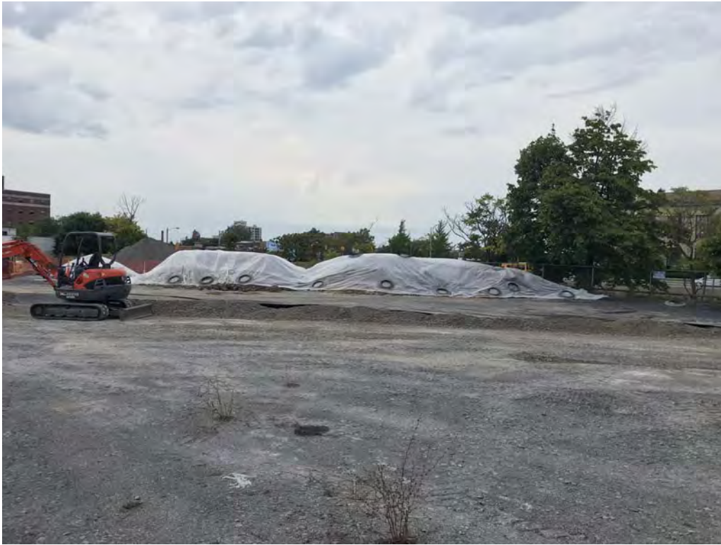
Staged re-useable soil covered with plastic sheeting – looking northwest (9-10-2019)
