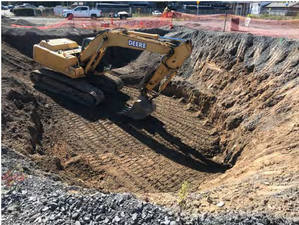
Backfilling excavation using re-usable Site soil – looking south (9-17-2019)
