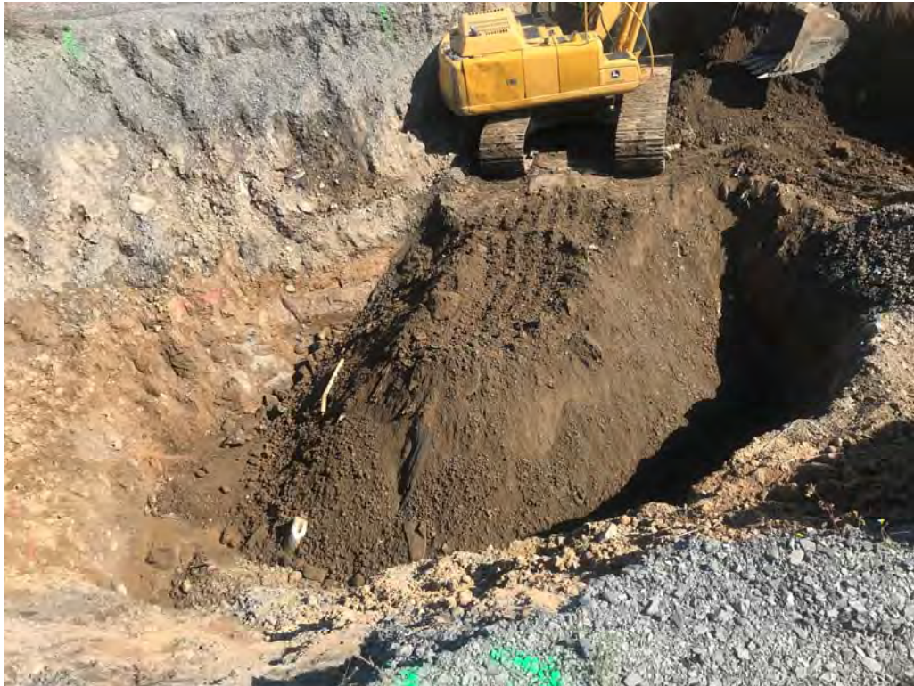
Backfilling excavation using re-usable Site soil – looking southeast (9-16-2019)
