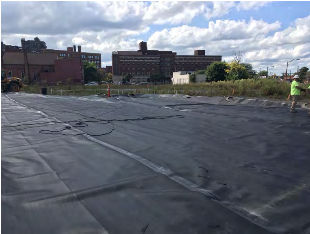
Plastic welding sheet of soil staging area liner – looking west (9-5-2019)
