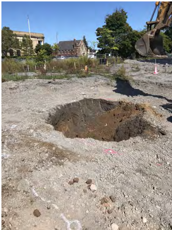
Excavating re-usable soil – looking northeast (9-9-2019)
