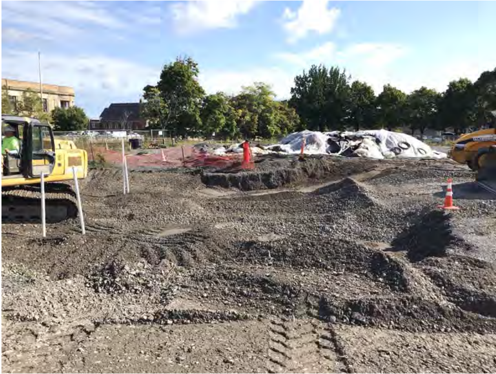
Backfilling with existing staged crusher run #2 cover system material – looking east (9-24-2019)
