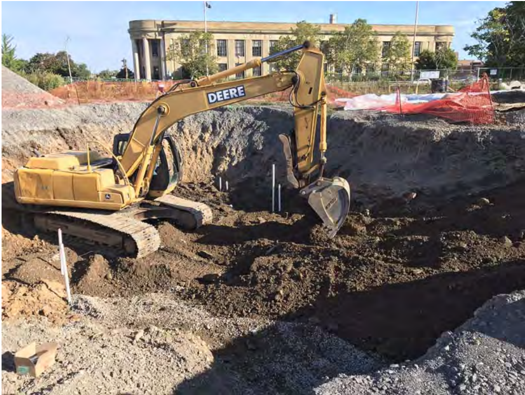
Resuming backfill of excavation with re-usable Site soil – looking northeast (9-19-2019)
