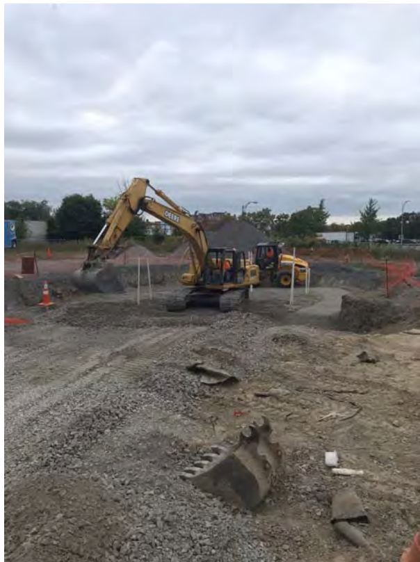
Backfilling with imported crusher run #2 – looking northwest (9-23-2019)
