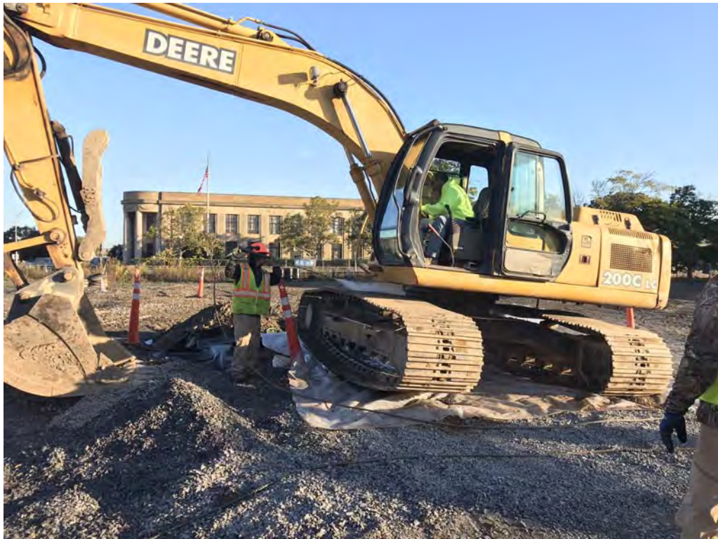
Decontaminating excavator tracks – looking north (10-11-2019)
