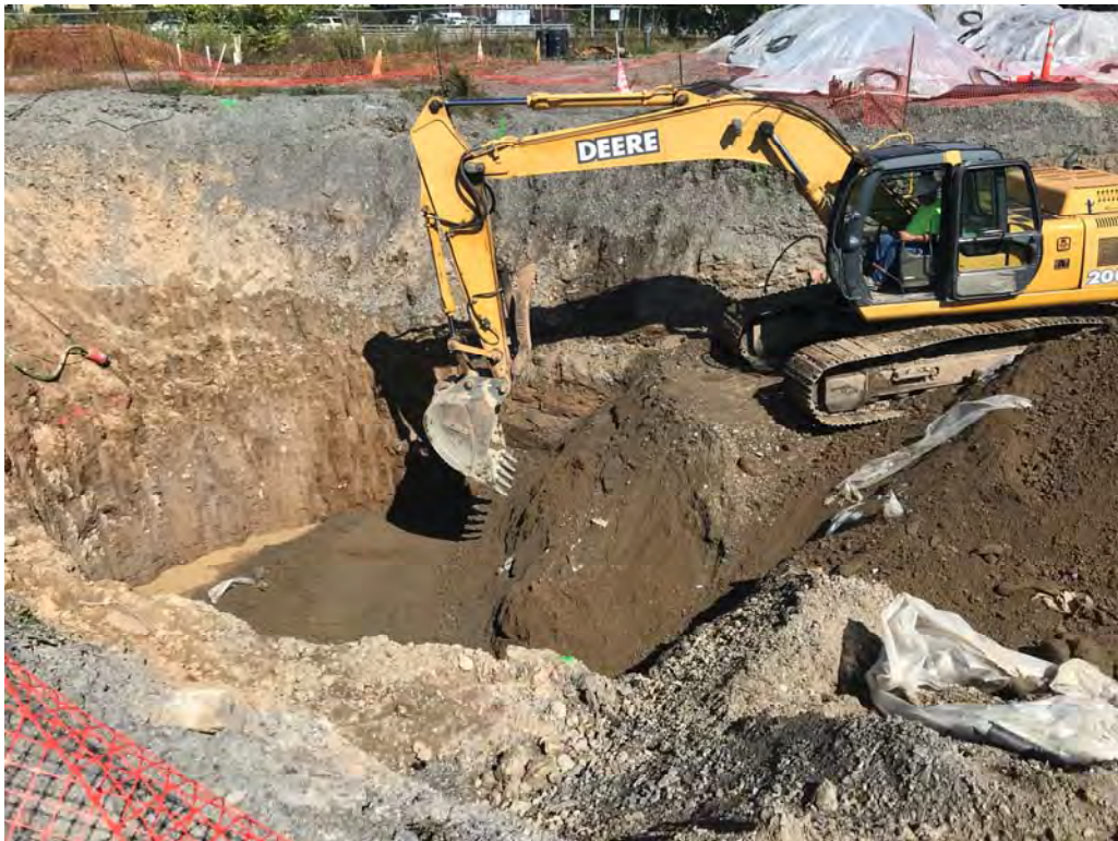
Backfilling excavation using re-usable Site soil – looking northeast (9-16-2019)
