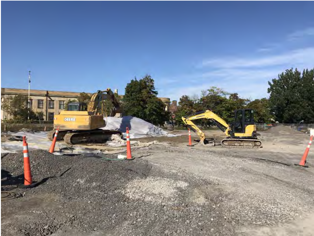
Cover remaining contaminated soil pile at end of day – looking northeast (10-9-2019)
