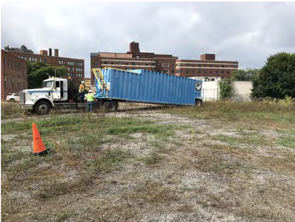
Delivery of frac tank for excavation dewatering – looking northwest (9-11-2019)
