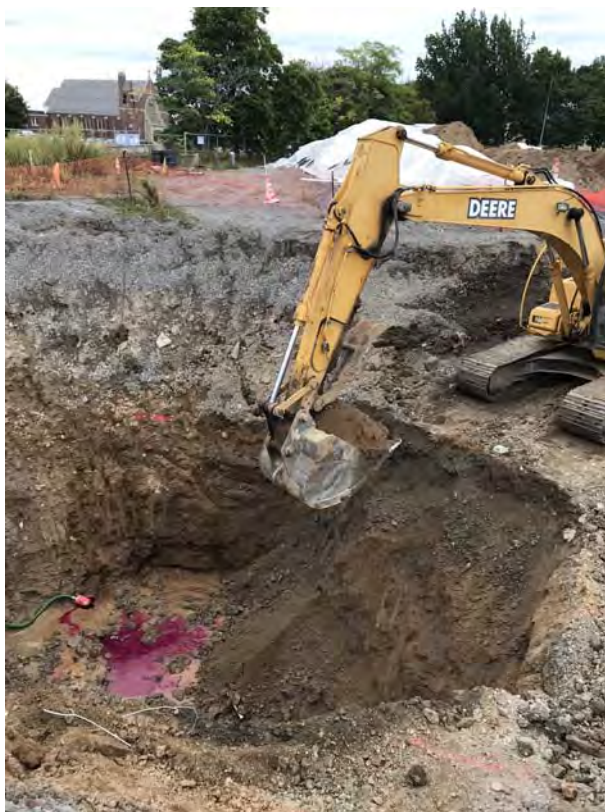
Contaminated soil removal with concurrent excavation dewatering – looking east (9-13-2019)
