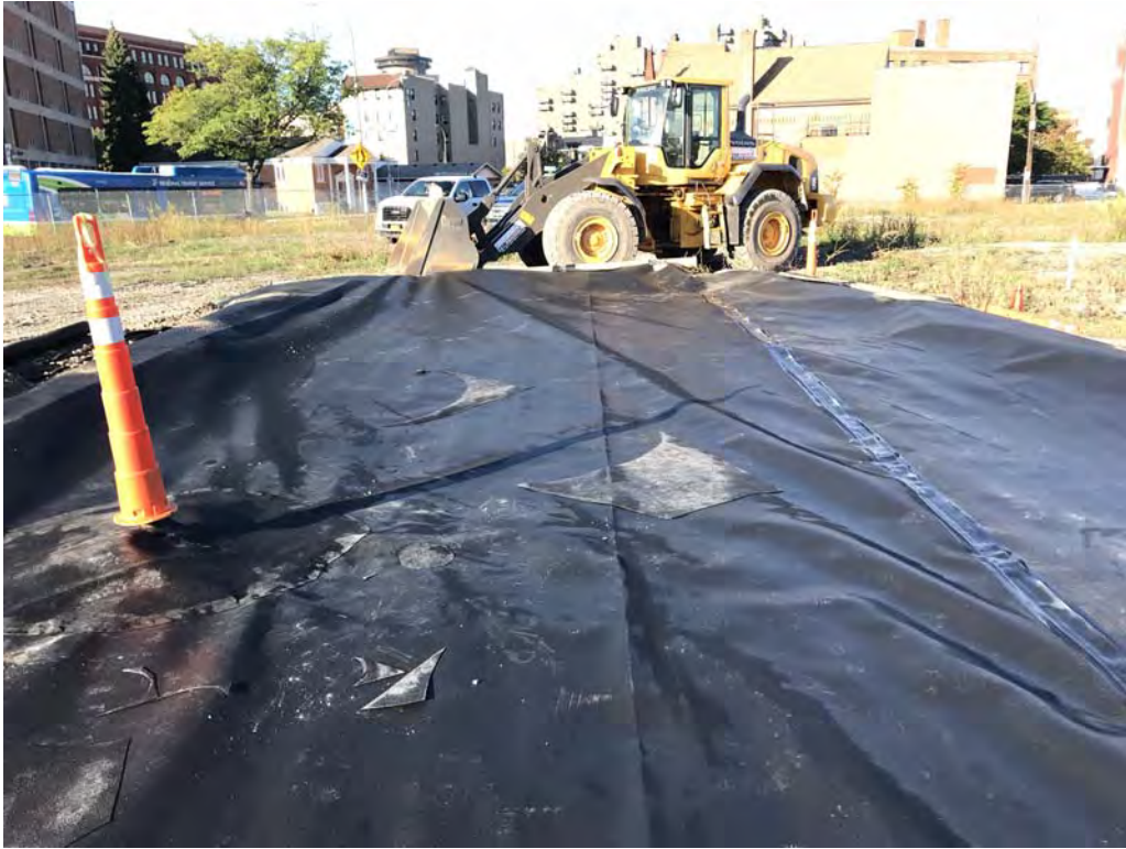
Plastic welded and bermed soil staging area – looking southwest (9-6-2019)
