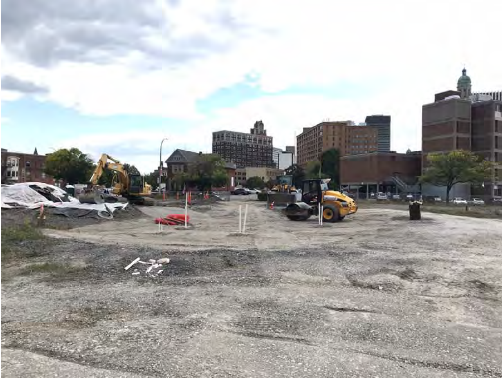
Compacting existing staged crusher run #2 cover system material – looking southeast (9-24-2019)
