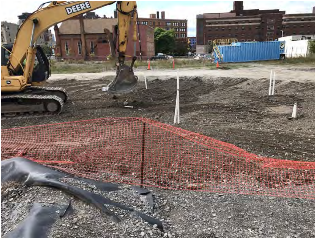
Backfilling with existing staged crusher run #2 cover system material – looking northwest (9-24-2019)
