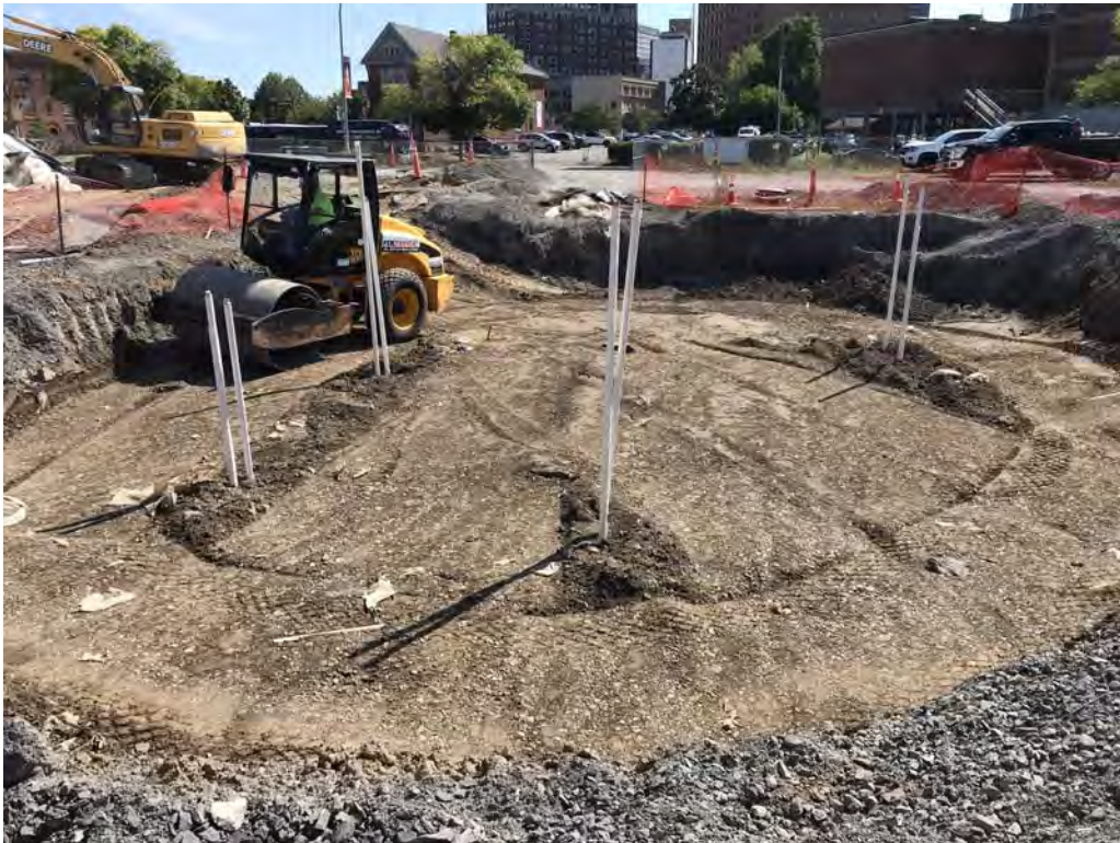
Compacting backfill with vibratory roller – looking southeast (9-20-2019)
