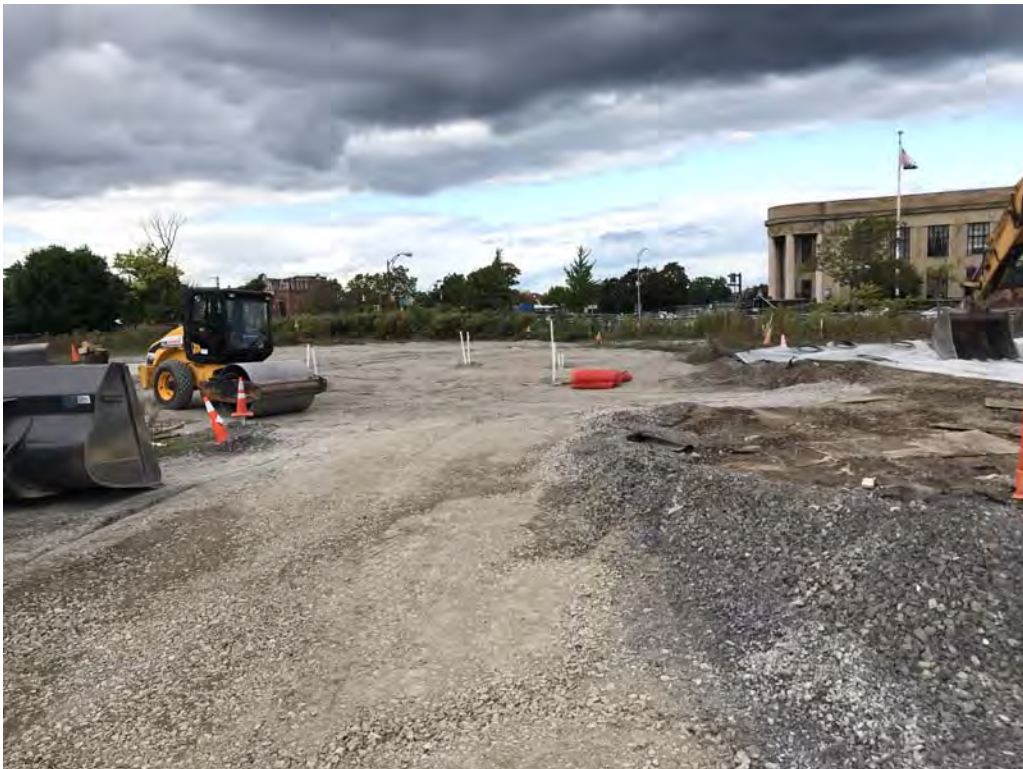
Compacting existing staged crusher run #2 cover system material – looking north (9-24-2019)
