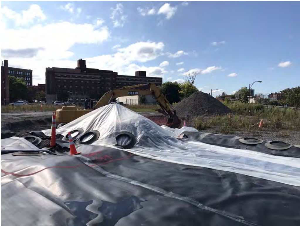
Staging re-usable soil – looking northwest (9-9-2019)
