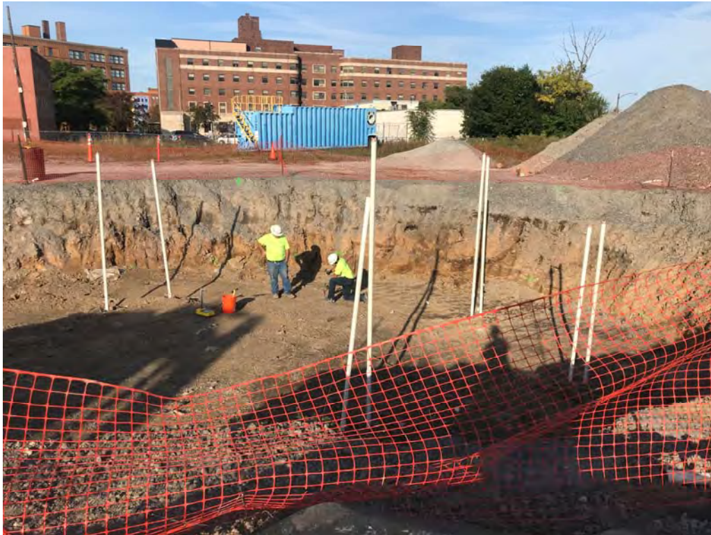
Compaction testing backfill – looking northwest (9-20-2019)
