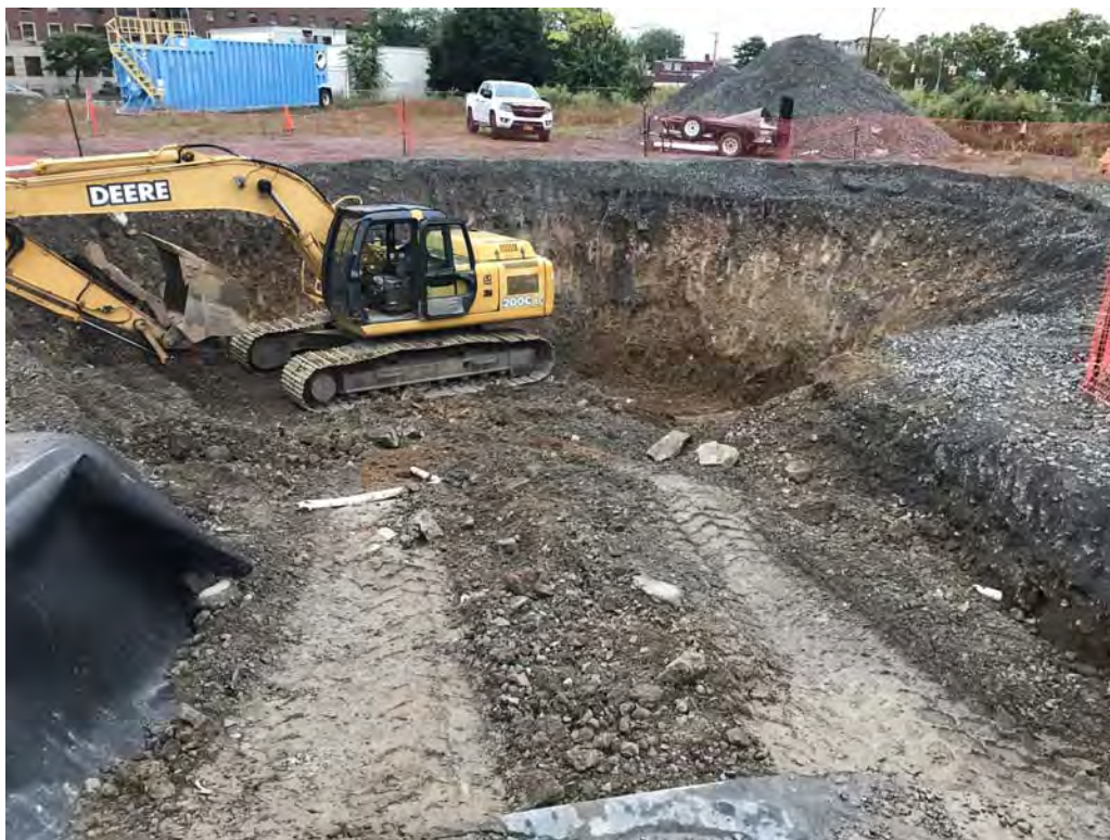
Ramp into soil removal excavation – looking northwest (9-12-2019)
