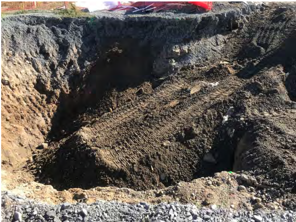
Backfilling excavation using re-usable Site soil – looking east (9-17-2019)
