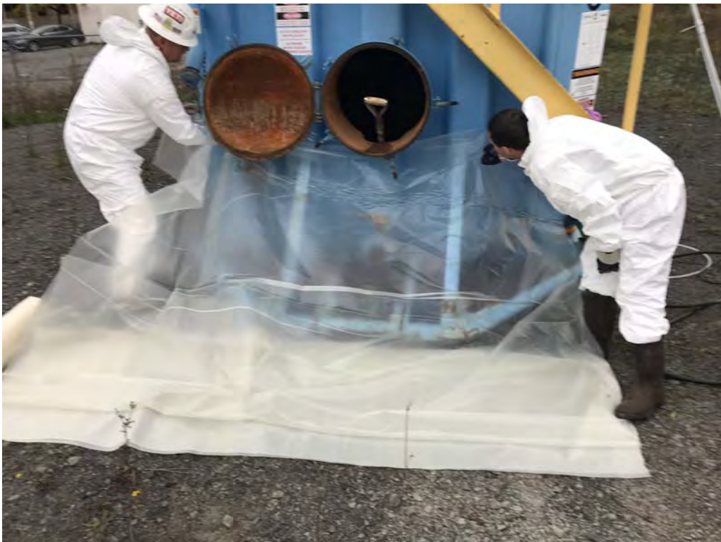
Clean out of frac tank – looking north (10-22-2019)
