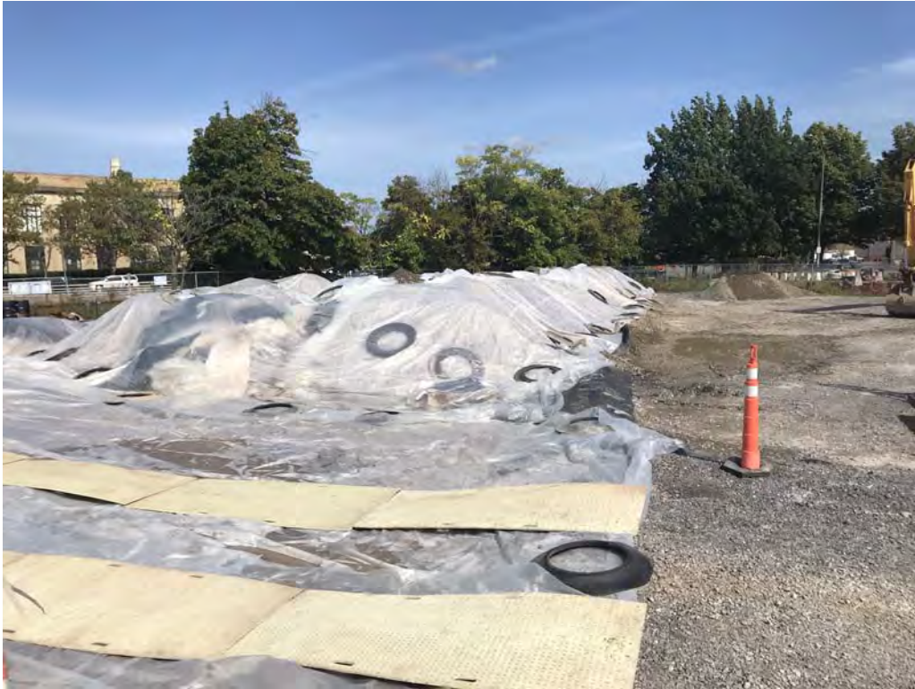
Staged contaminated soil piles pending disposal facility approvals – looking east (9-25-2019)
