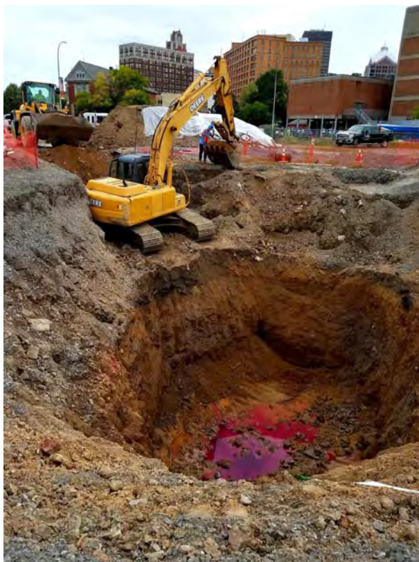
Removal of targeted contaminated soil nearing completion – looking southeast (9-13-2019)
