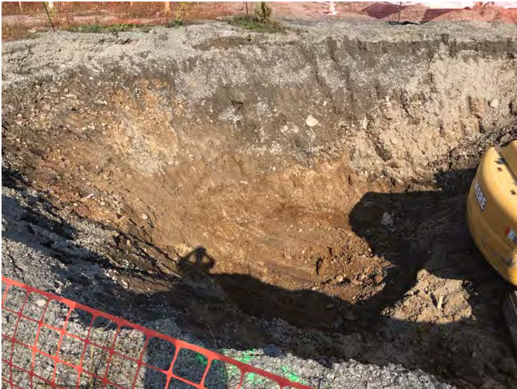
Start removing contaminated soil from north end of excavation – looking east (9-11-2019)
