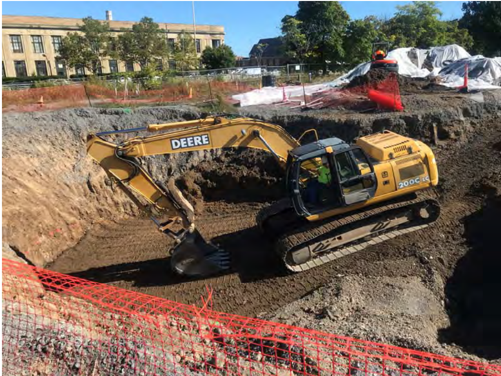
Backfilling excavation using re-usable Site soil – looking northeast (9-17-2019)
