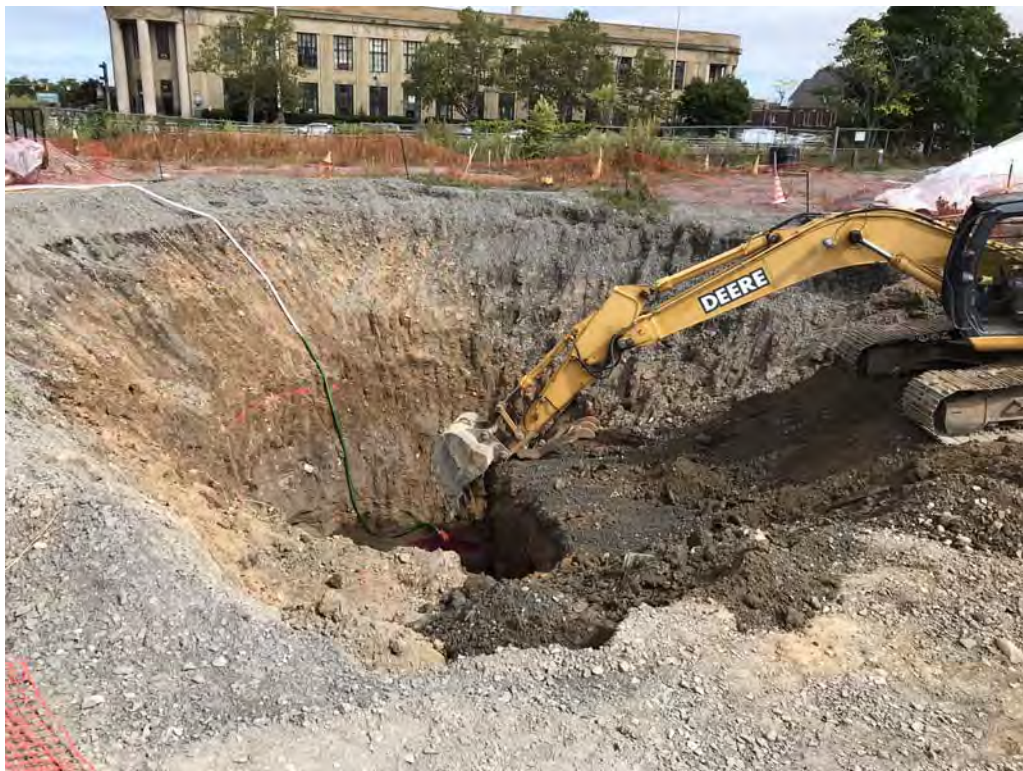
Contaminated soil removal with concurrent excavation dewatering – looking northeast (9-13-2019)
