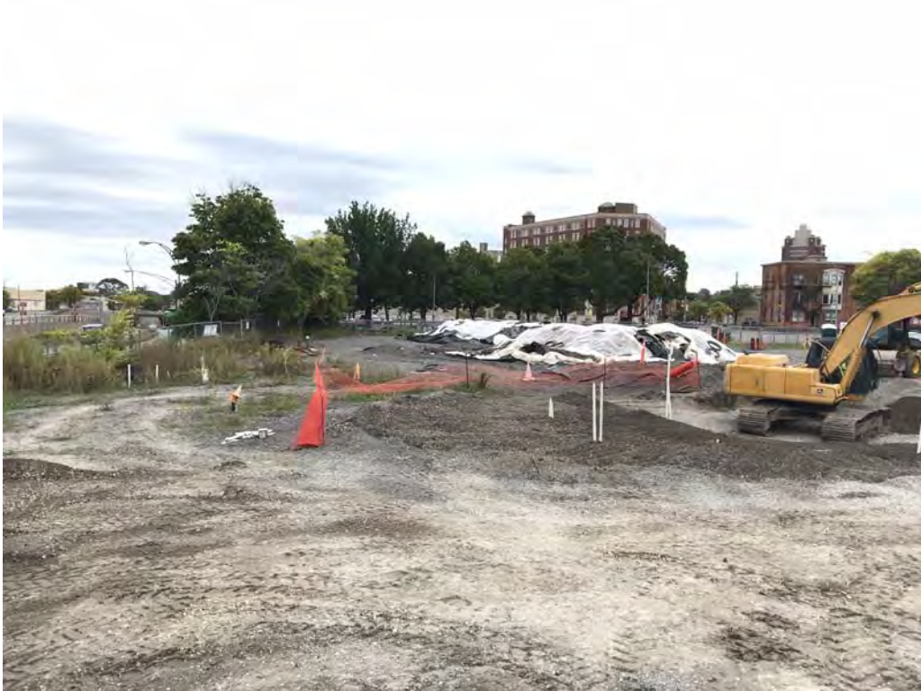
Backfilling with existing staged crusher run #2 cover system material – looking southeast (9-24-2019)
