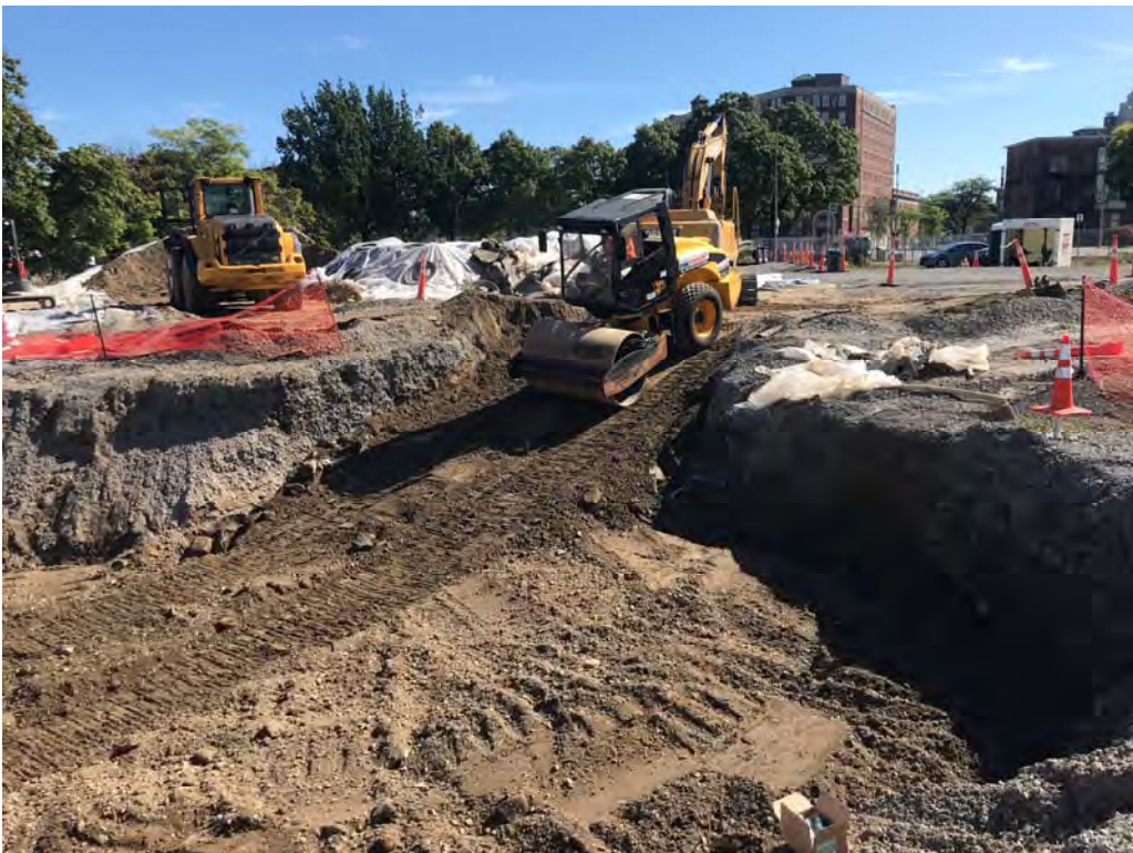
Vibratory roller entering ramp to compact backfill – looking southeast (9-19-2019)
