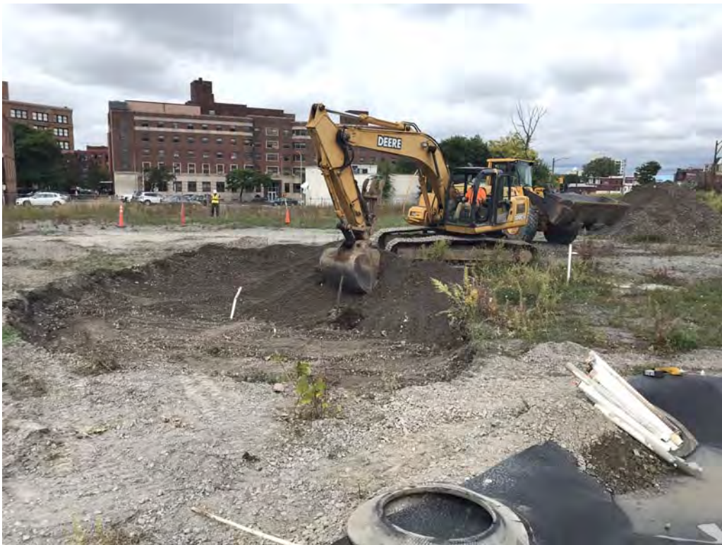
Removing and staging earthen cover system material – looking northwest (9-9-2019)
