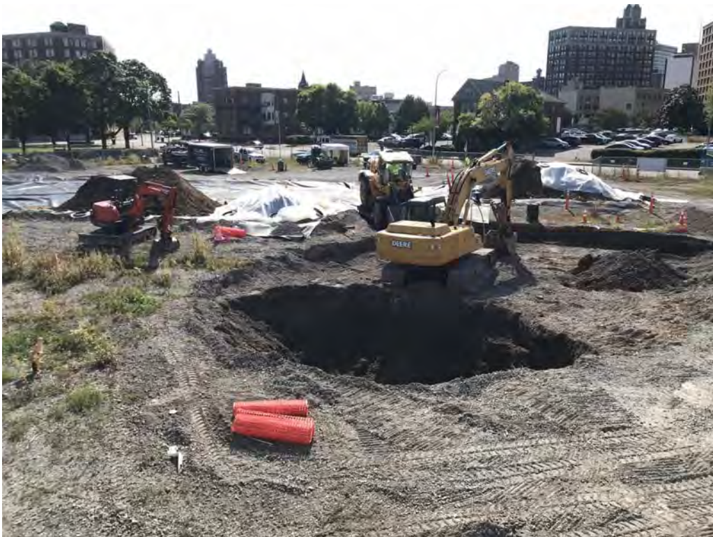
Excavating/staging re-usable soil – looking southeast (9-10-2019)
