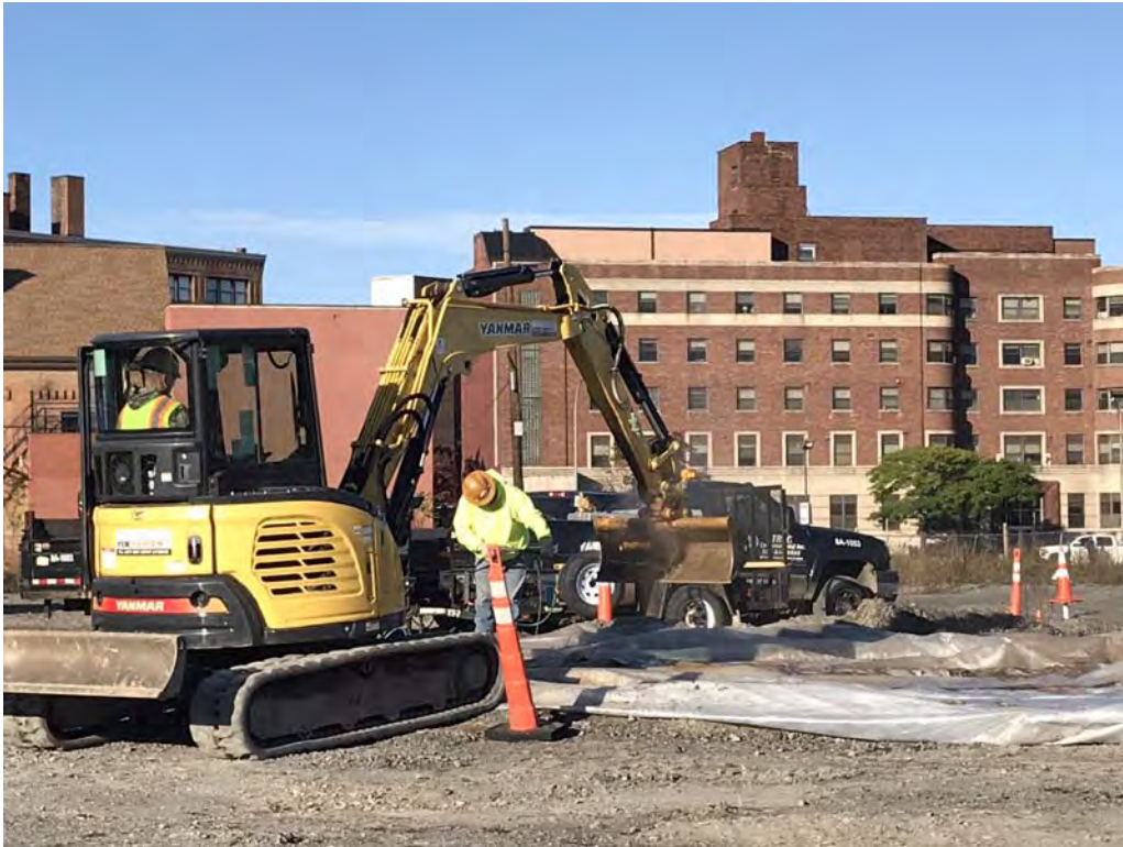
Decontaminating mini-excavator – looking west (10-11-2019)
