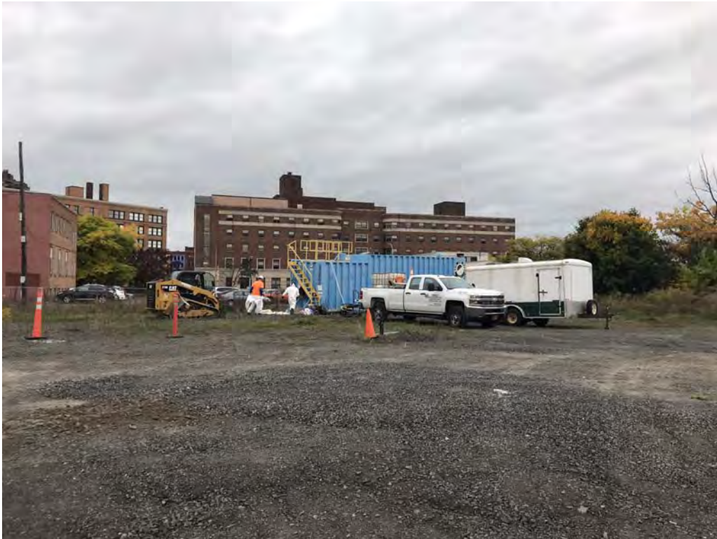
Clean out of frac tank – looking northwest (10-22-2019)
