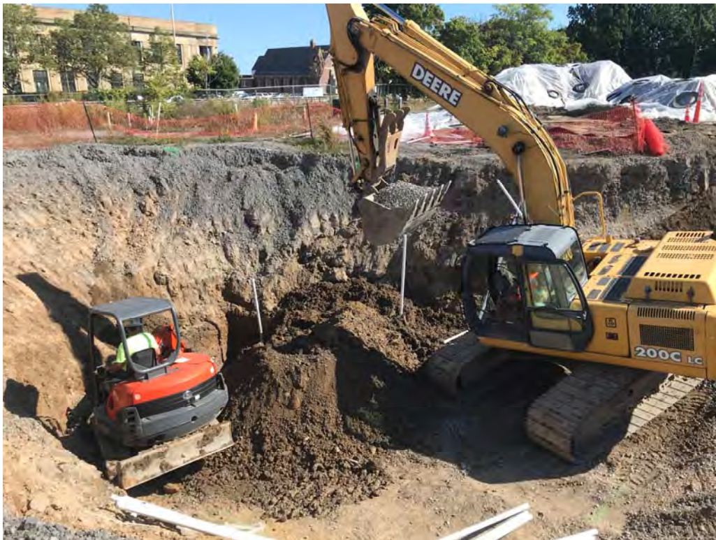
Installing ISCO piping in trench within partial backfill – looking northeast (9-18-2019)
