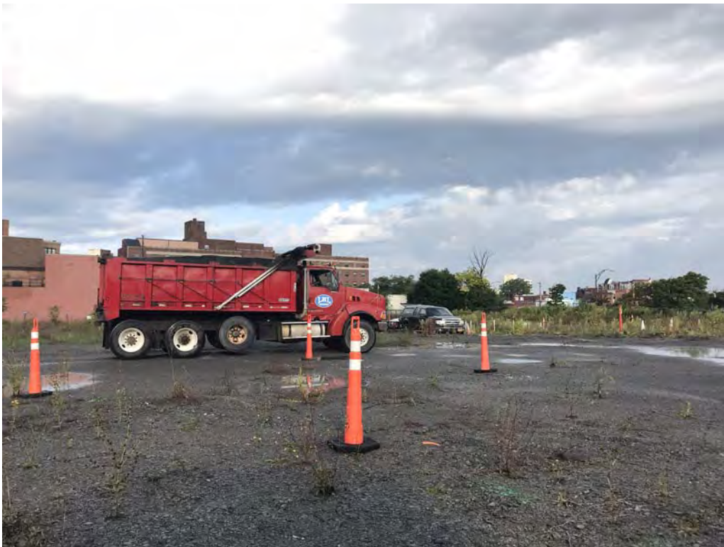
Delivery of imported crusher run #2 (CR2) – looking northwest (9-4-2019)
