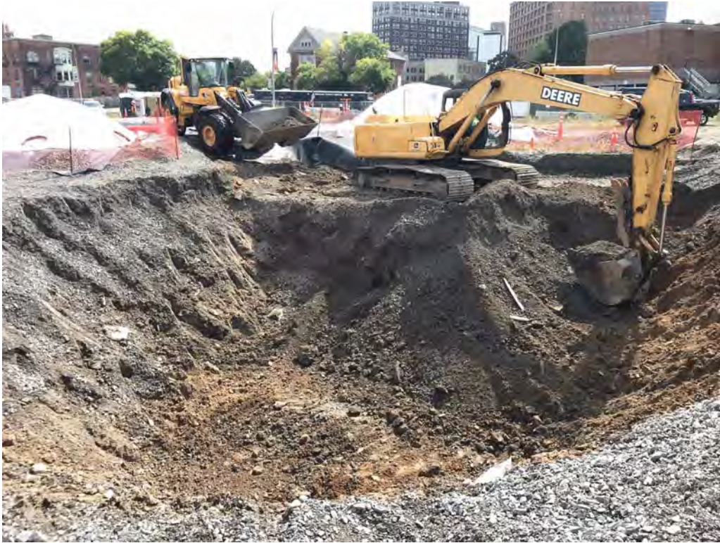
Excavating re-usable soil – looking southeast (9-11-2019)
