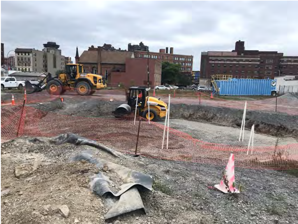
Compacting imported crusher run #2 – looking southwest (9-23-2019)
