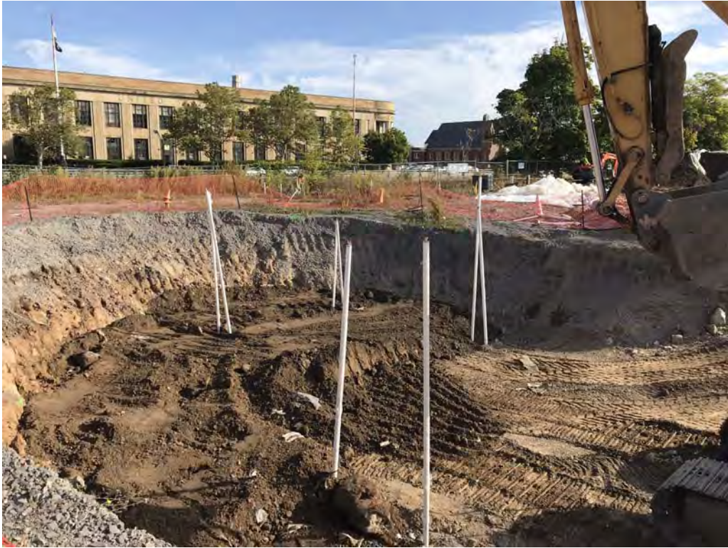
Backfilling around ISCO riser piping in excavation – looking northeast (9-20-2019)
