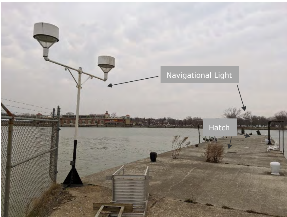
Figure 2.5. Pier South of Sheriff Station: Navigational Lights
