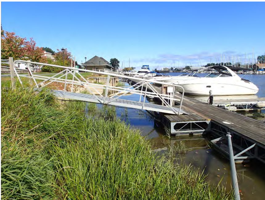
Figure 2-12. Existing Floating Docks in Zone E
