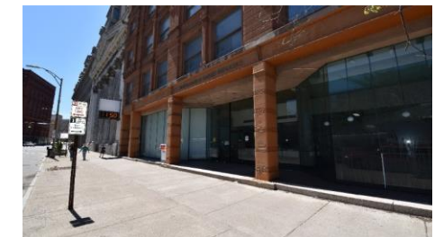
Figure G: ADA accessibility is prevented by steps at many building thresholds, view south.
