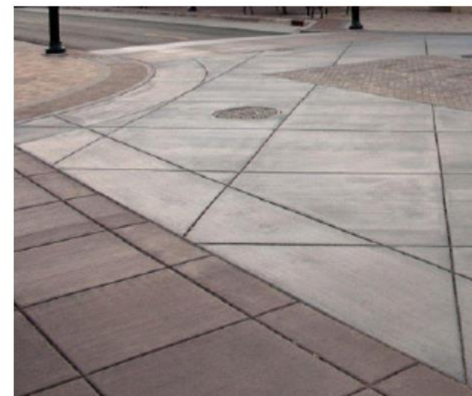
Pavement Scored Concrete Paving with Integrally Colored Concrete Accents
