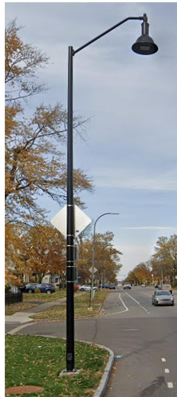
Light Pole and Fixture Cyclone "Domia"
