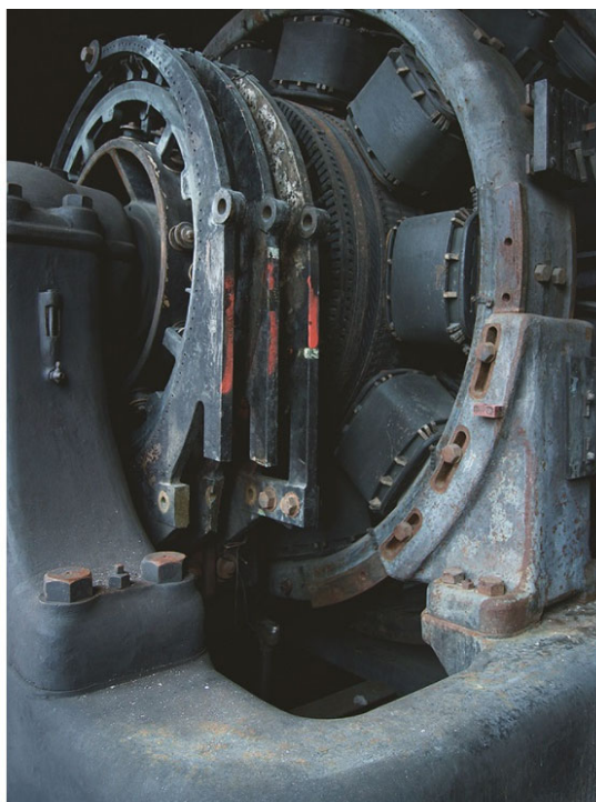
RG&E Beebe power station prior to demolition, Rochester, NY, Summer 2016. [IMAGE: Anonymous]
