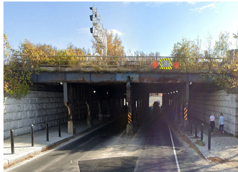
St Paul Underpass Improvements
