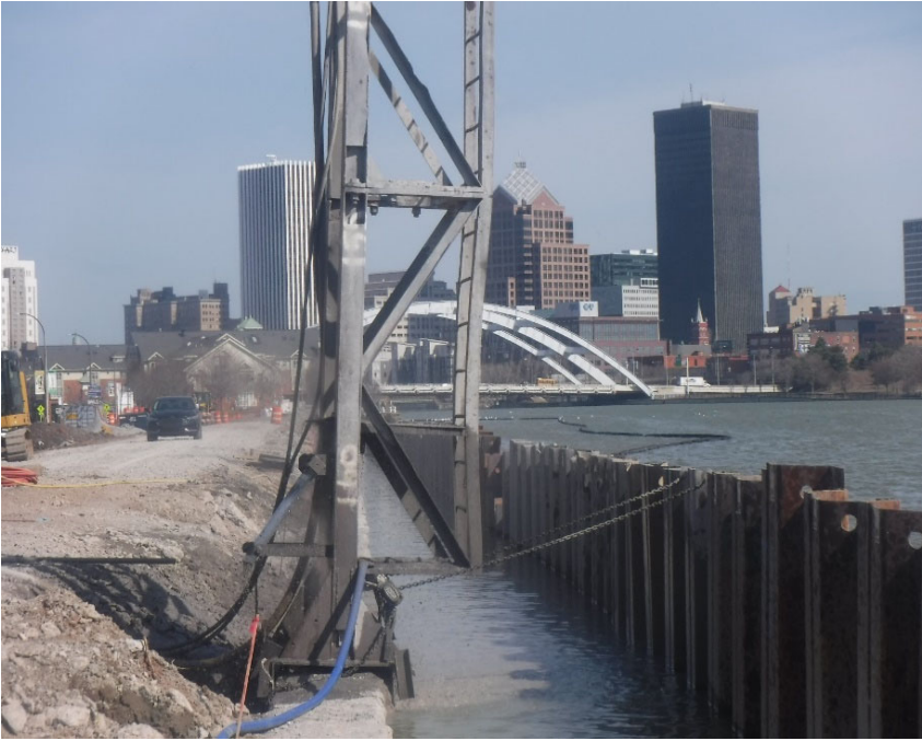
West River Wall – Corn Hill Segment Proposed Completion: 2022
