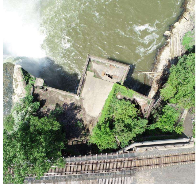
Figure 3 - Drone photo of Station No. 4
