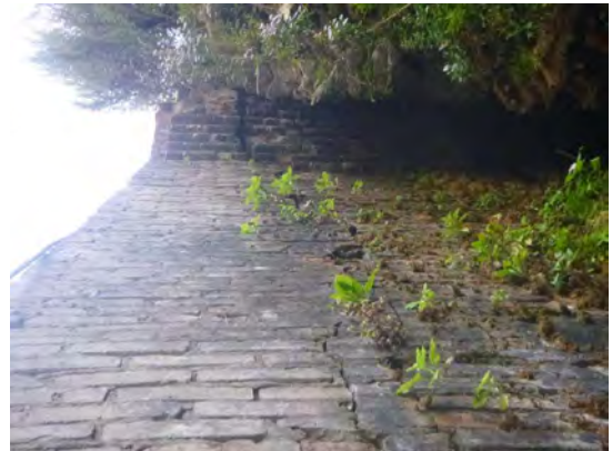
Figure 14 - Horizontal Displacement of Brick
