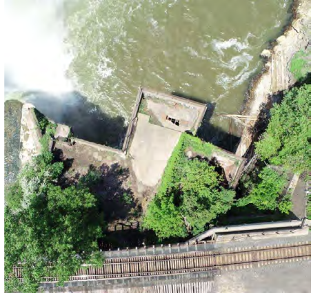
Figure 3 - Drone photo of Station No. 4
