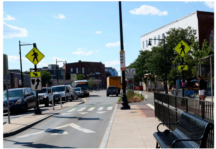
Raised mid-block crossing Somerville, MA featuring flashing beacons (RRFBs) and a pedestrian crossing island, slowing traffic and facilitating bus stop access
