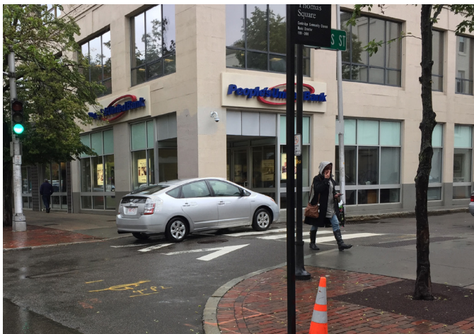
Raised crosswalk along a major road in Cambridge, MA, slowing vehicle turns and improving pedestrian visibility
