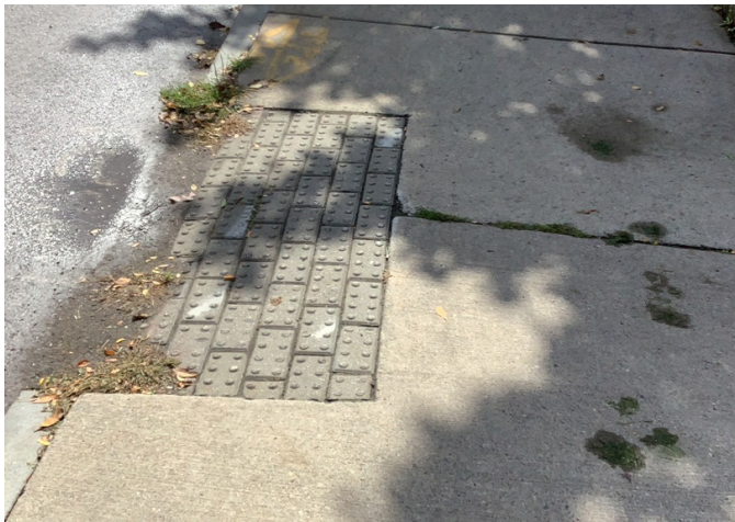
Detectable warning strip on Lake Avenue that does not provide sufficient color contrast
