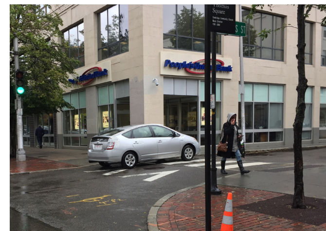
Raised crosswalk along a major road in Cambridge, MA, slowing vehicle turns and improving pedestrian visibility
