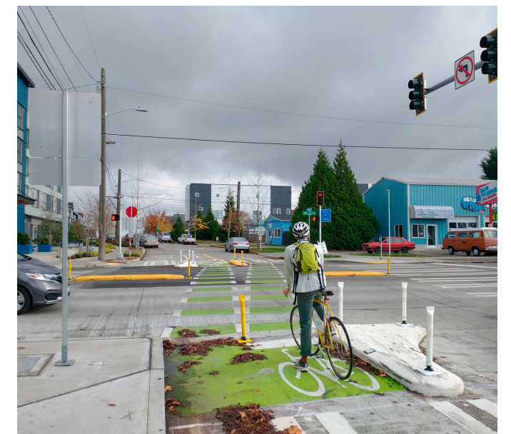
Bike boulevard crossing, including a traffic diverter, at a major road in Seattle, WA
