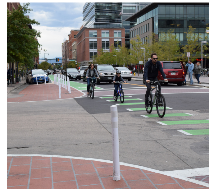
Bike lane crossing, with temporary curb extensions to slow vehicle turns, in Denver, CO
