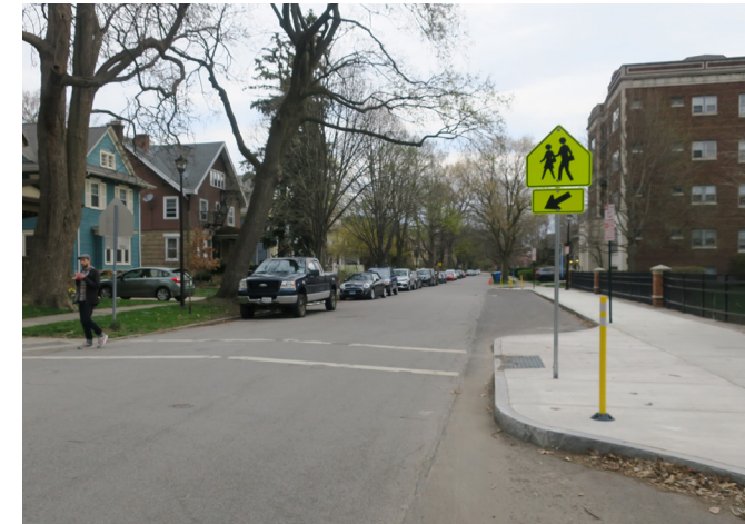
Crosswalk in front of a Rochester school with a curb extension, shortening crossing length and improving pedestrian visibility
