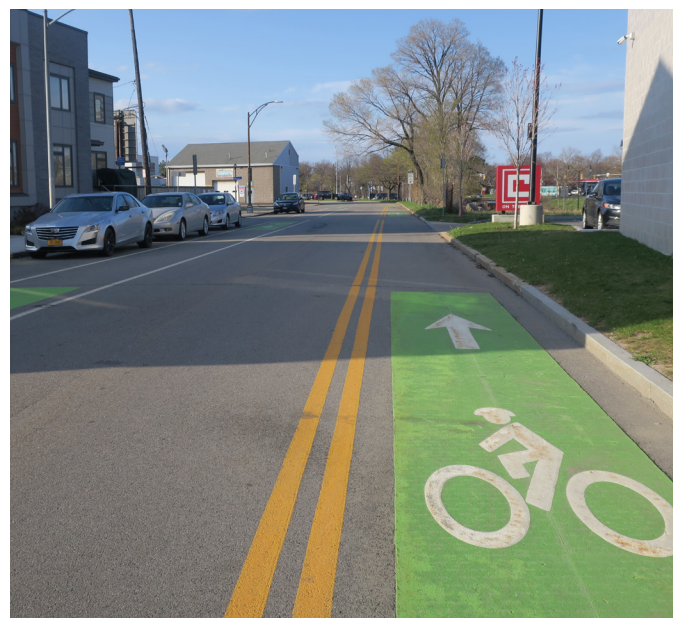
Contraflow bike lane in Rochester, creating a two-way bike connection on a one-way street
