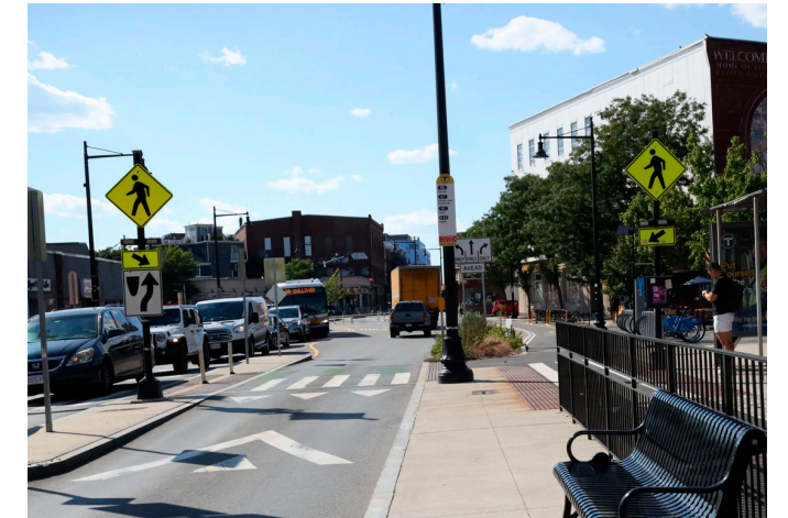
Raised mid-block crossing Somerville, MA featuring flashing beacons (RRFBs) and a pedestrian crossing island, slowing traffic and facilitating bus stop access
