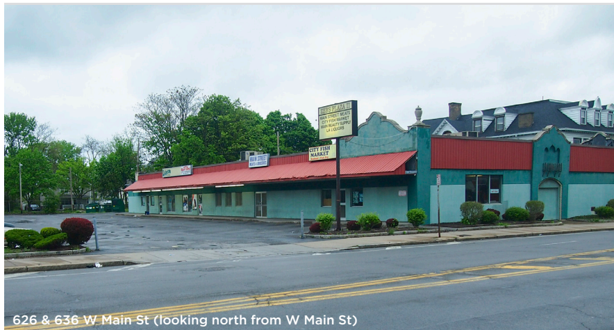
626 & 636 W Main St (looking north from W Main St)
