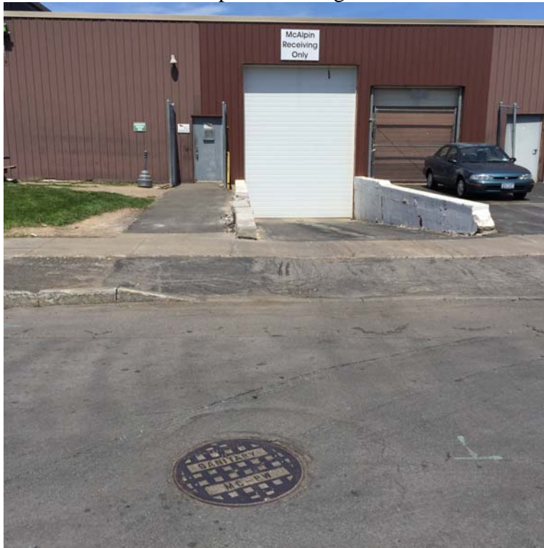
Manhole 1 (MH-1), located south of the Site in Balfour Drive, looking north.
