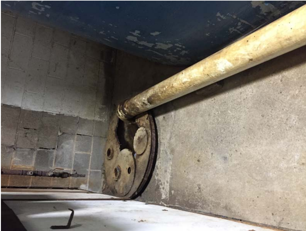
Sump #2, located south of the water treatment plant
