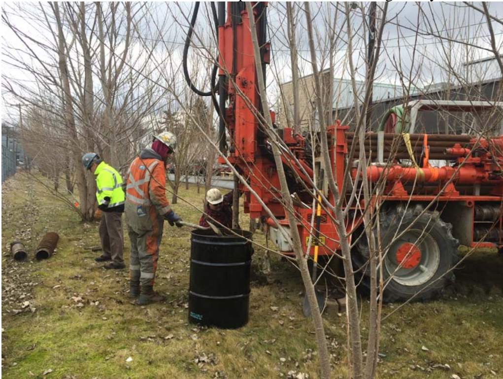
Installation of bedrock monitoring well MW-10R
