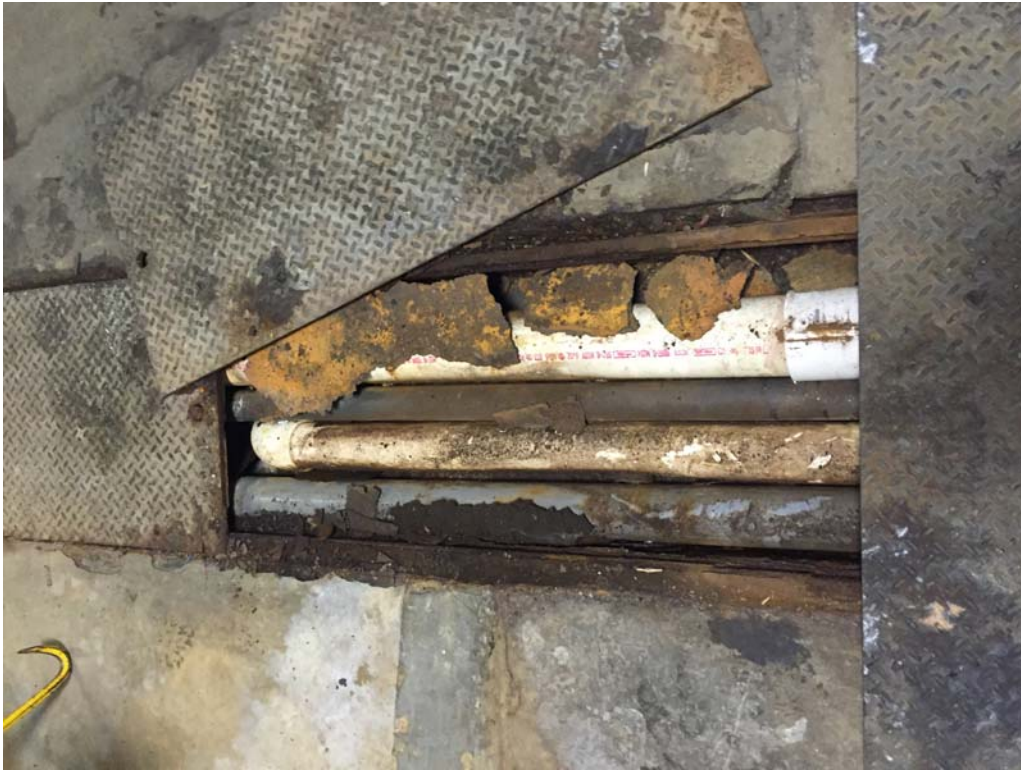
Pipe chase within northern portion of main building
