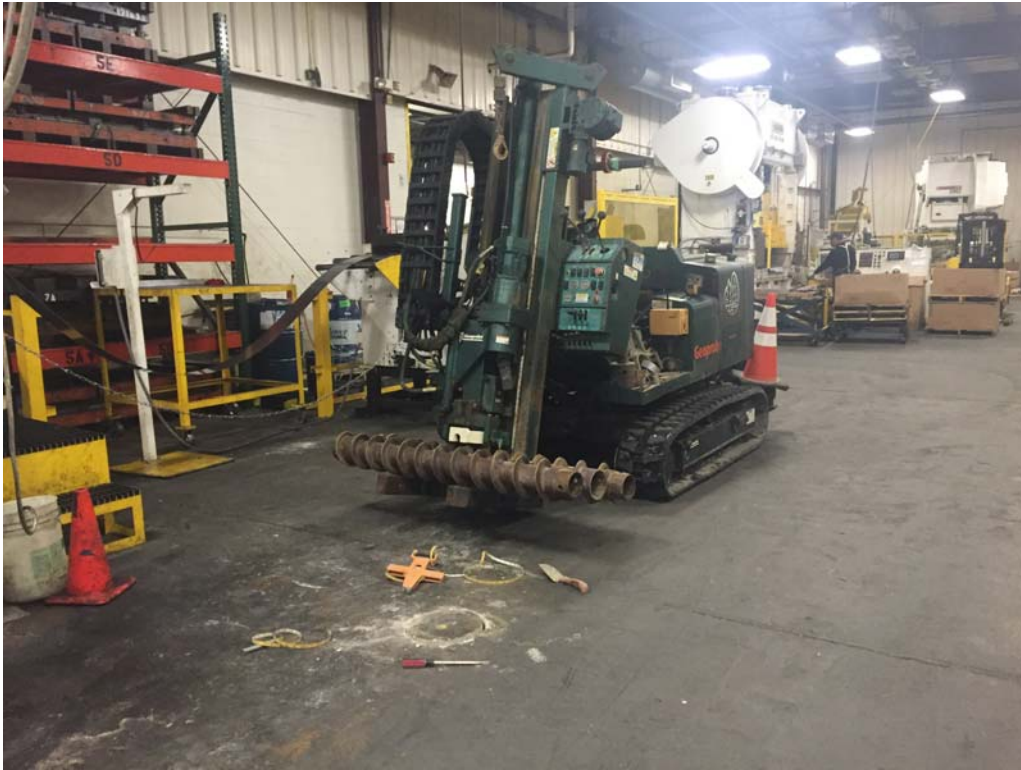
TREC track-mounted Geoprobe drill rig within the main building
