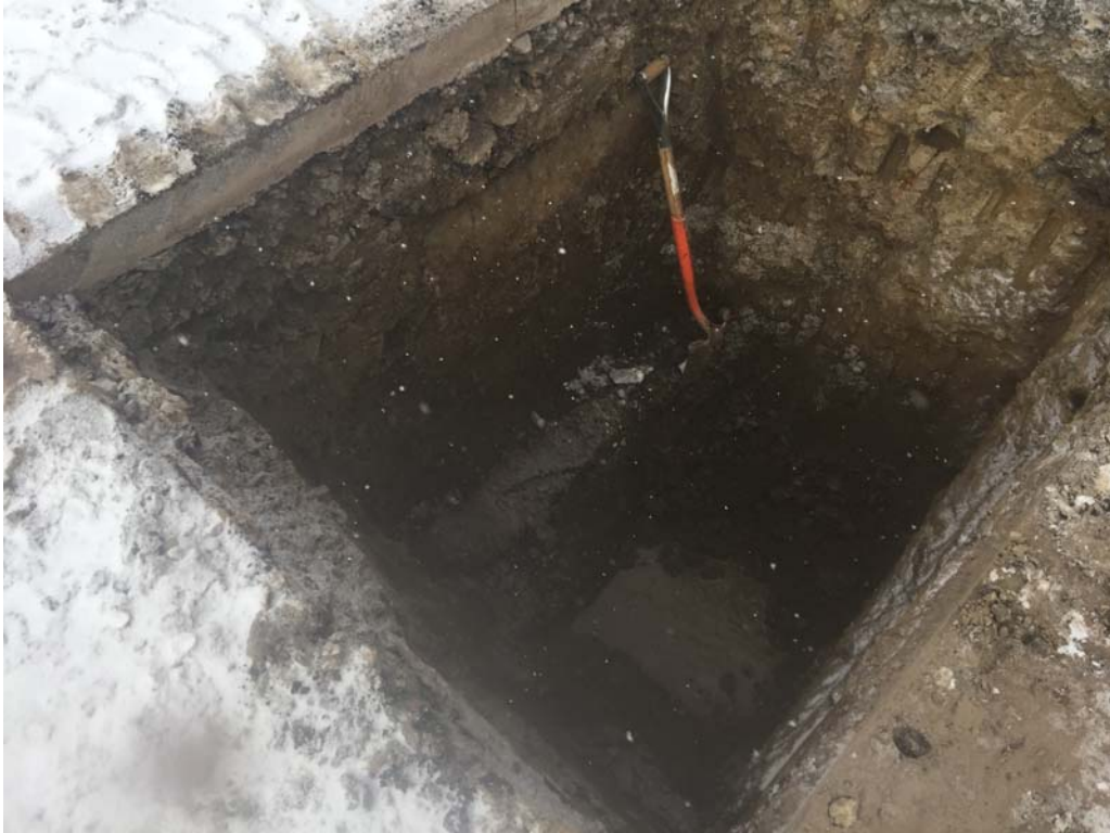
Excavated area of damaged sewer line (i.e., original location of MW-19)
