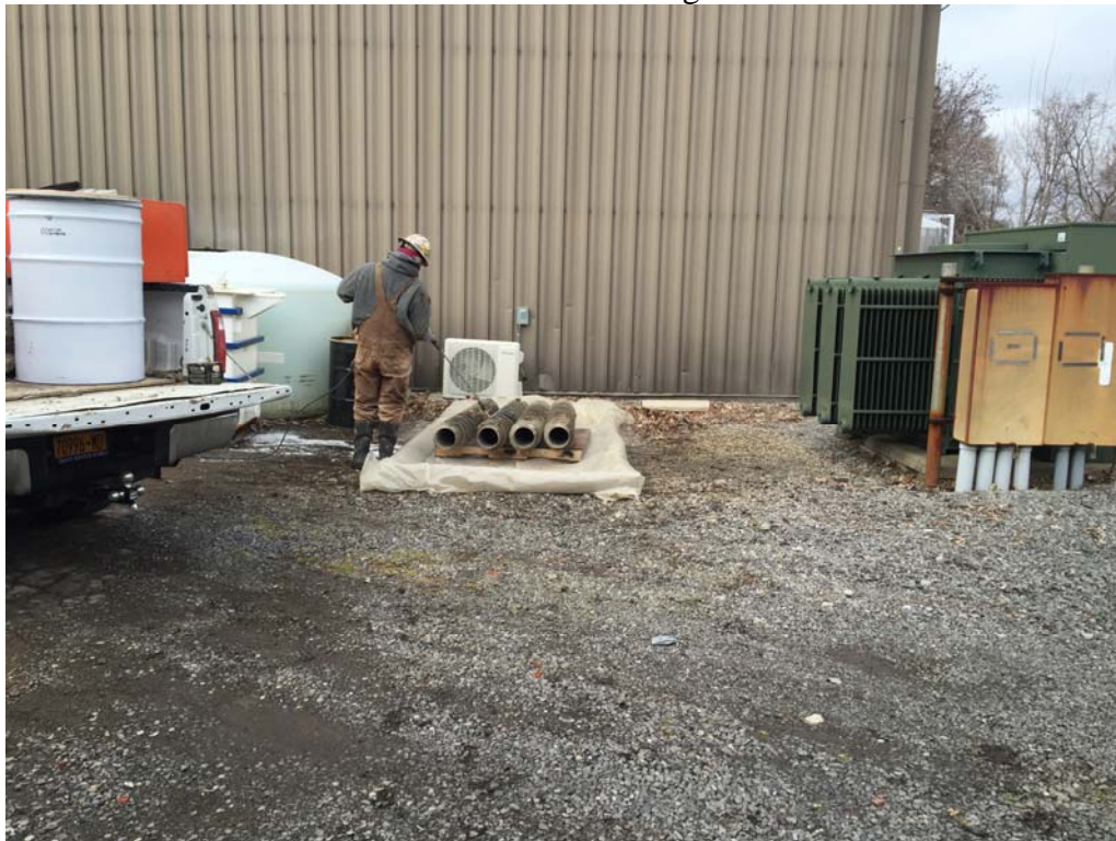
Decontamination pad set up by Applus in north courtyard area
