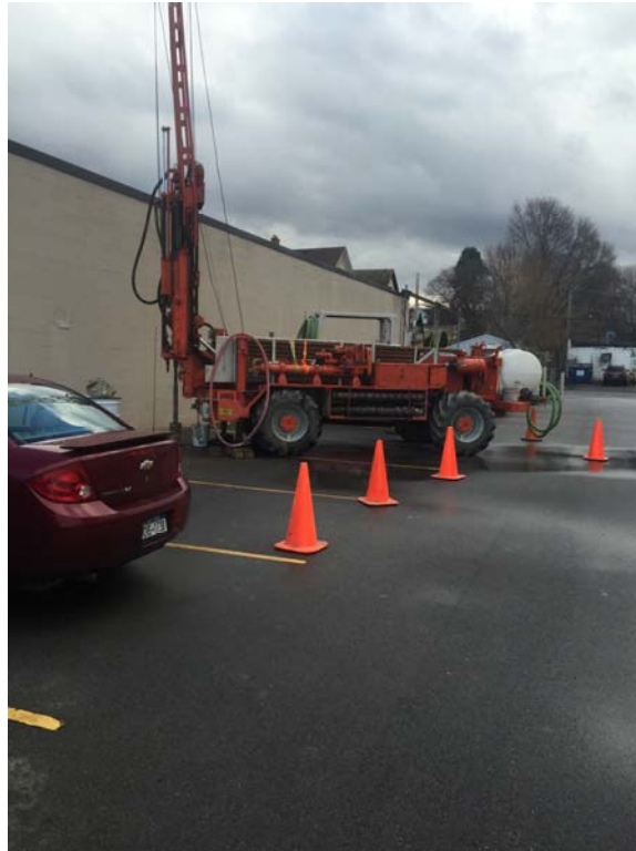
Installation of bedrock monitoring well MW-12R
