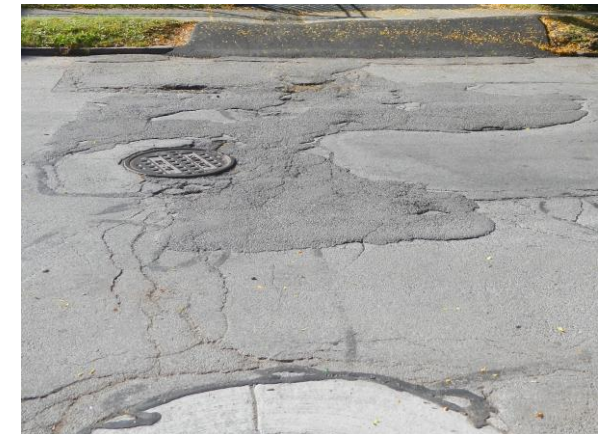
Emerson Street Pavement
