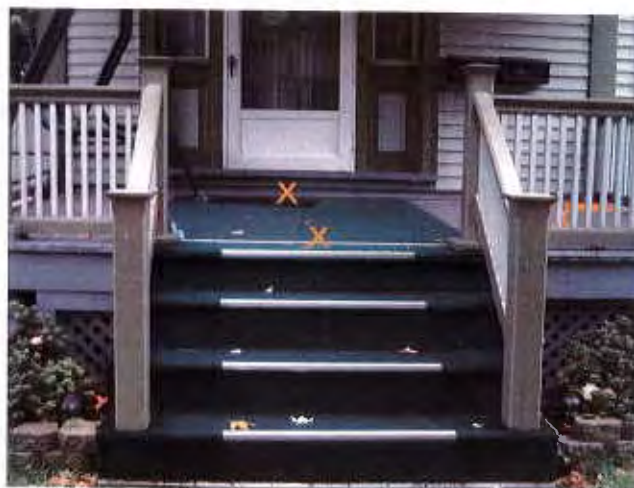
Fig. 1. Typical exterior porch in Rochester, New York (X=dust wipe sampling locations; square=location of dust collection plate).
