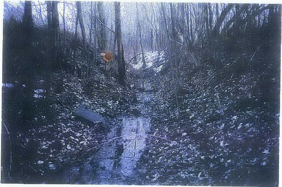
PHOTO 1. Channelized intermittent ditch (Wetland A). Note extensive fill bordering both sides of the channel.
