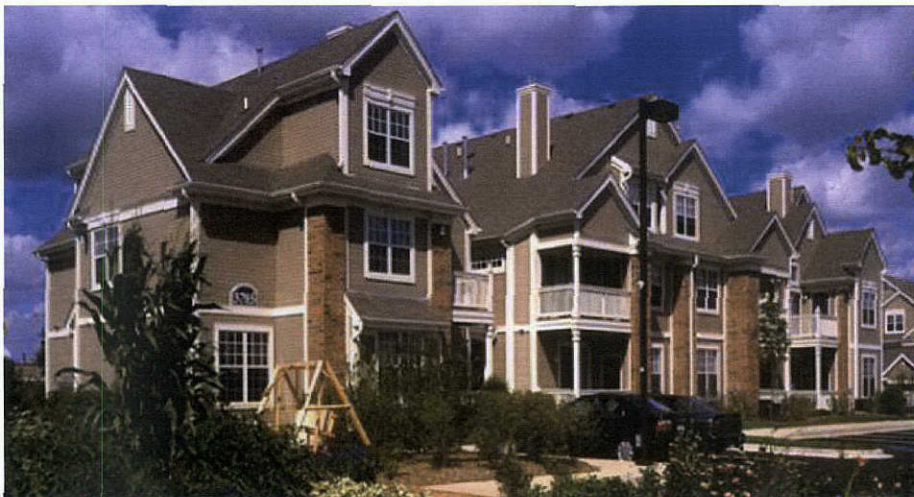
FIGURE 13 Use of materials enhance the architectural massing of the building
