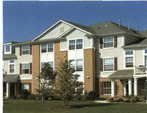
FIGURE 12 Accents used to enhance facade
