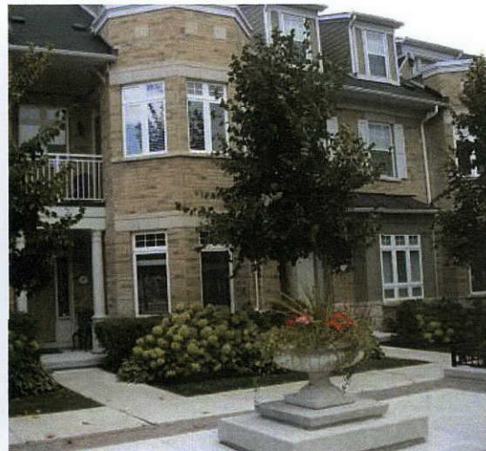
FIGURE 16 Articulation of wall surfaces include bay windows, balconies, and dormers
