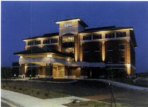
FIGURE 10 Portico and vertical entry feature
