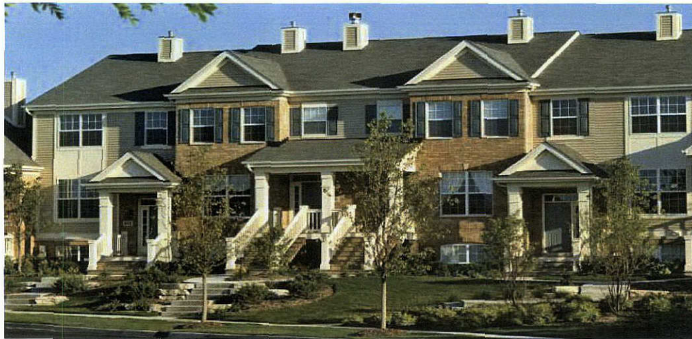
FIGURE 10 Facade is articulated to create interest and is visually divided into smaller sections
