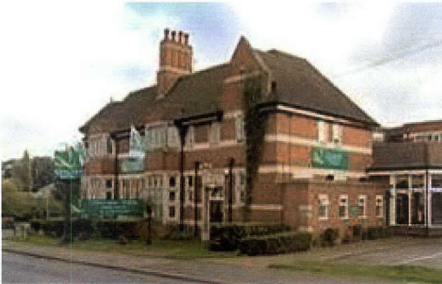
FIGURE 8 Natural materials used on facade
