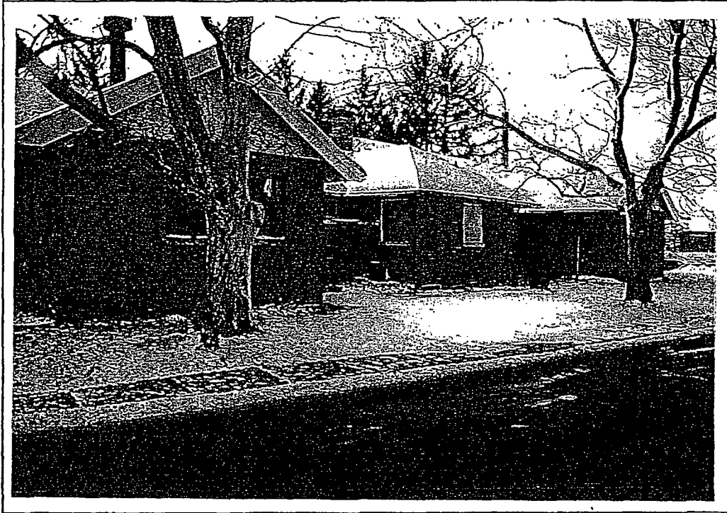
17 Building 4, service wings at north side.
