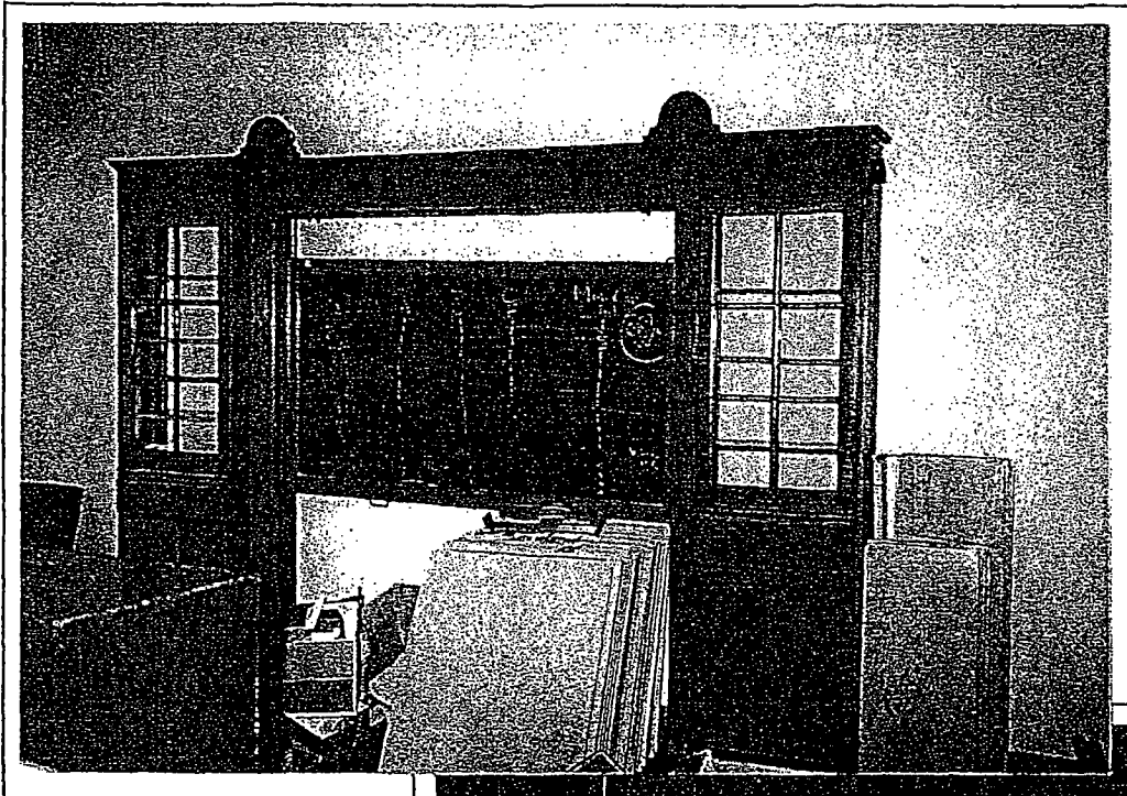
35 Building 5, classroom chalkboard at east wing.
