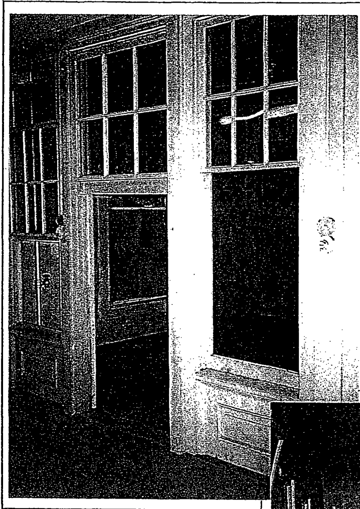
15 Building 4, windows and door between patient room and porch.
