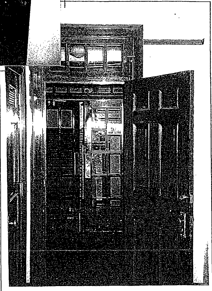
10. Building 1, typical oak six-panel door and stair beyond.
