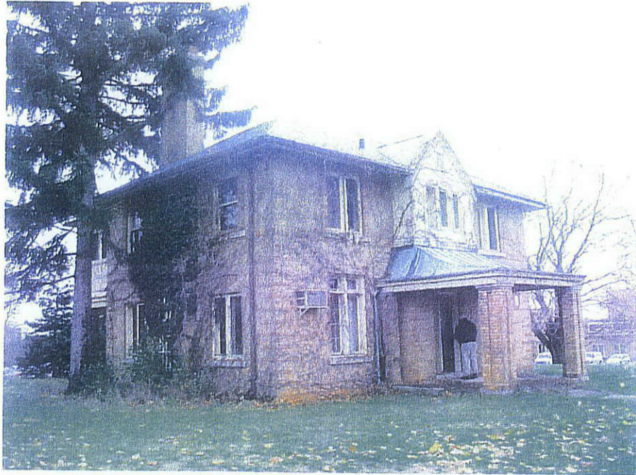
Photo 19 Looking at Building - 8.
