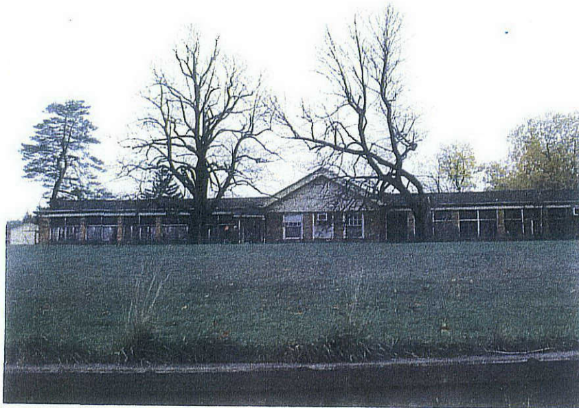
Photo 21 Looking at Building - 9.
