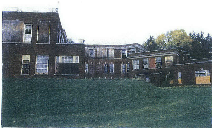
Photo 8 Looking at the south-west corner of Building – 5.
