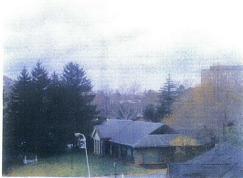
Photo 6 Looking at Building - 4.
