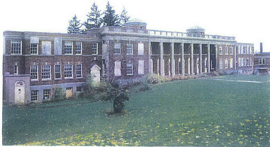
Photo 7 Looking at the West elevation of Building – 5.
