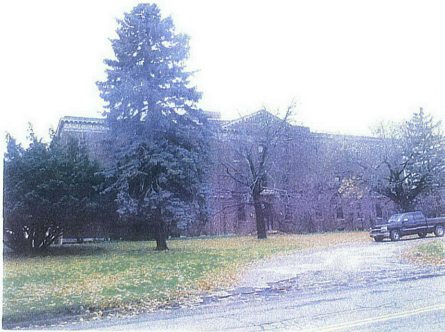
Photo 1 Looking at Building – 1.
