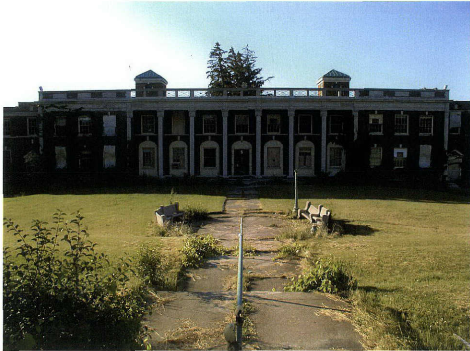
Photograph 31: View of Structure 11 (i.e., the children's building), presently abandoned, facing southeast.
