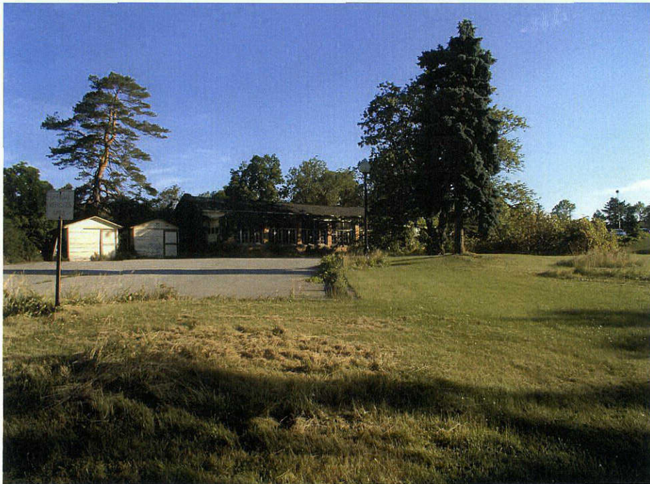
Photograph 20: View of Structure 6 (i.e., Pavilion A), presently abandoned, facing north.
