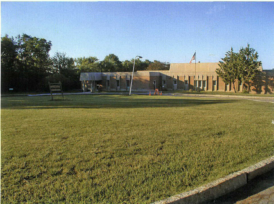
Photograph 36: View of Structure 15, presently a children's detention center, facing south.
