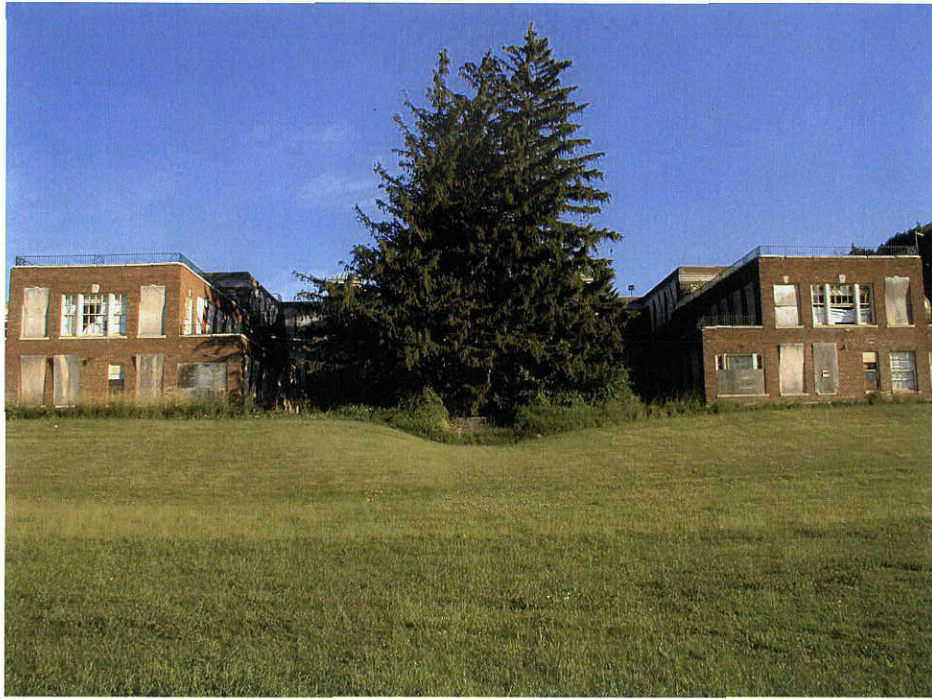
Photograph 29: View of Structure 11 (i.e., the children's building), presently abandoned, facing northwest.
