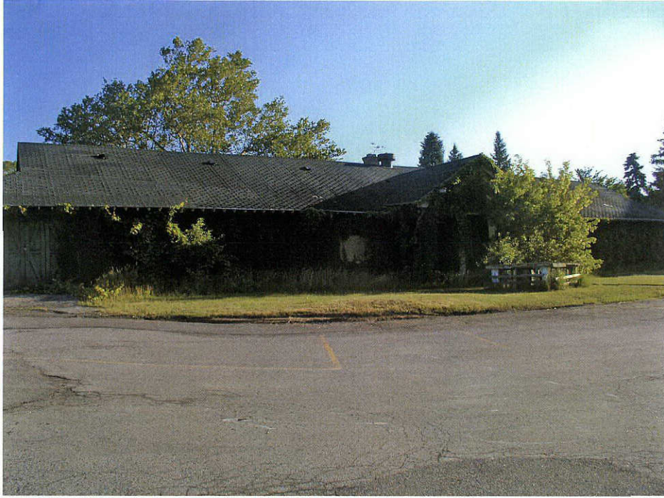
Photograph 23: View of Structure 8 (i.e., Pavilion C), presently abandoned, facing north.
