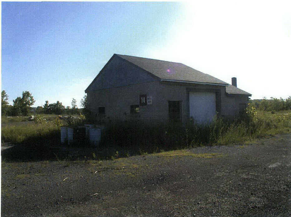
Photograph 40: View of Structure 18, presently abandoned, facing northeast.
