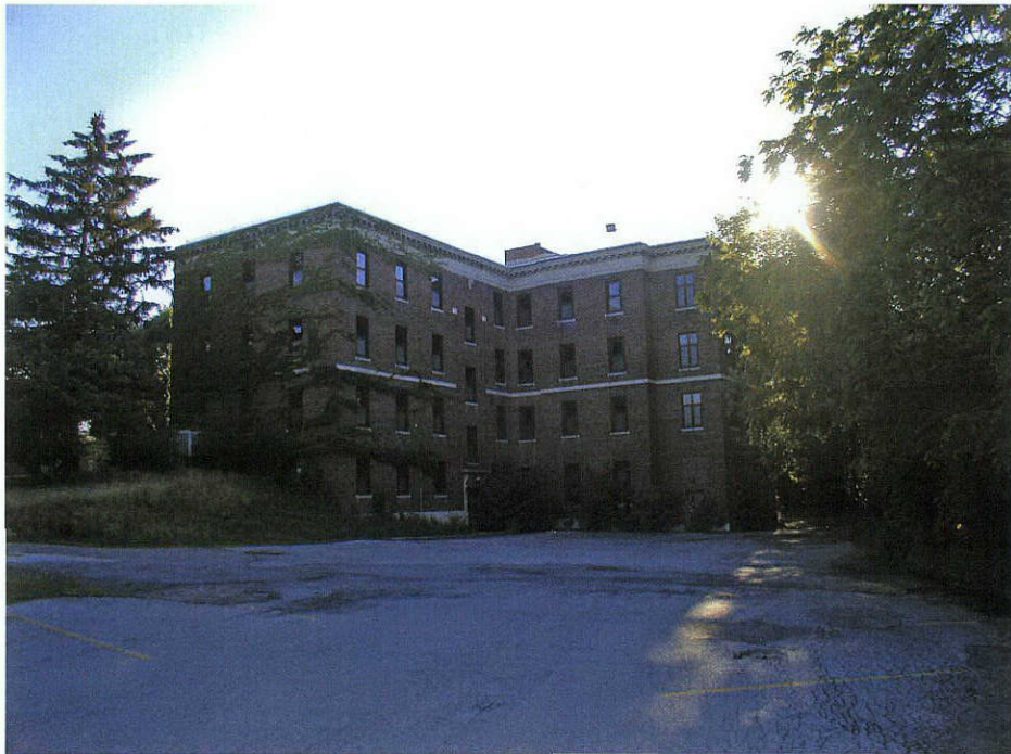
Photograph 26: View of Structure 10 (i.e., the nurse's home), presently abandoned, facing northeast.
