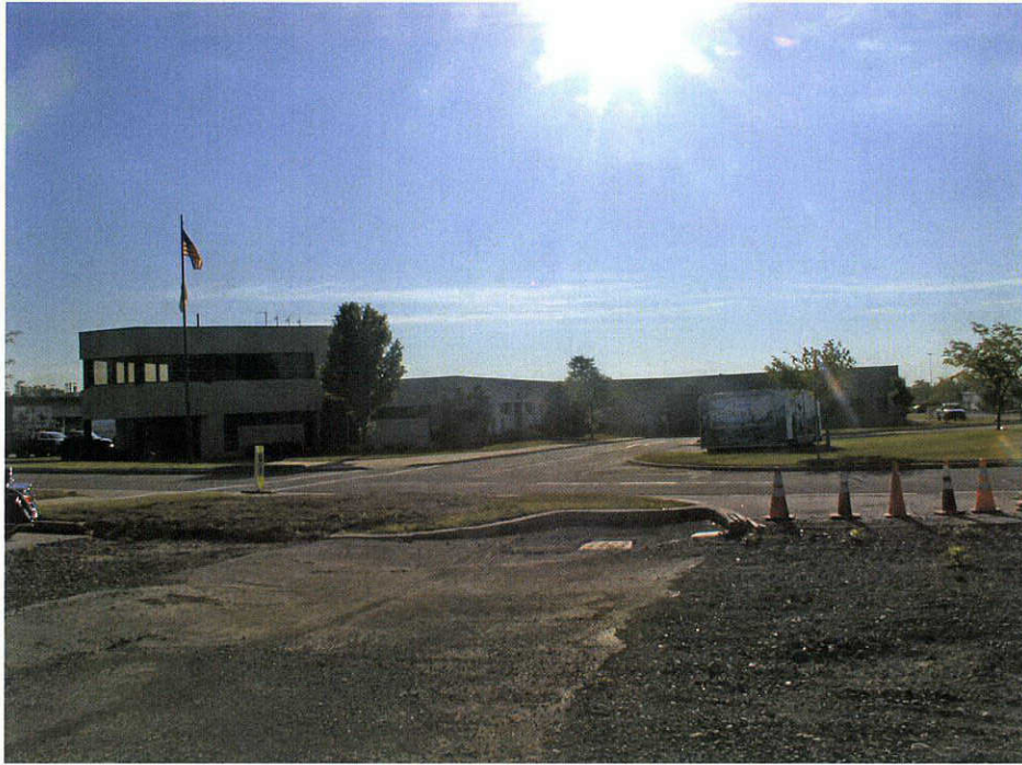
Photograph 37: View of Structure 16, presently a Monroe County recycling center, facing northeast.
