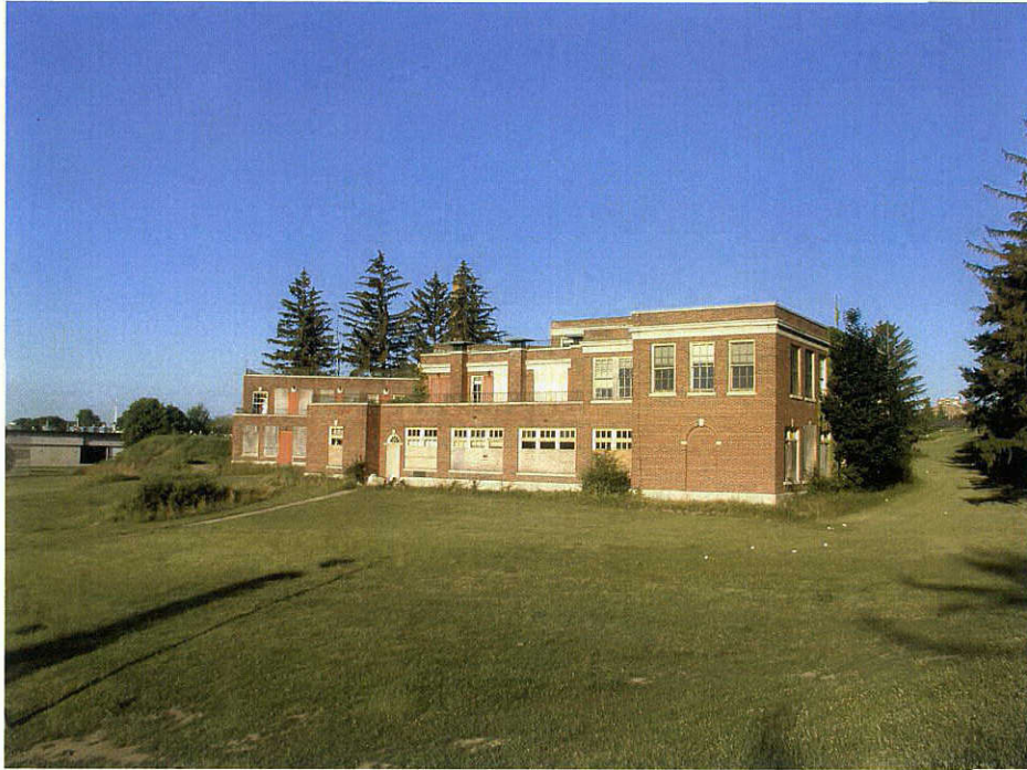
Photograph 27: View of Structure 11 (i.e., the children's building), presently abandoned, facing southwest.
