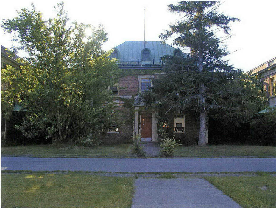
Photograph 33: View of Structure 13 (i.e., a staff building), presently abandoned, facing east.
