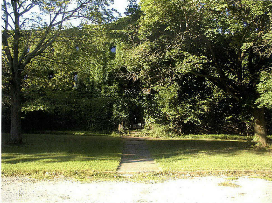
Photograph 25: View of Structure 10 (i.e., the nurse's home), presently abandoned, facing south.
