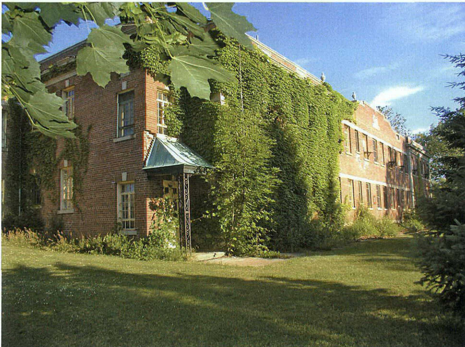
Photograph 34: View of Structure 13 (i.e., a staff building), presently abandoned, facing northwest.
