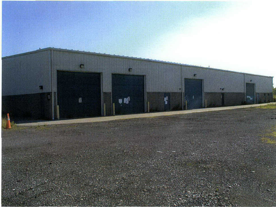
Photograph 39: View of Structure 17, facing northeast.
