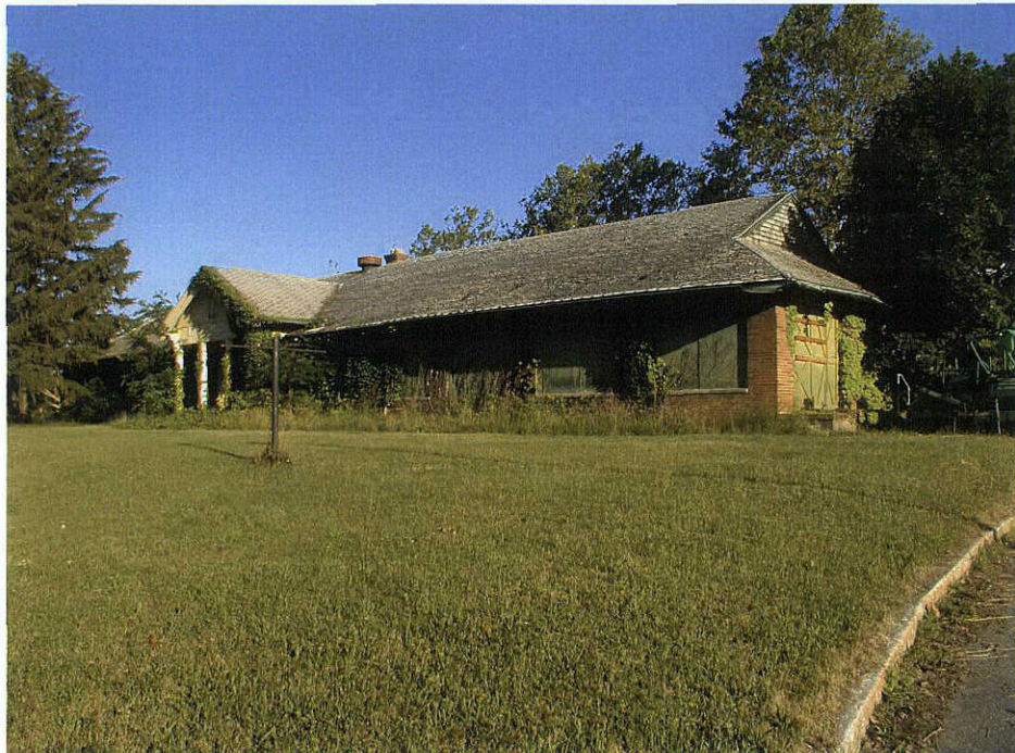
Photograph 22: View of Structure 7 (i.e., Pavilion B), presently abandoned, facing northwest.
