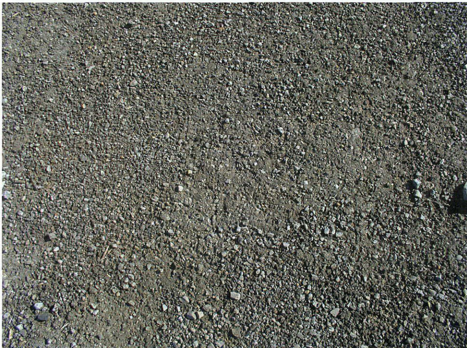
Photograph 48: Close-up view of typical untested area of gravel.
