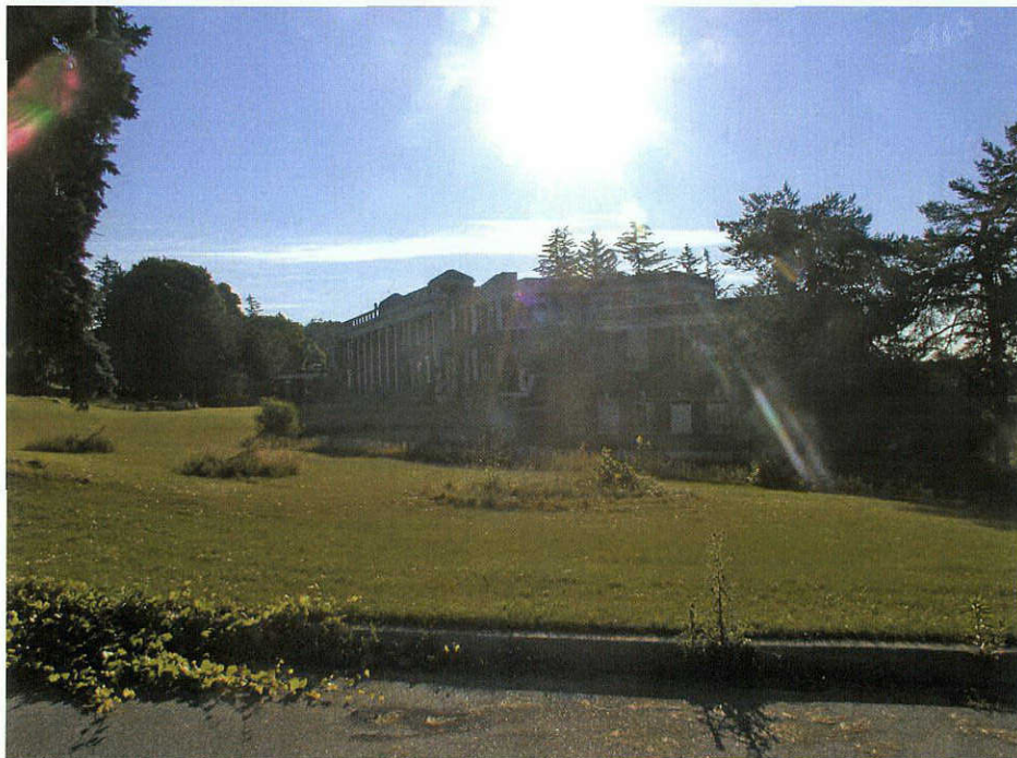
Photograph 30: View of Structure 11 (i.e., the children's building), presently abandoned, facing southeast.
