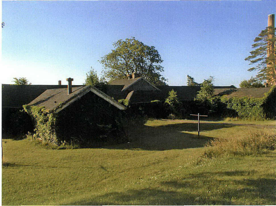
Photograph 21: View of Structure 6 (i.e., Pavilion A), presently abandoned, facing south.
