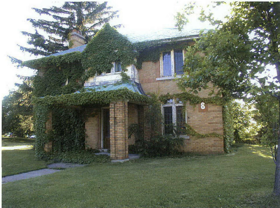
Photograph 32: View of Structure 12, presently abandoned, facing northeast.
