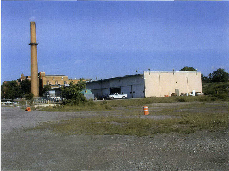
Photograph 35: View of Structure 14, presently a Siemens facility, facing northwest.
