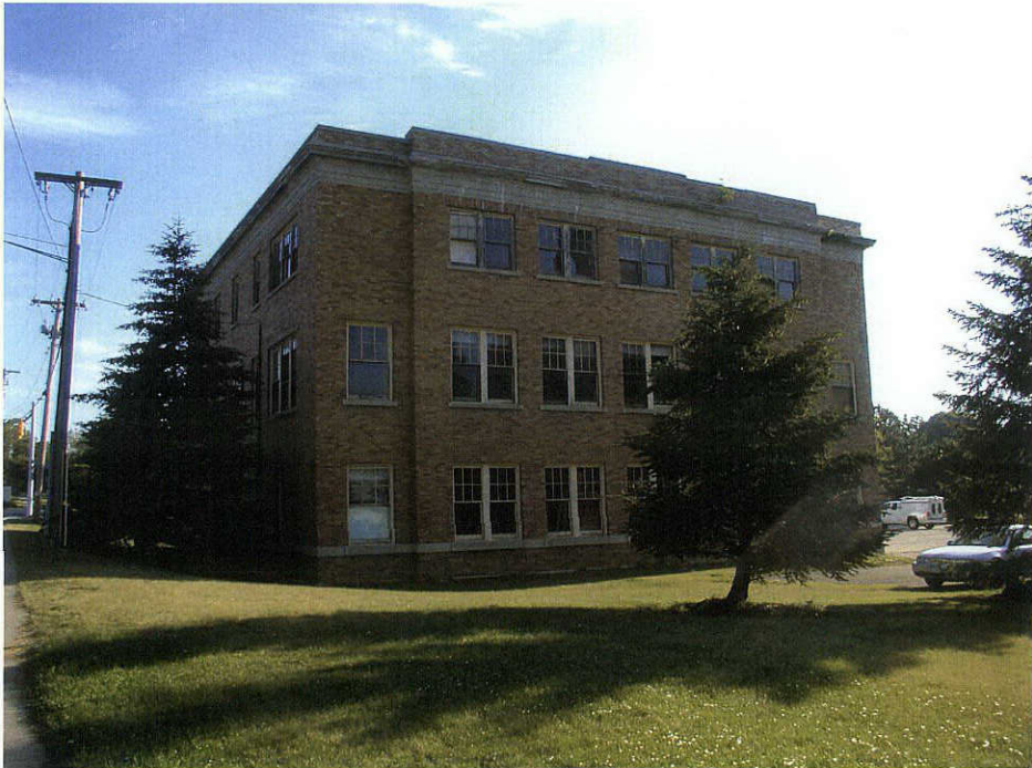
Photograph 24: View of Structure 9 (i.e., a service building), presently abandoned, facing northeast.
