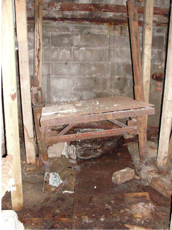
34. Basement abandoned sidewalk lift.
