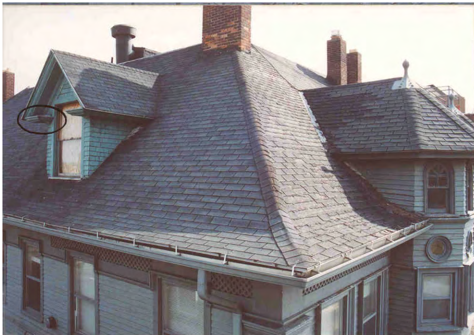
11. Main sloped roofing. 1
