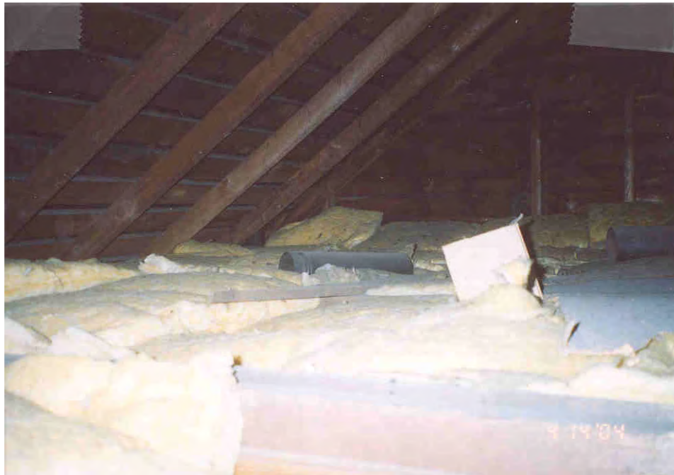
16. Attic of building rafters recommended
