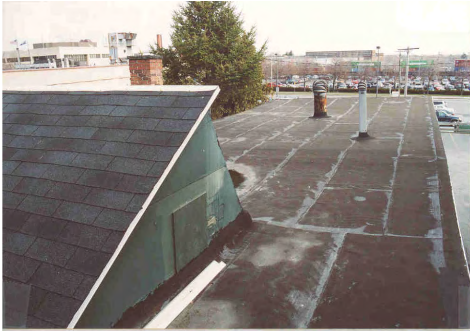
7. Building 2a roofing 1
