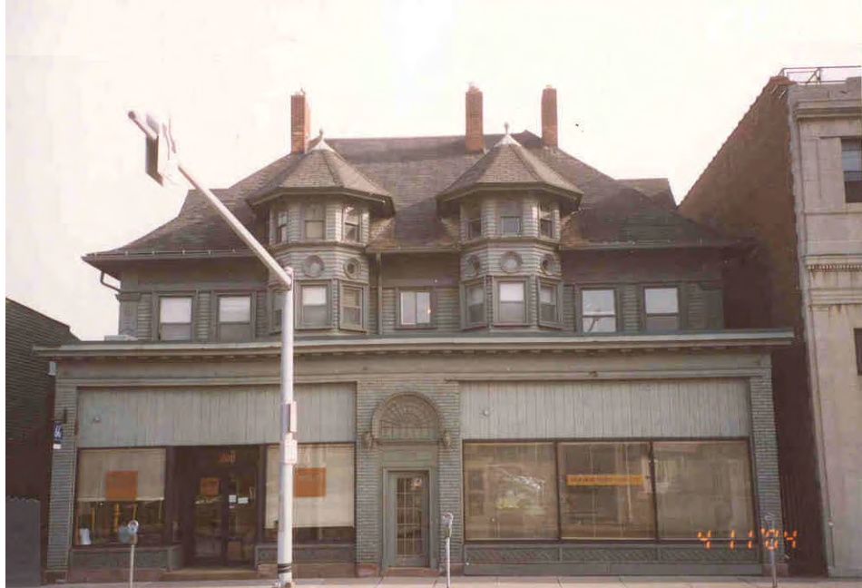
1. Building 3 looking north.
