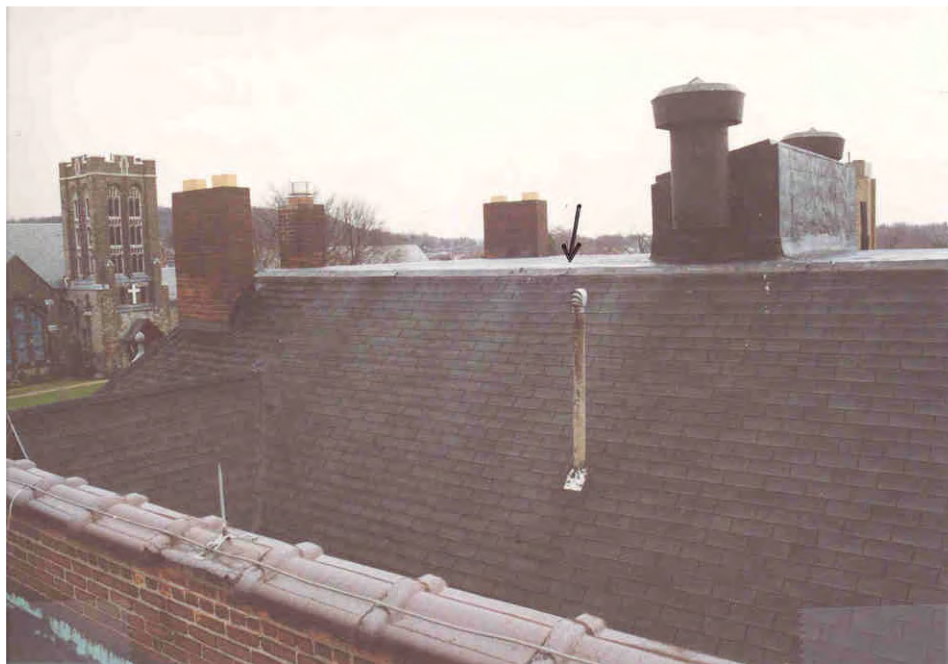
9. Upper flat roofing.
