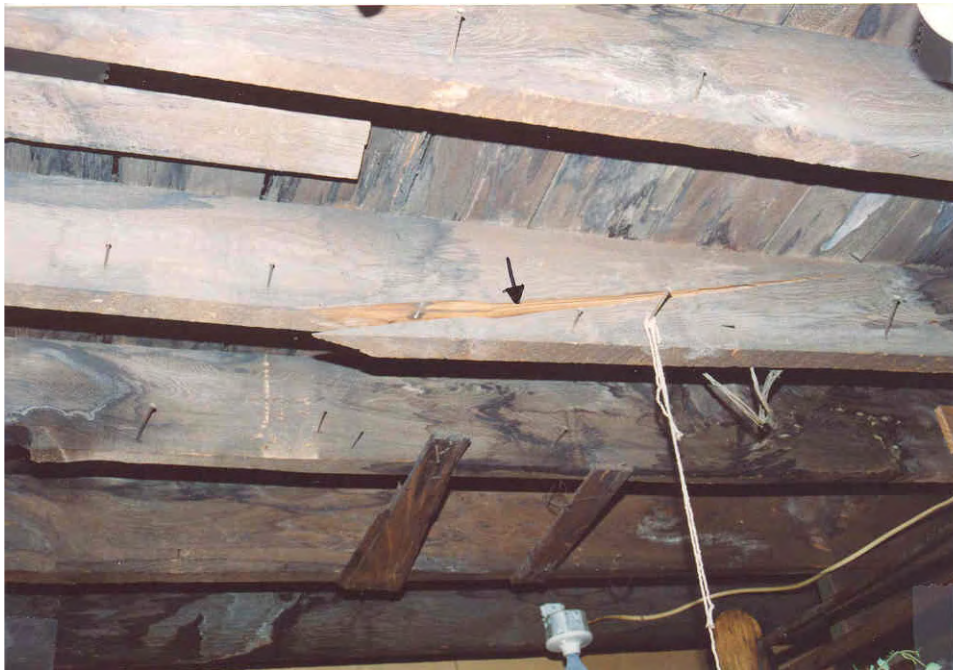
10. No insulation or finish at east side.
