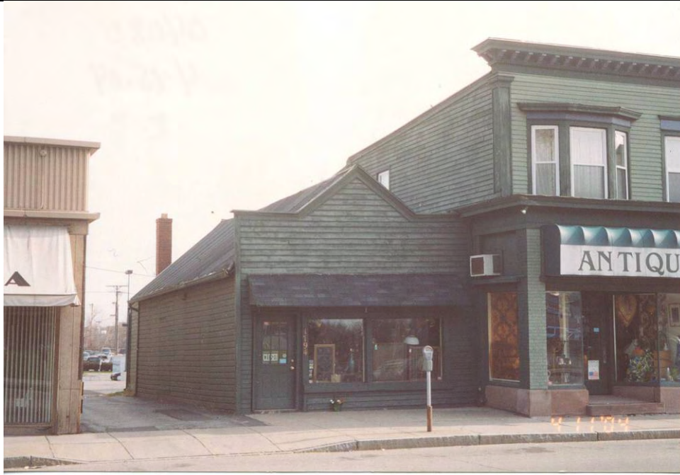
1. Building 1 looking north.
