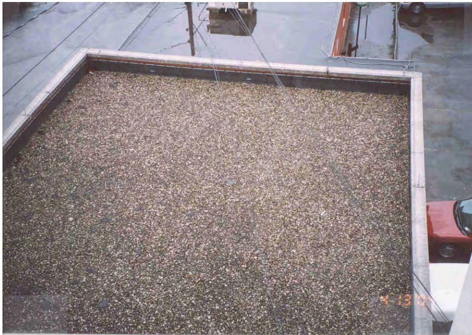
6. Roof 4a from above.
