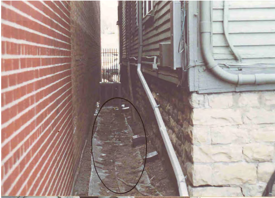
4. Wet alley between buildings 3 and 4.
