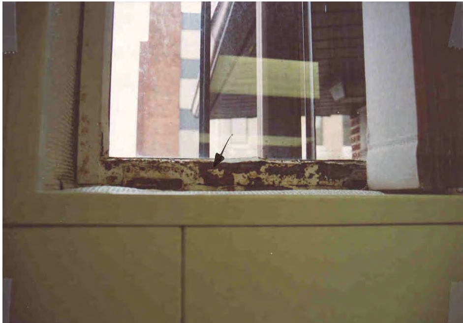
20. Typical condition of steel windows.
