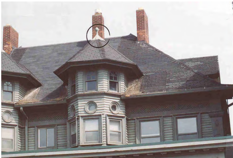
13. Main slope roofing, note cap.
