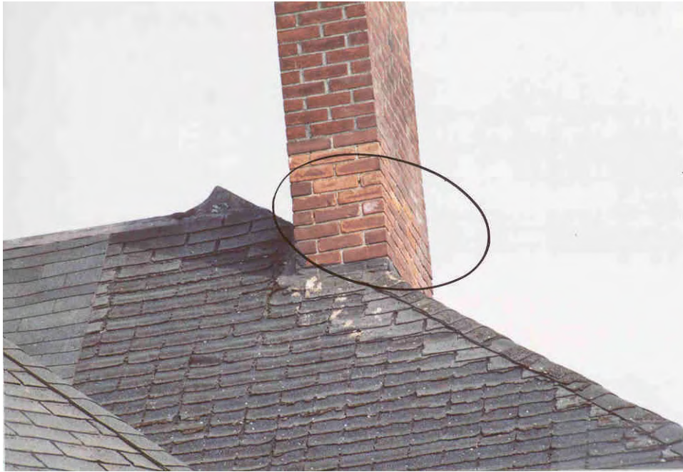
18. Typical chimney flashing.
