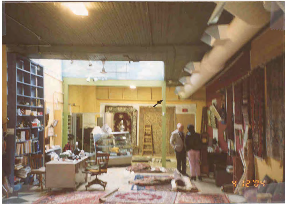
21. Post supporting skylight.
