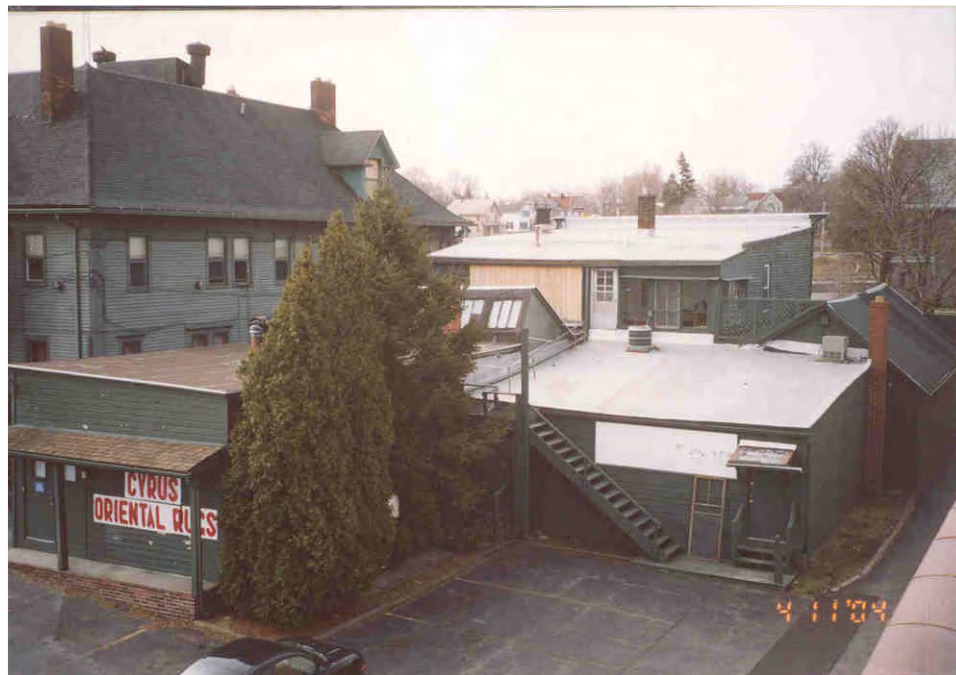
2. Buildings 1 & 1a looking south
