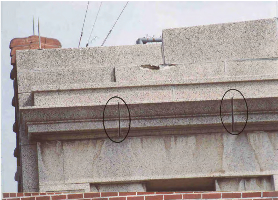
14. Close-up of south facade joints.
