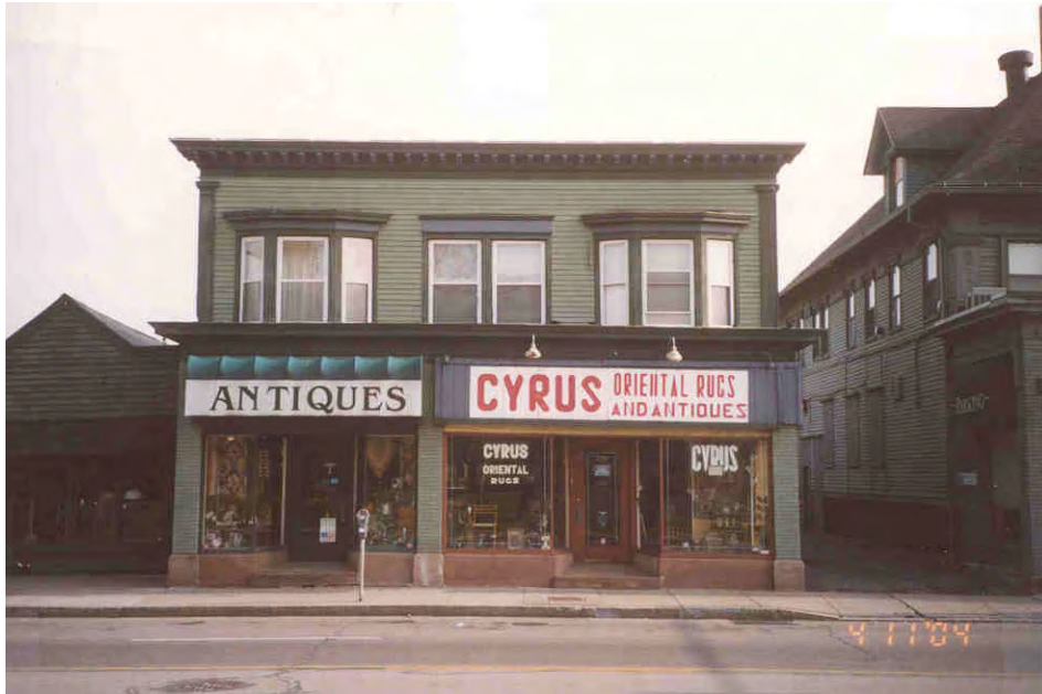
1. Building 2 looking north.
