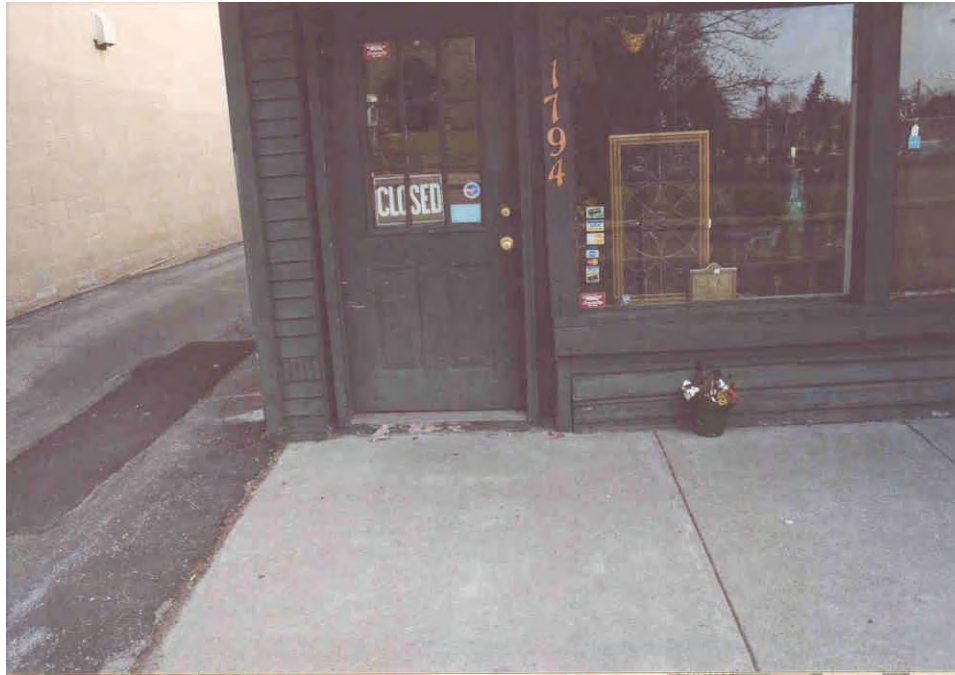
17. Cracked grille on door, note small step into building.
