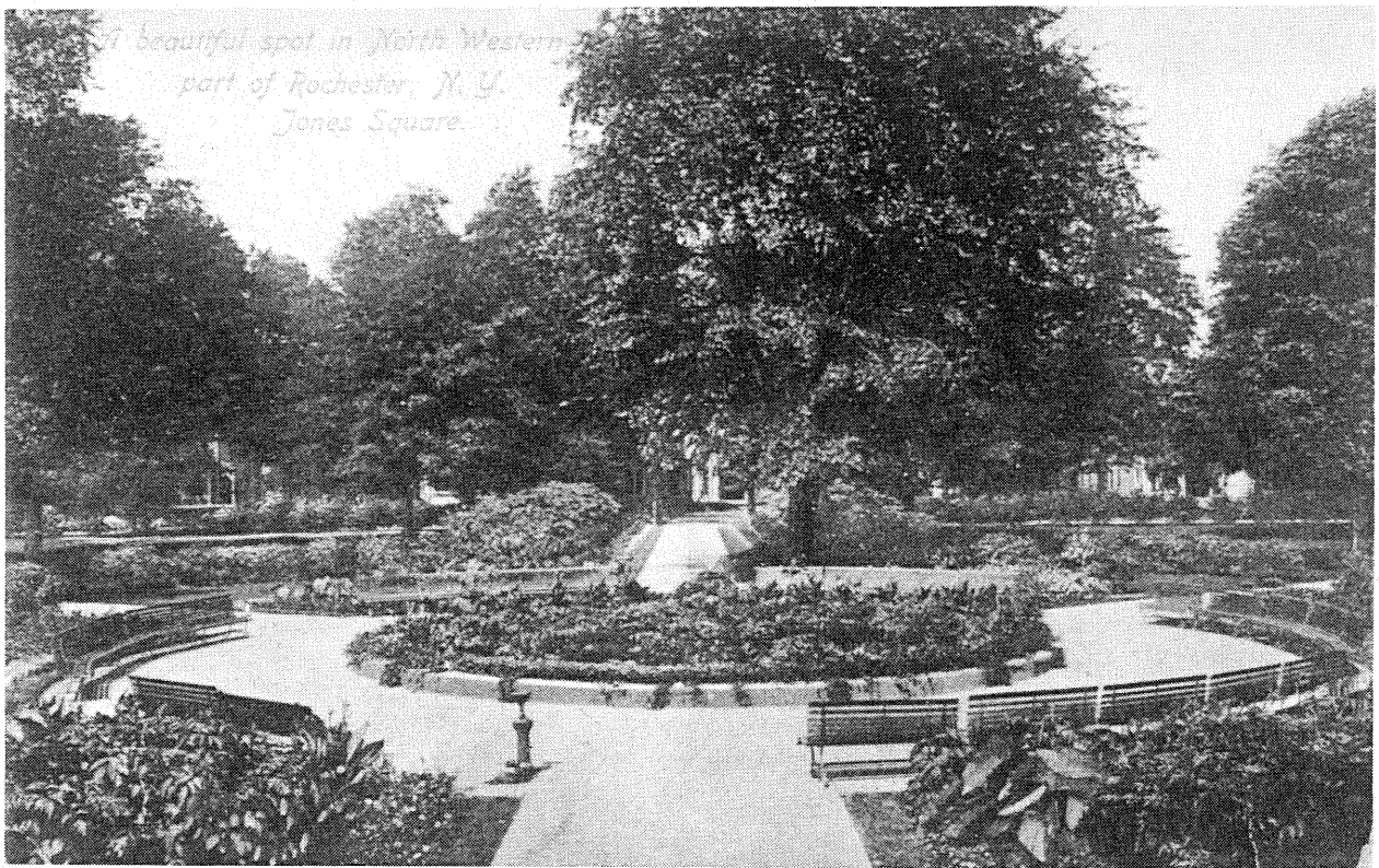
Figure II.10: Jones Park with central water feature in operation.
