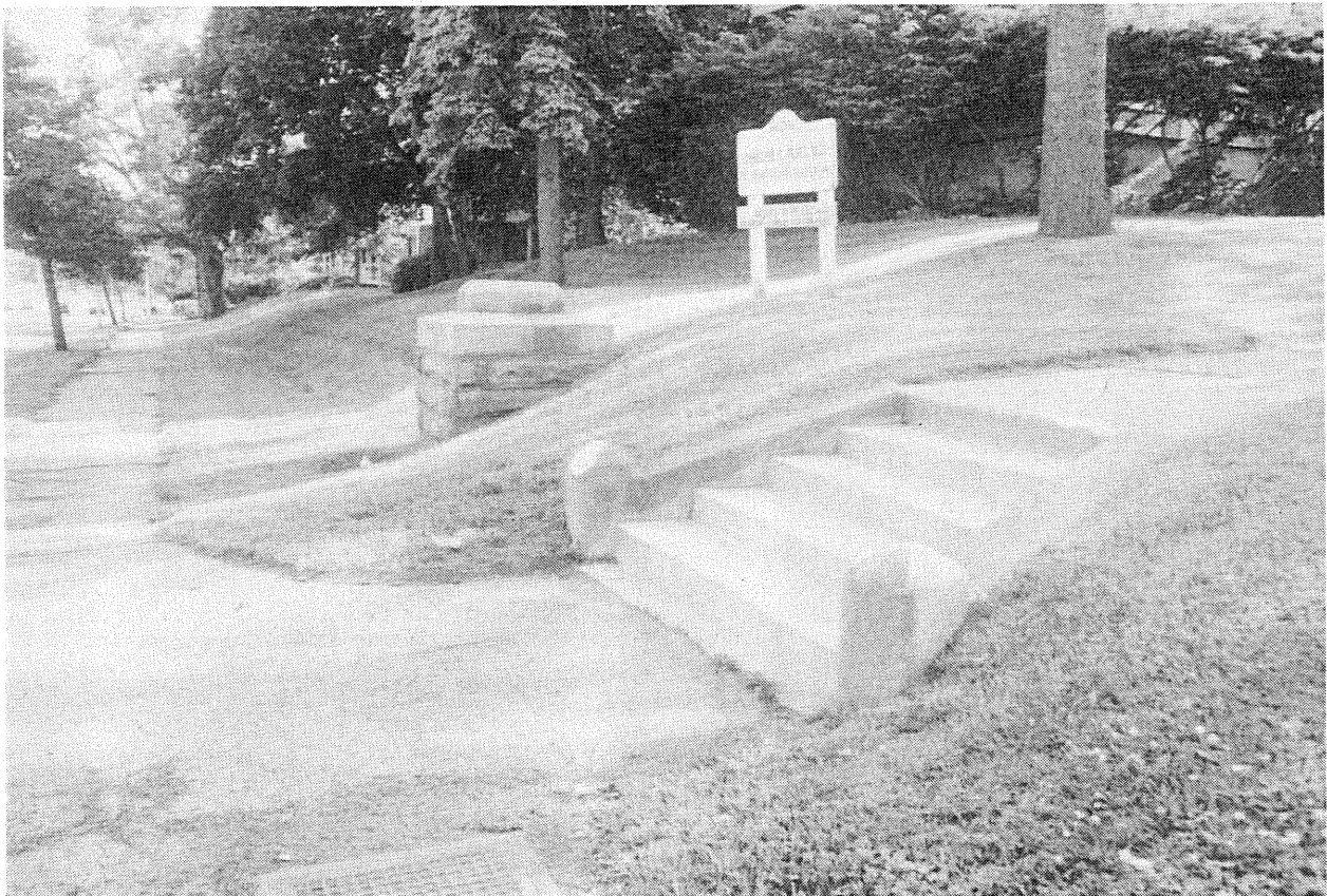
Figure II.23: Current view of the more southerly entrance from Lake Avenue to Lake View Park and the remnant light base. LANDSCAPES 1993.
