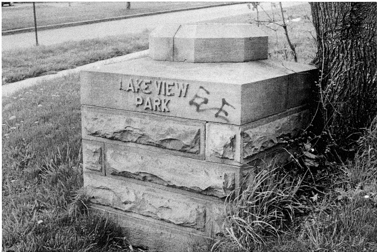
Figure III.2: Base of one of the historic Lakeview Park light standards. Notice the encroachment of earth and trees at the back and the missing light fixture. Courtesy of George Wheeler, 1993.
