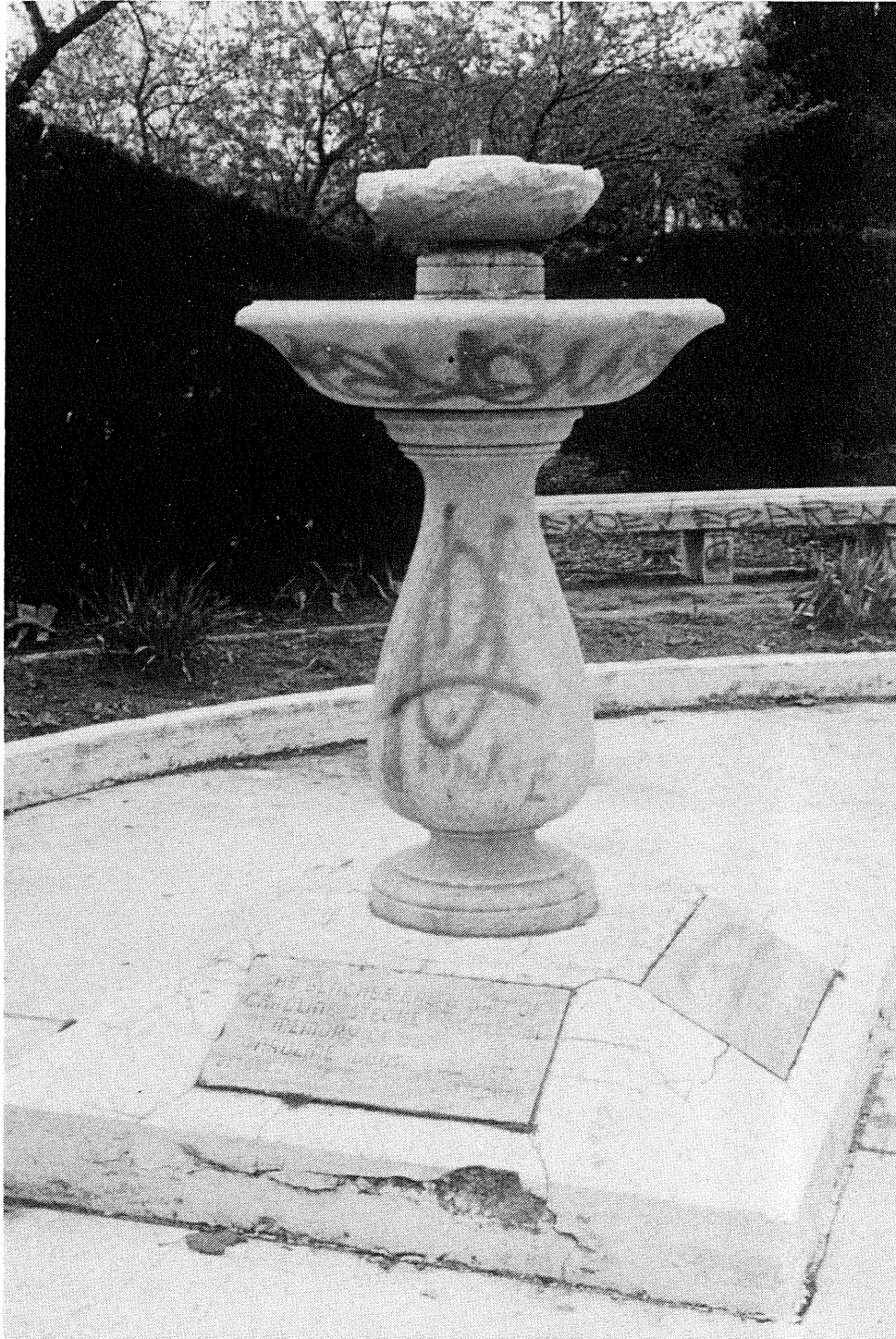
Figure III.4: Stecher Memorial Fountain in the Maplewood Rose Garden. The fountain is non-operational. Extensive cracks are noticeable on the fountain. Graffiti covers the marble fountain and the adjacent bench. Courtesy of George Wheeler, 1993.
