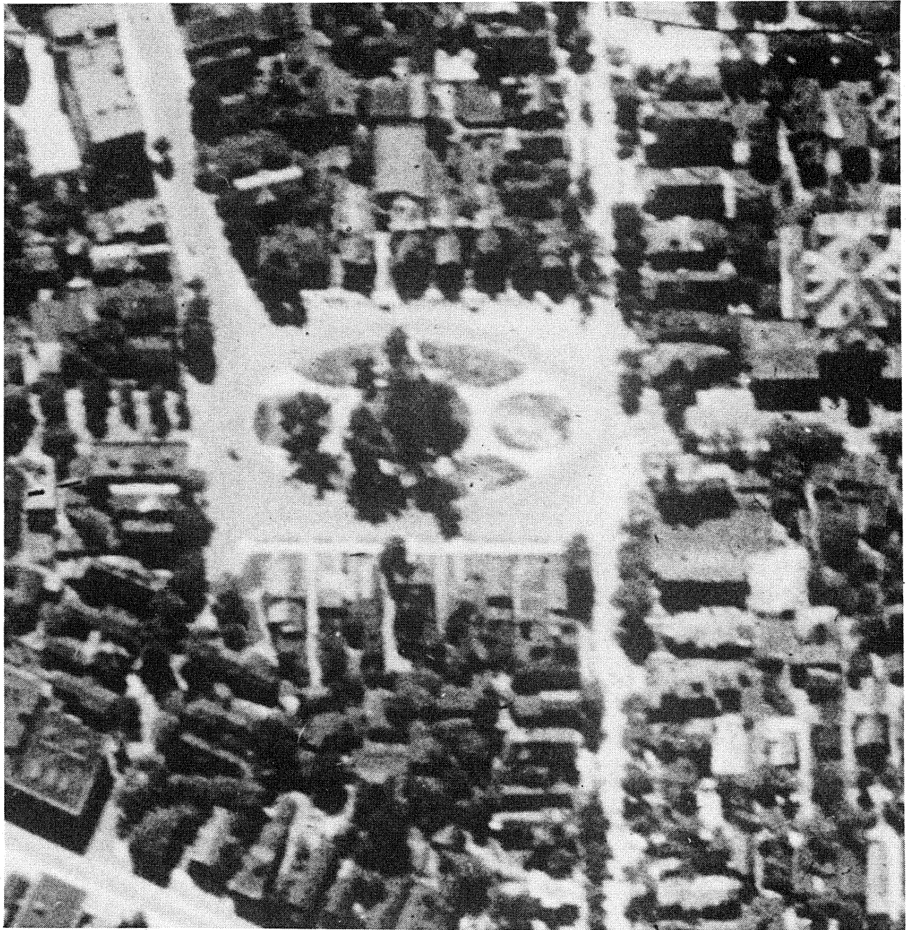
Figure II.37: Aerial photograph of Franklin Square, c.1926. Courtesy of City of Rochester, Department of Engineering Records.
