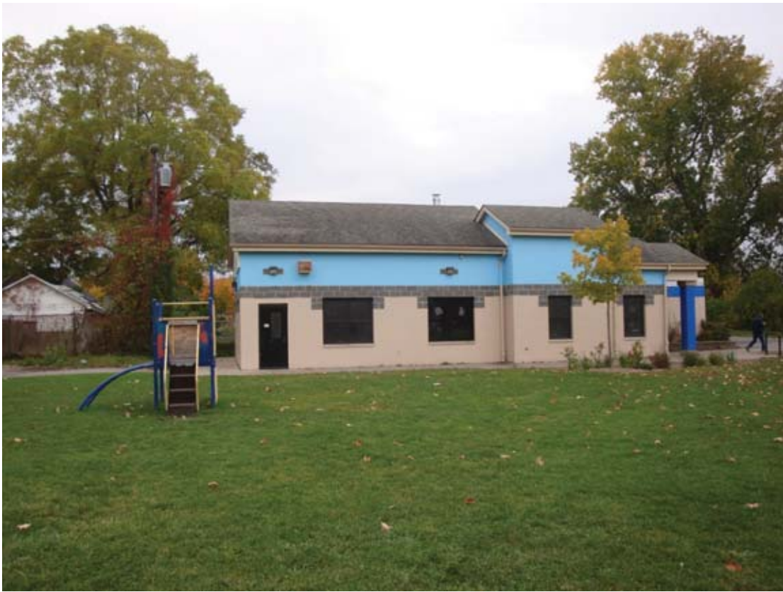
Campbell Street Recreation Center, looking south, 2009.
