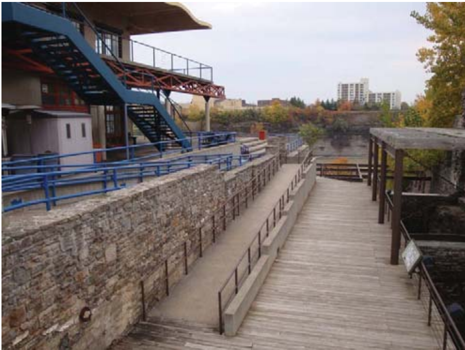
Triphammer Park, looking east, 2009.
