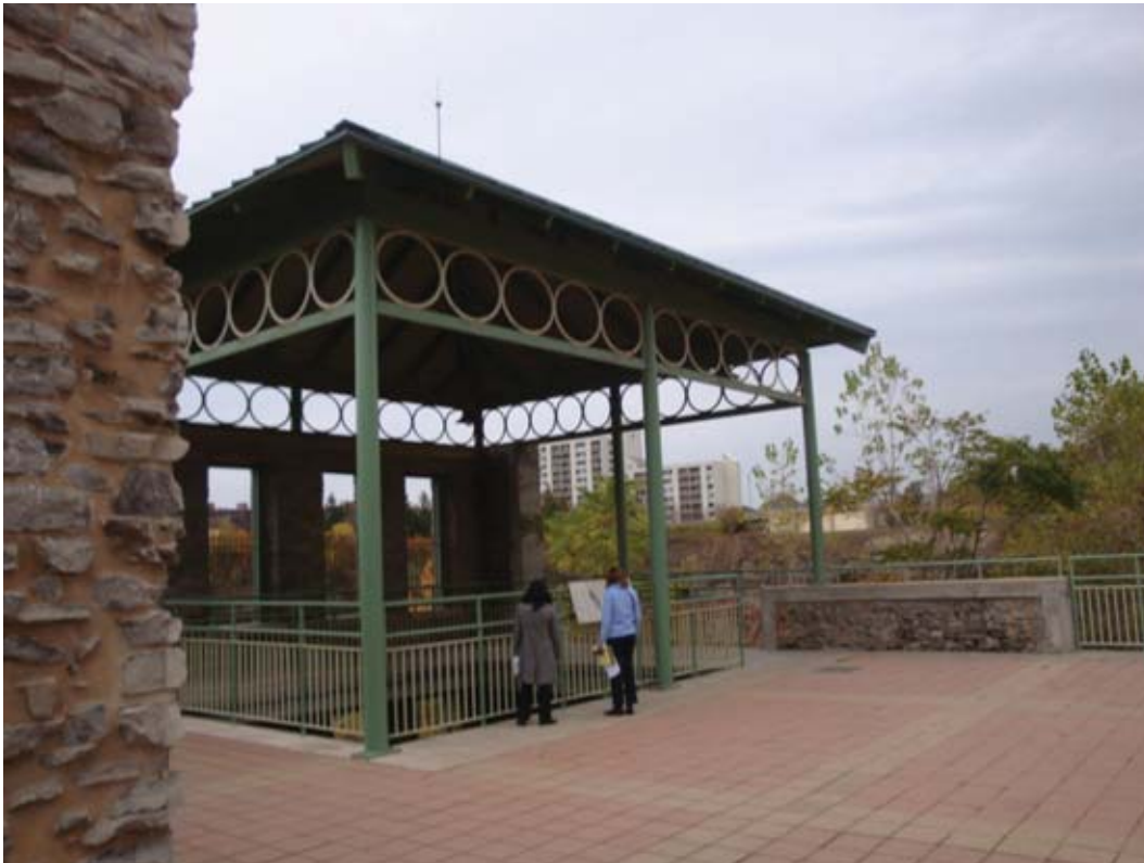
High Falls Festival Site, structural canopy over industrial remnants, 2009.
