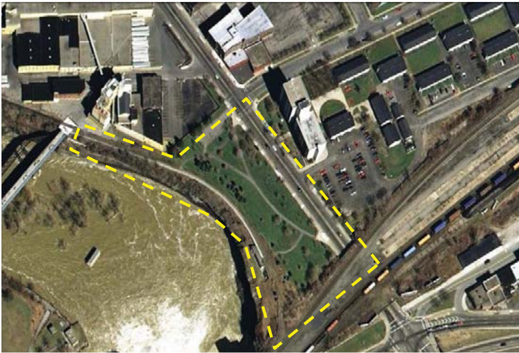
High Falls Terrace Park, aerial photo. (Google / NYS GIS Clearinghouse)
