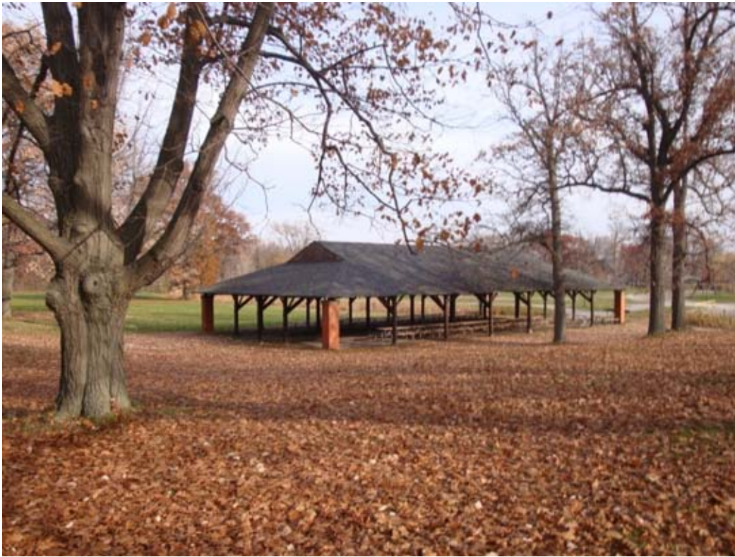
Genesee valley Park, CCC era pavilion structure, 2009.
