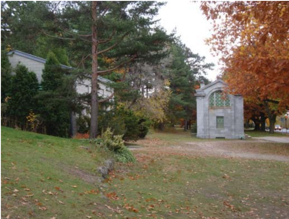
Cobbs Hill Park, pump house buildings near Monroe Avenue, 2009.
