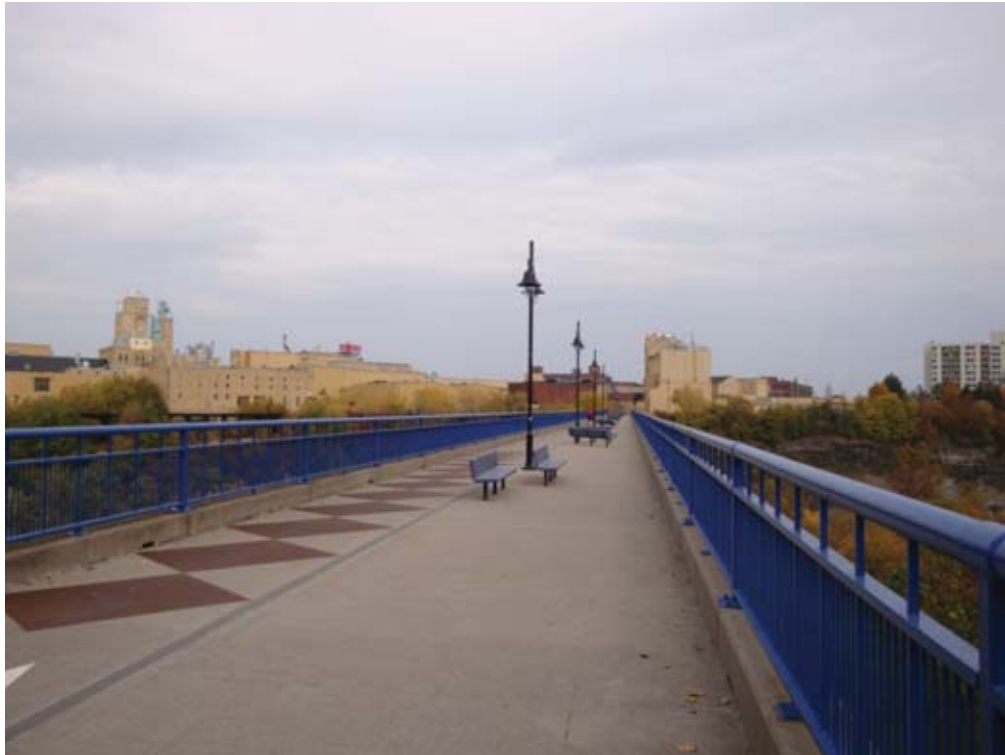
Pont de Rennes Bridge, looking east across bridge promenade, 2009.
