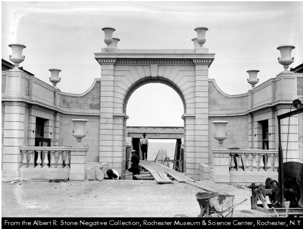
Durand-Eastman Bathhouse under construction, c. 1920
