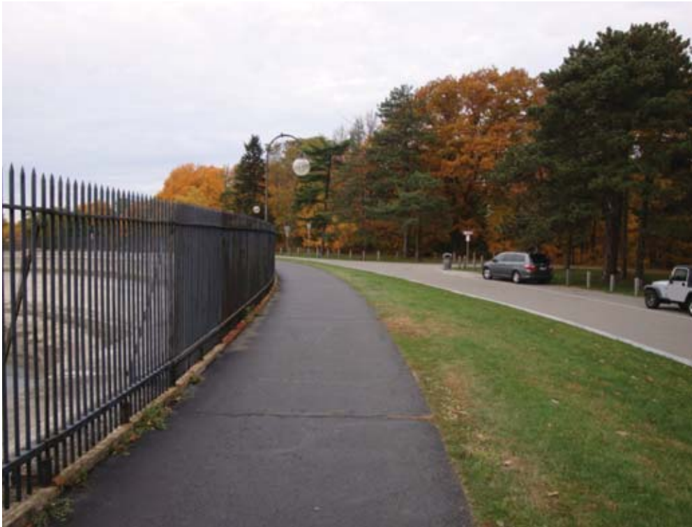
Cobbs Hill Park, reservoir fence and loop road, 2009.
