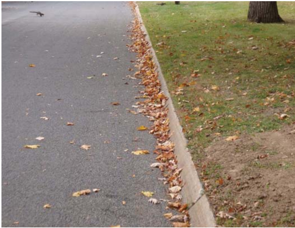
Knickerbocker Mall, angled curbing, 2009.
