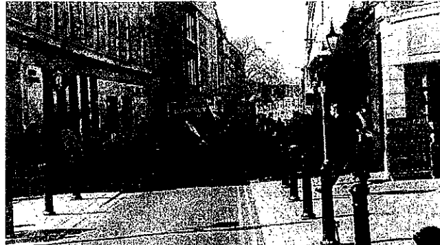
FLUSH CURBS AND STEEL BOLLARDS
