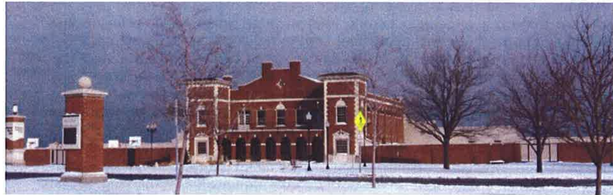
Former park bathhouse at the Ontario Beach Park, now a community center, is a reminder of the area's history. Photo: ZHA, Inc.
