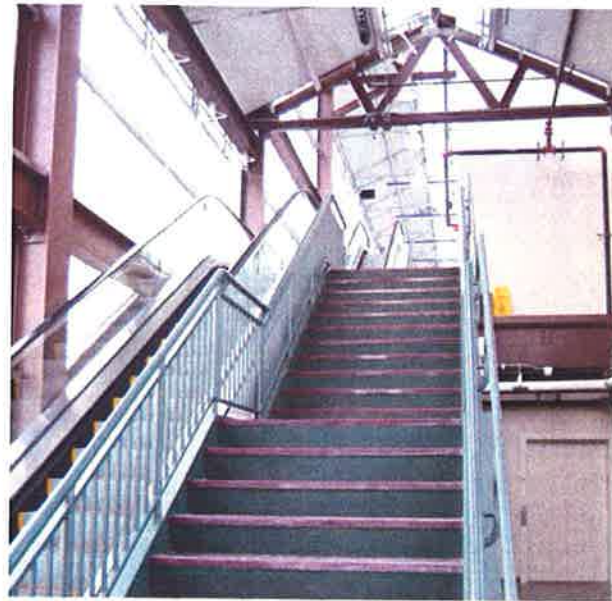
Figure 15. Interior of Link Building
