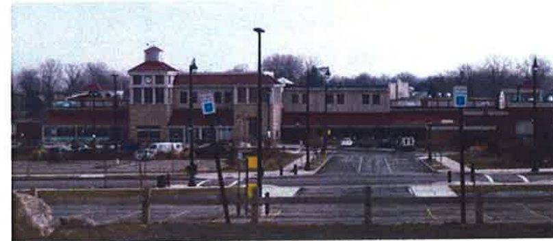
Figure 13. Ferry Terminal Building
