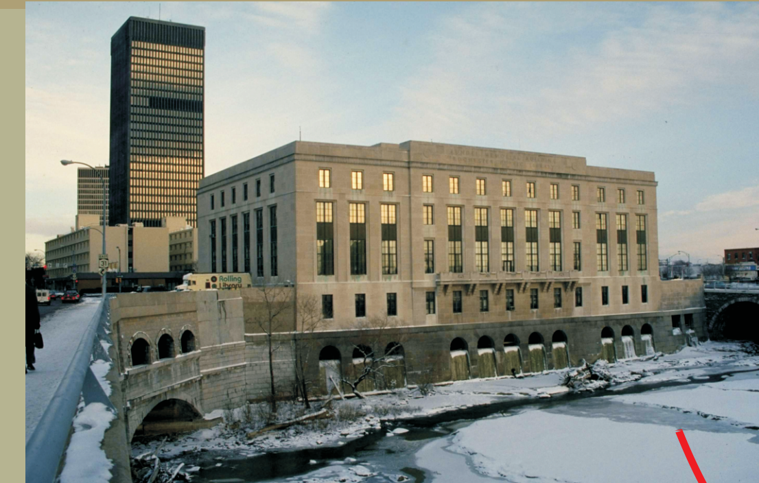
Above 1989 view of Rochester Public Library - Note the arched tail races below the building and the arches of the aqueduct to the left of the building. Site of library shown by dotted box on map. Rochester Images: From the Collection of the Rochester City Hall Photo Lab
