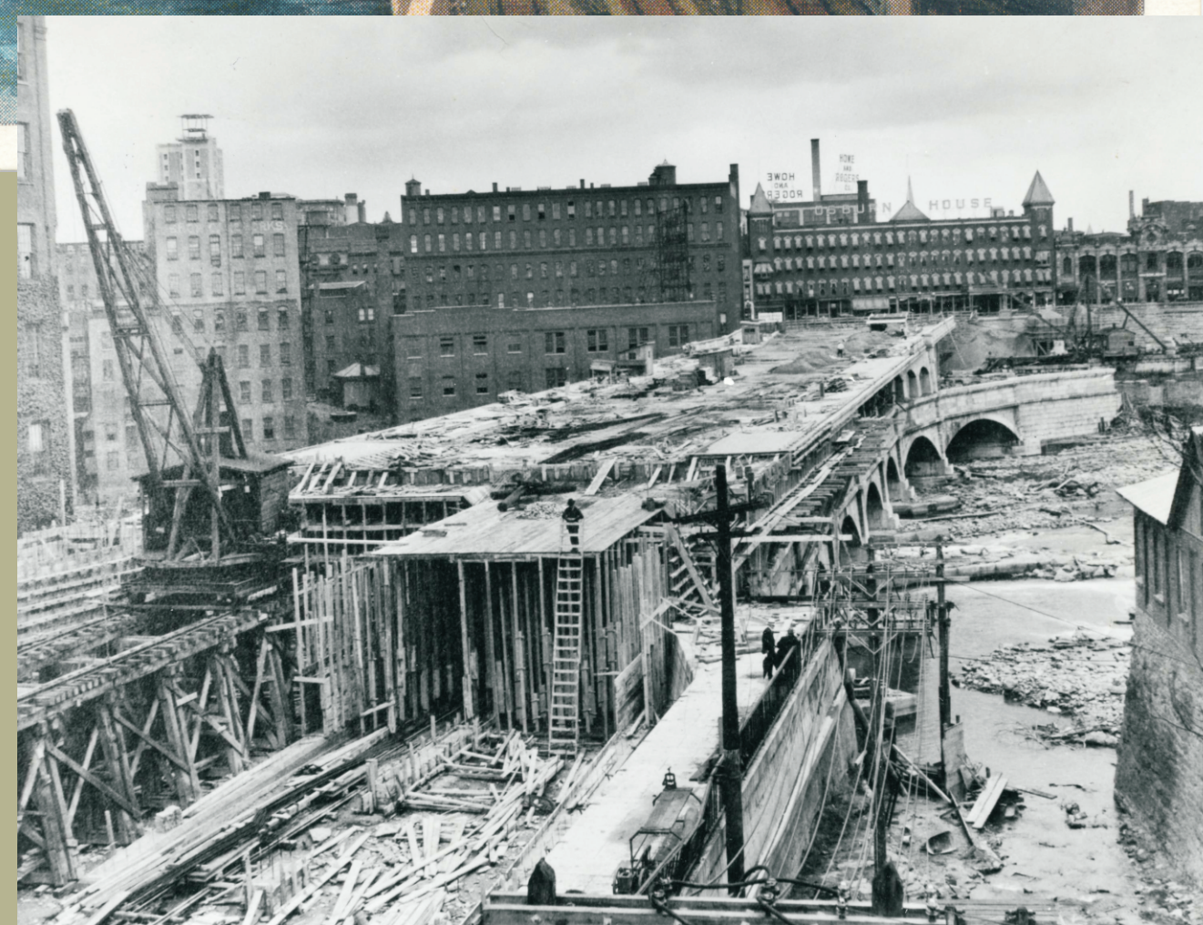
Above: 1923 Construction of second level over the old Erie Canal aqueduct. Note the Osburn House hotel in the background. From the Albert R. Stone Negative Collection, Rochester Museum & Science Center
