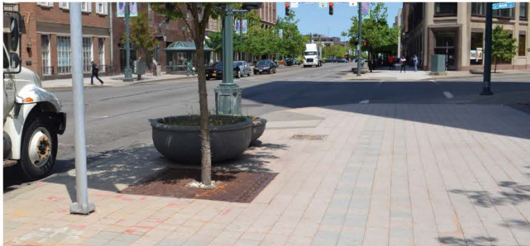
Existing Main Street tree grate, planters and paving
