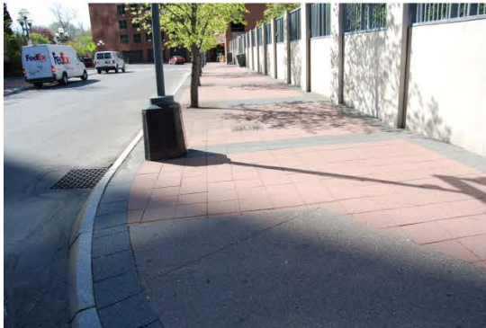
Existing Clinton Avenue and Broad Street paving
