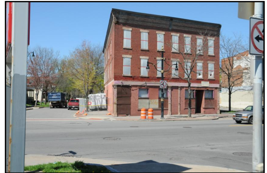
Figure 13 - The Wertz Building at 556-560 W. Main St. undergoing renovations as a part of Voter's Block Development
