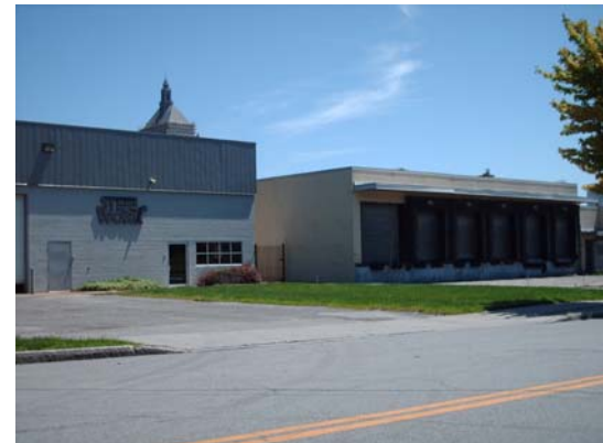
View looking east along Oak Street south of Jay Street
