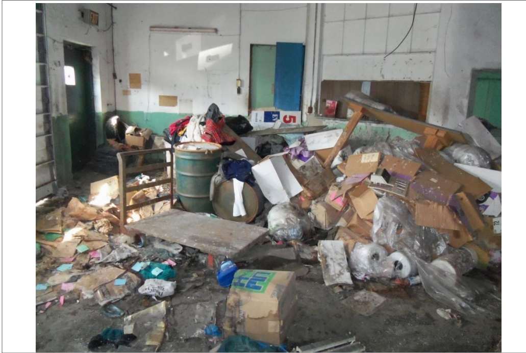
Garbage and drums in the main room of the vacant former United Cleaners building.
