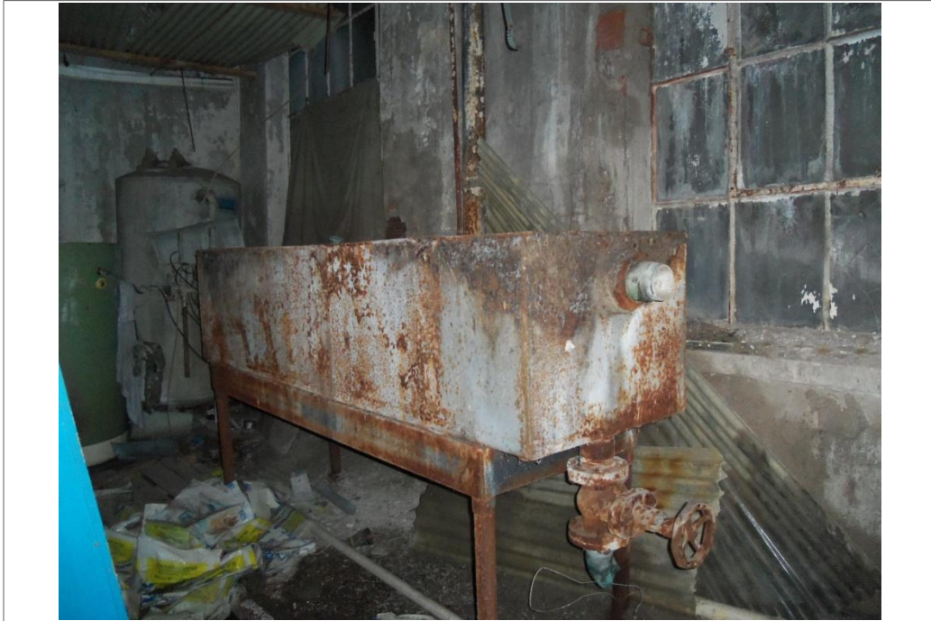
Container the main room of the vacant former United Cleaners building.
