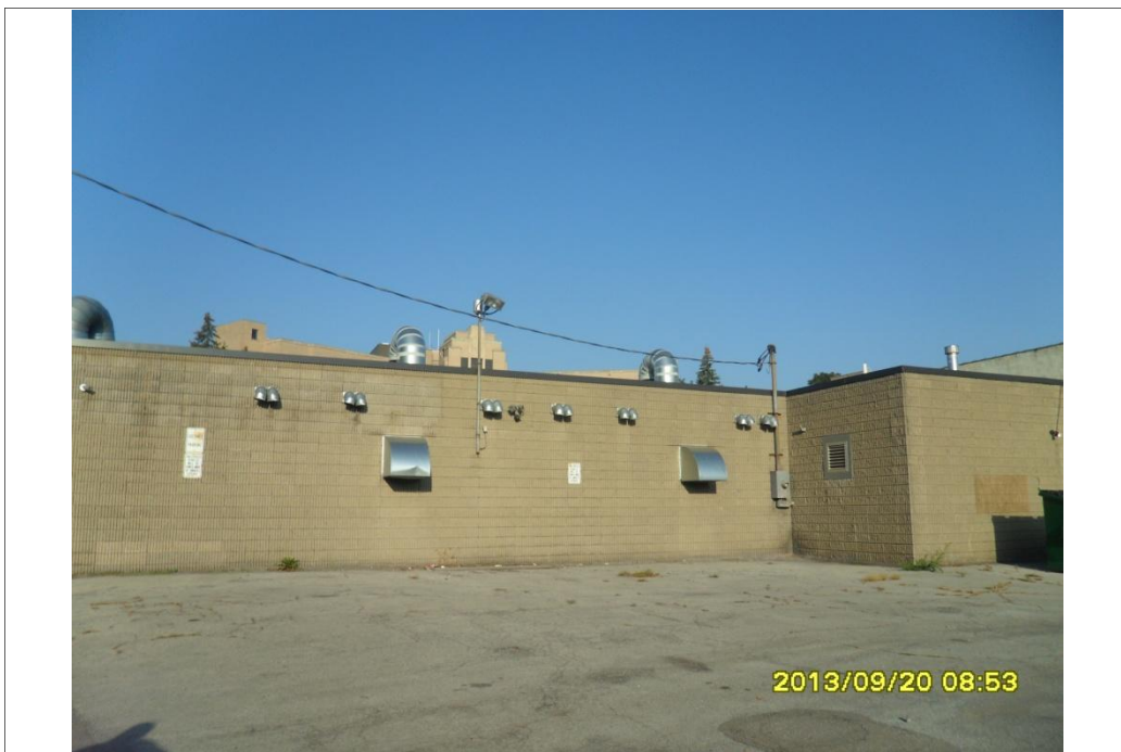
Rear of the Canopy Laundromat building..
