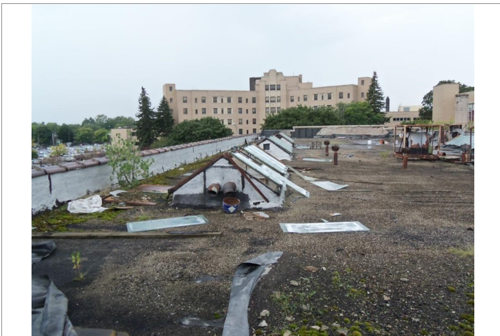
Roof of the vacant former United Cleaners building.
