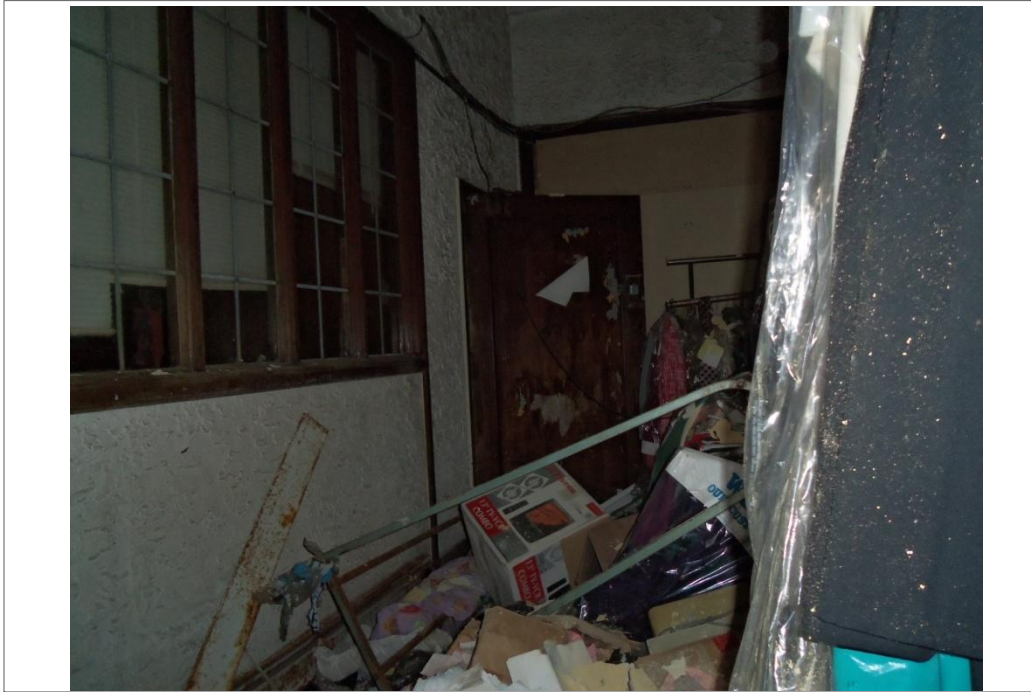
Storage room in the vacant former United Cleaners building.
