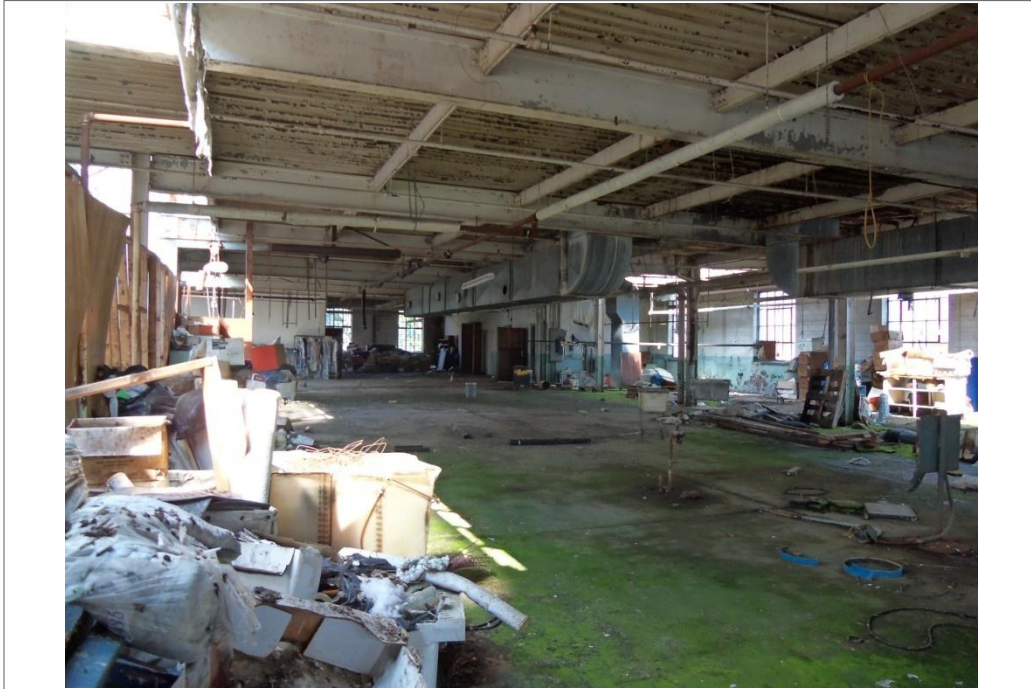
Second floor of the vacant former United Cleaners building.
