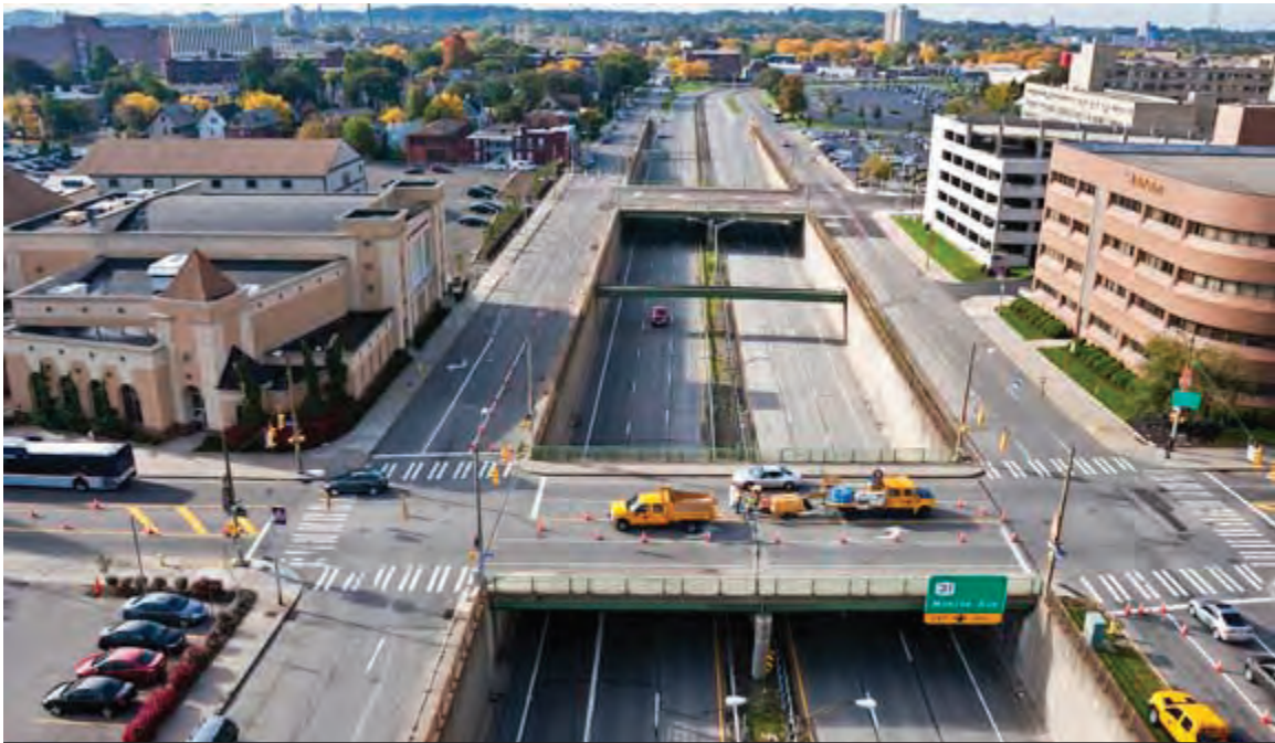
VIEW SOUTH LOOKING AT EAST AVENUE AND BROAD STREET BRIDGES
