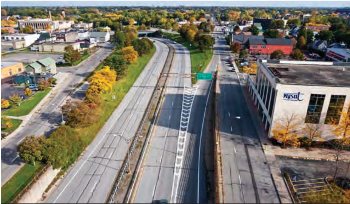
VIEW NORTH LOOKING AT N. UNION STREET OFF-RAMP
