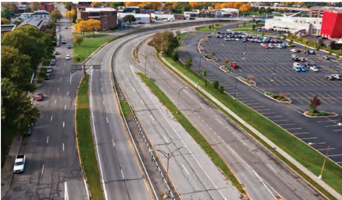
VIEW SOUTH LOOKING AT S. UNION STREET OFF-RAMP AND NATIONAL MUSEUM OF PLAY
