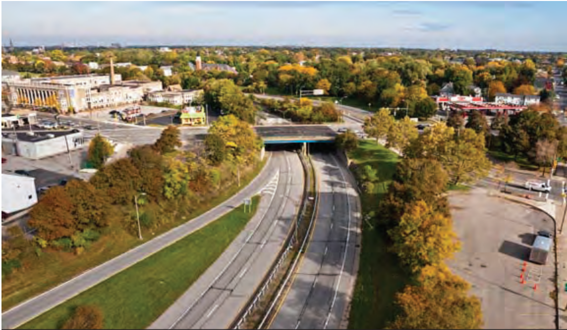
VIEW NORTH LOOKING AT EAST MAIN STREET
