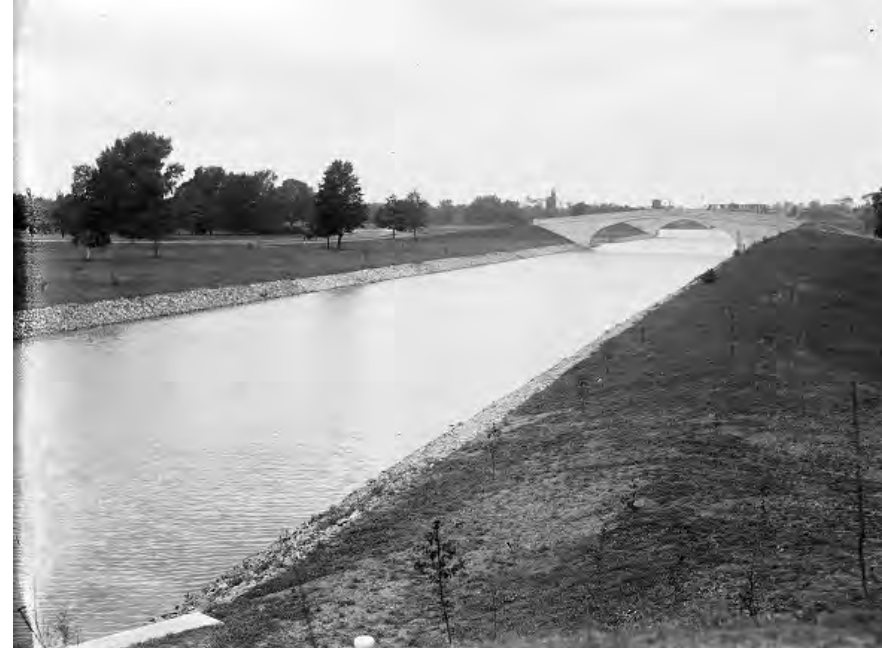
1921 Work is complete on efforts to remediate the damage done to the park landscape by the Barge Canal. View of Olmsted Brothers-designed pedestrian bridges across the canal.
