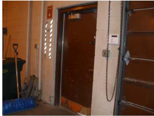
Interior side of exterior doors
