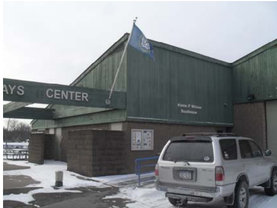
Main Entry approach from Parking lot
