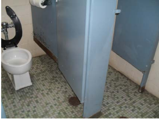
Interior Toilet Room
