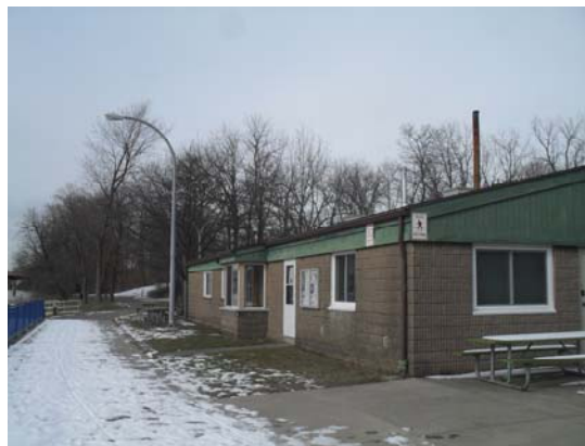
Exterior side along the Genesee River
