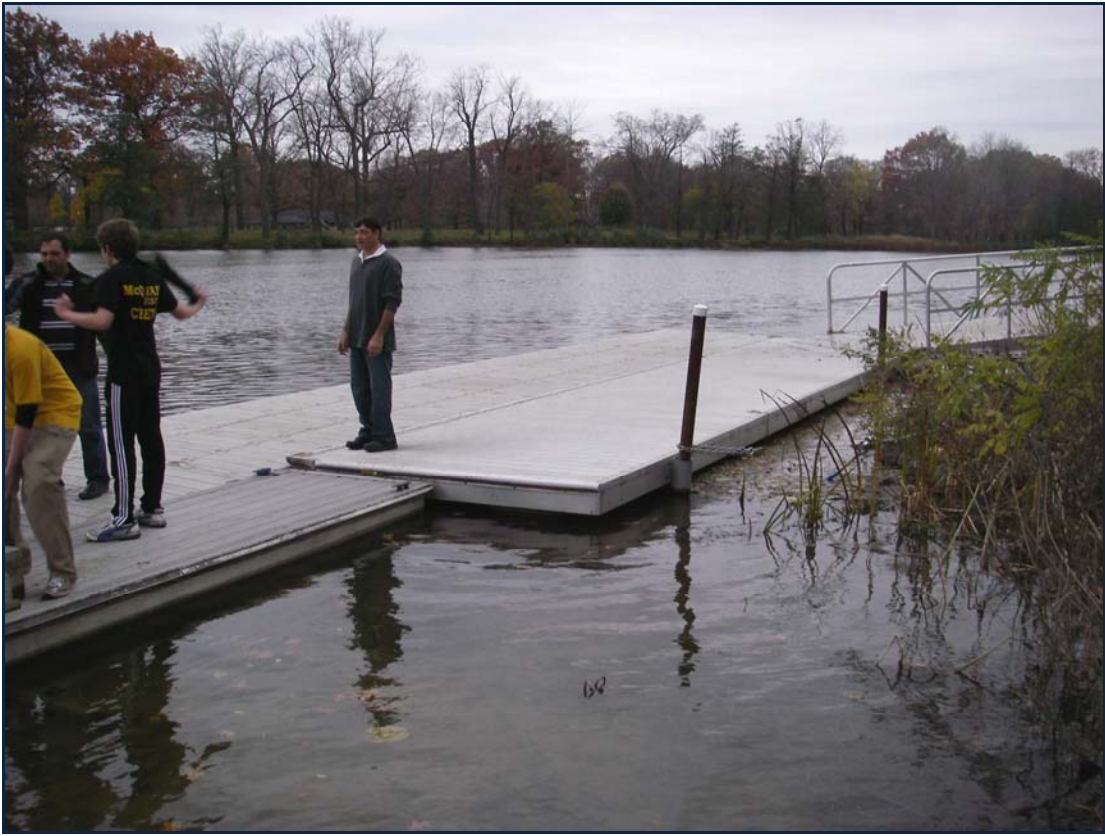
Figure 11 Privately Owned Dock
