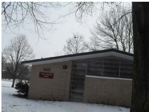
Front view of grade at building
