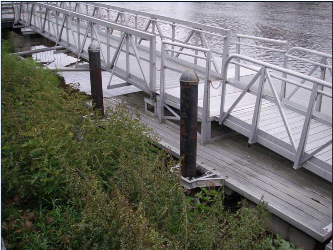
Figure 8 Steel Pipe Piles with Roller Guides
