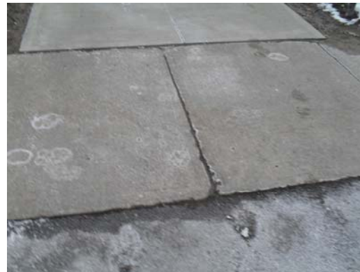
Sidewalk/Ramp transition - Accessible
